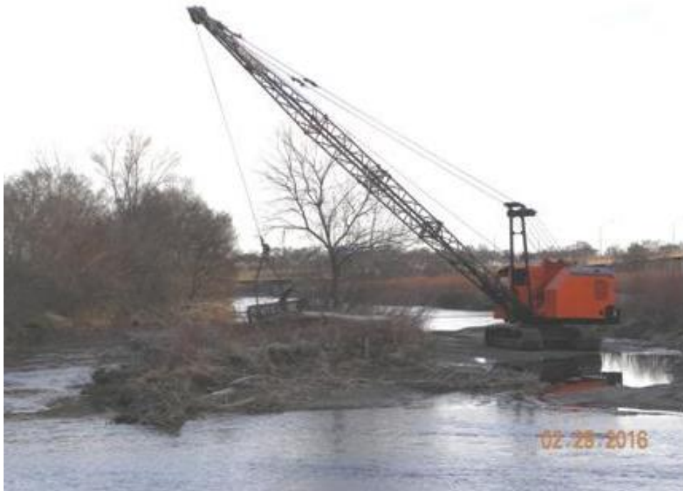
Dragline Removing Island A
