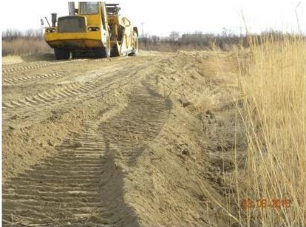
Pedal Scrapper Picking Up the 2014 “New” Dike
