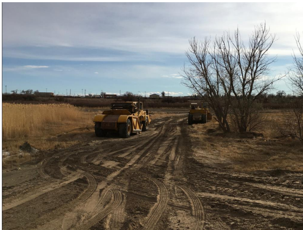
Pedal Scrapper Moving Material to the 1980’s Dike
