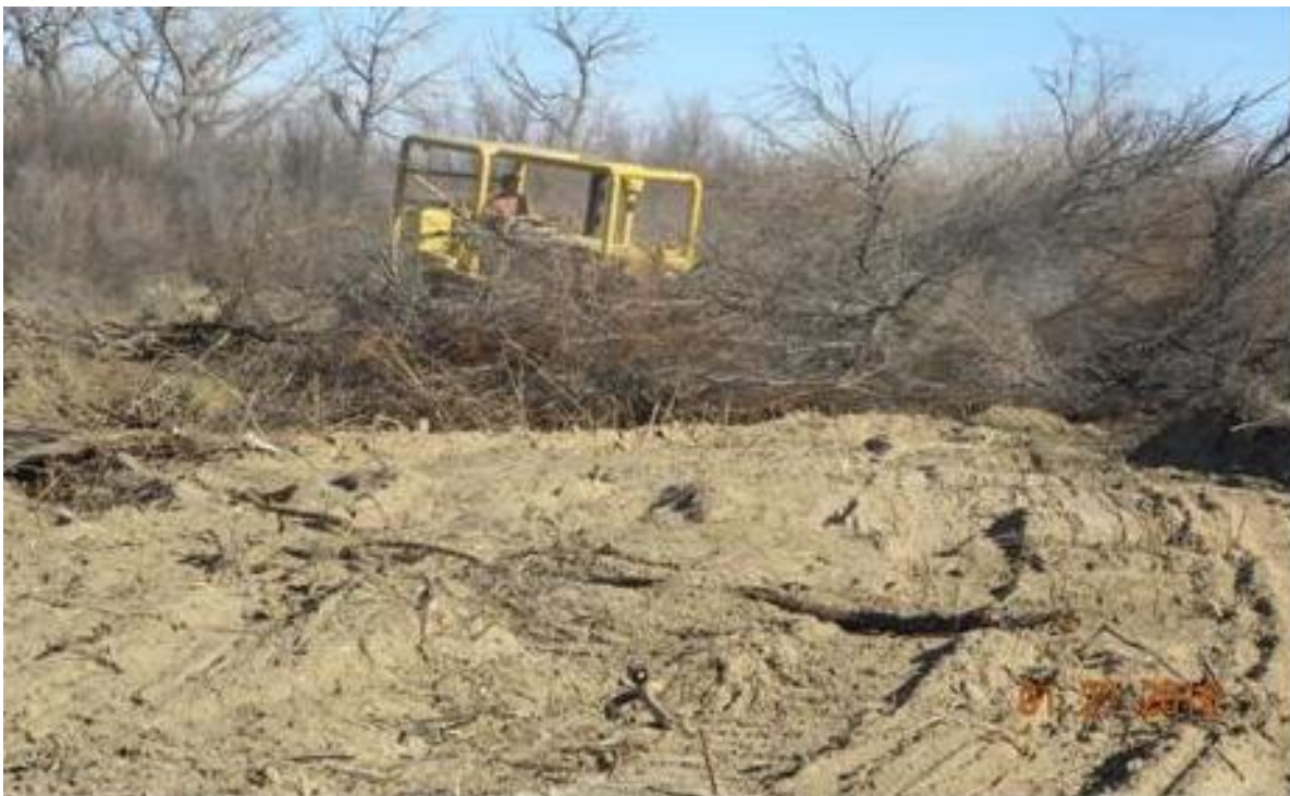
Bulldozer Moving Sediment from Island B
