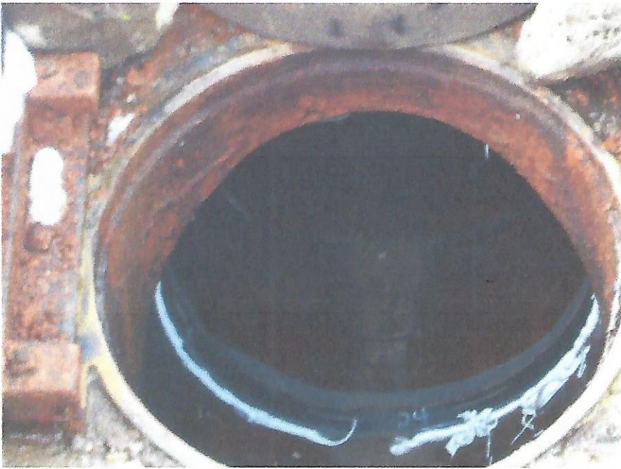
Hydrophilic seal in position at the upstream end of the existing outlet pipe.
