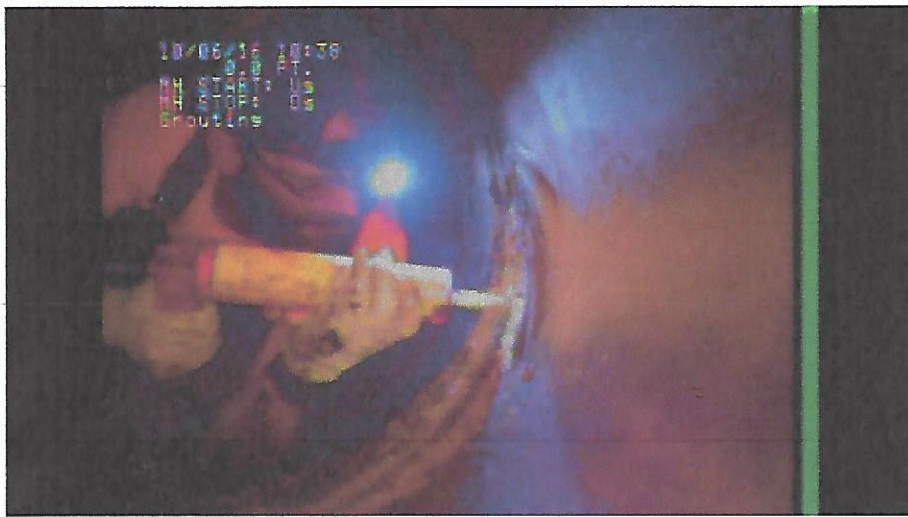
Contractor sealing and cleaning joint at location of observed infiltration. No infiltration was present at this time.
