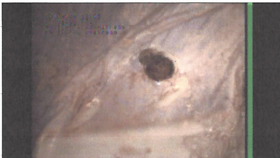
View of open airvent near crown of pipe.
