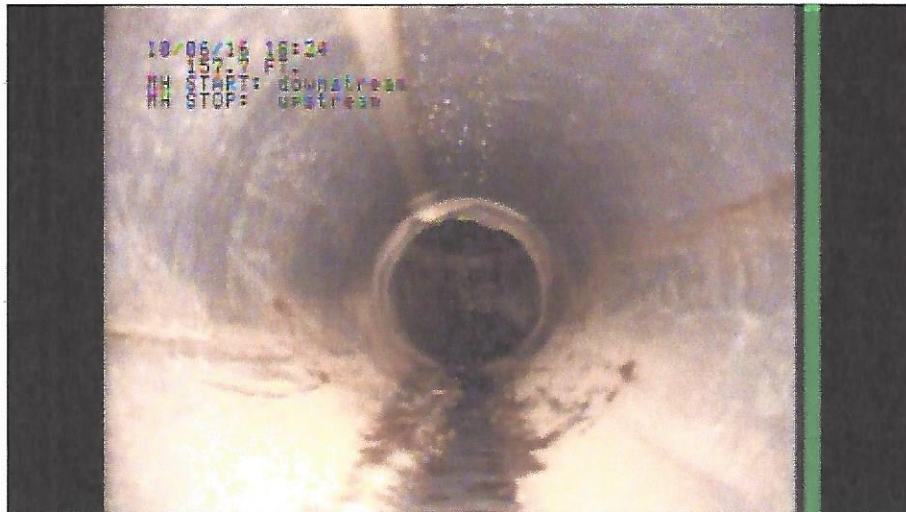
Interior view of upstream liner terminus shows small wrinkles in crown of pipe
