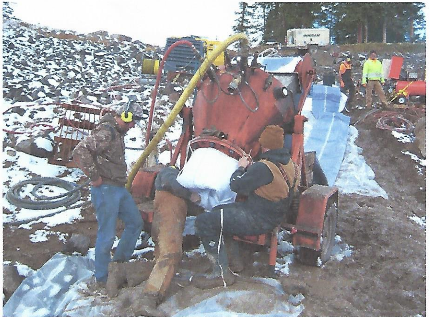
Liner being deployed from a pallette through the shooter and being inverted.
