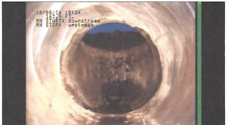
Interior view of the liner terminus and the elbow at the upstream end.
