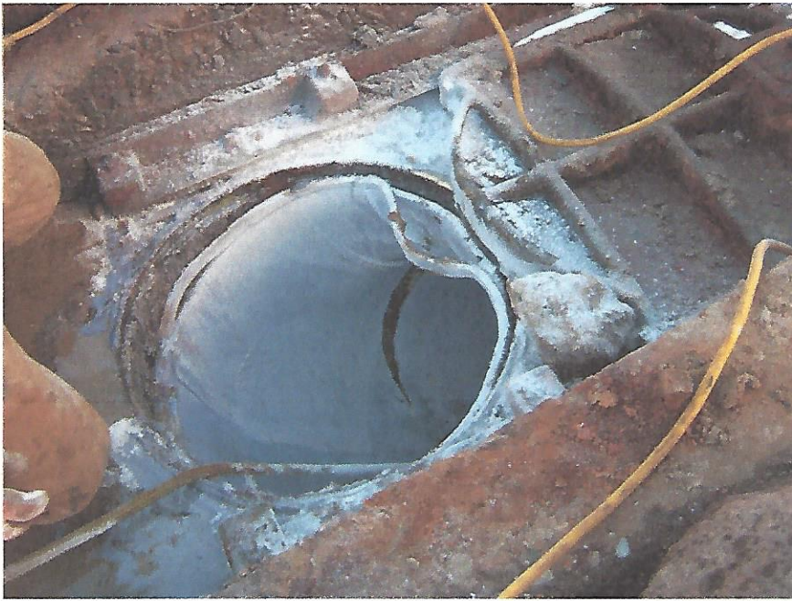
Fracture of liner occurred around the circumference at the transition with the elbow in front of the hydrophilic seal.
