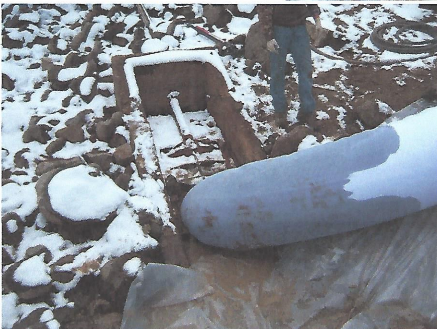
Liner inserted and inverted from upstream end using compressed air.
