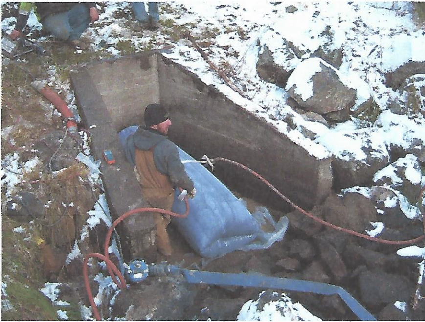
Downstream end of liner. Hoses are provided for steam venting allowing transmission through the entire length of the liner.
