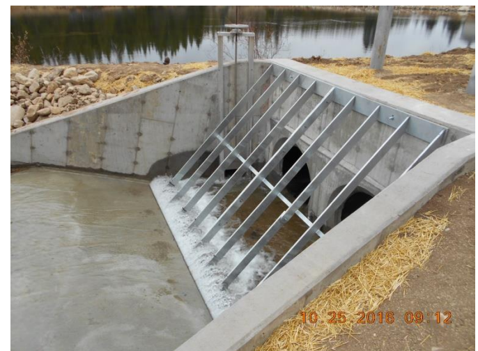
Trashrack at Inlet With Water Flow
