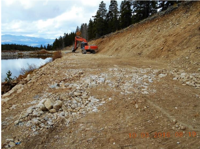
Fill Being Placed Over Pipes
