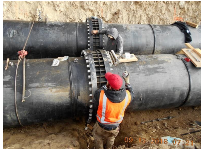
Final Bolting Of Flanges
