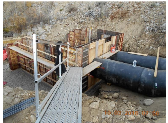
Forms Around Outlet Structure
