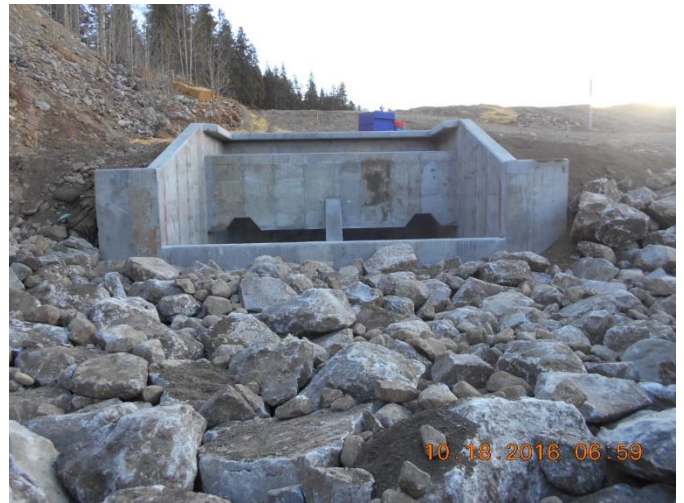
End View of Outlet Structure
