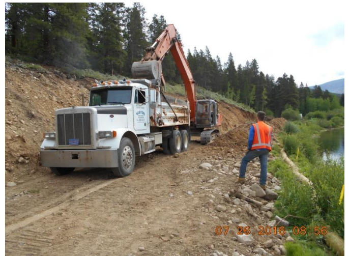
Trench Material Being Removed
