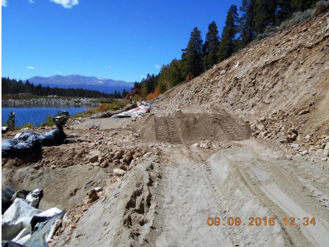
Initial Backfill Over Pipeline
