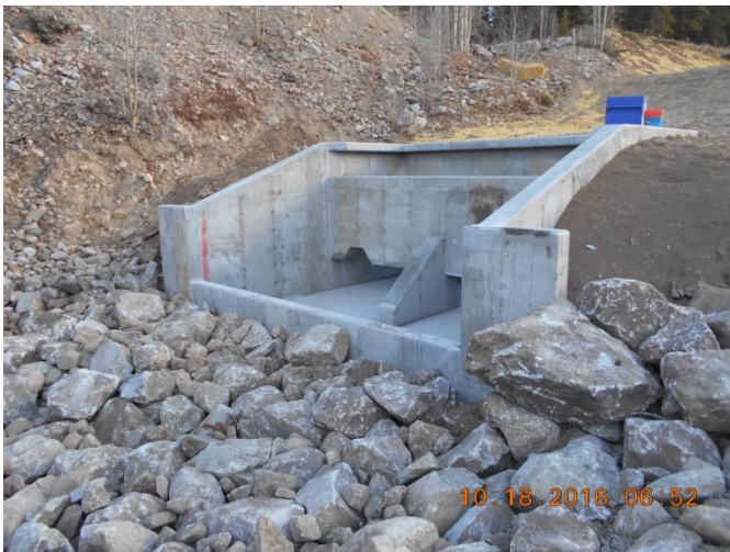
Completed Outlet Structure
