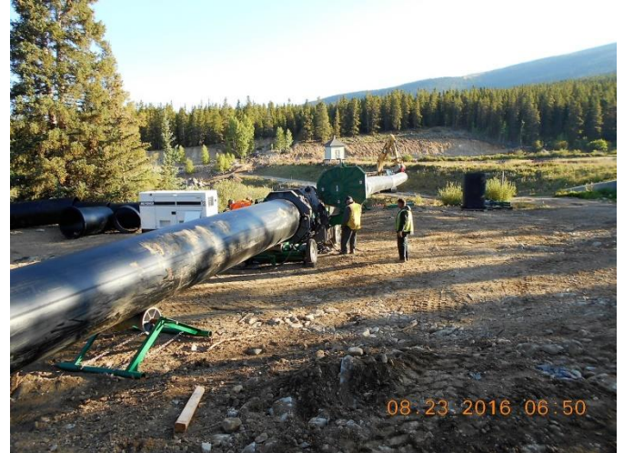
48" HDPE Pipe Being Fused
