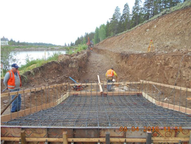
Inlet Structure Under Construction
