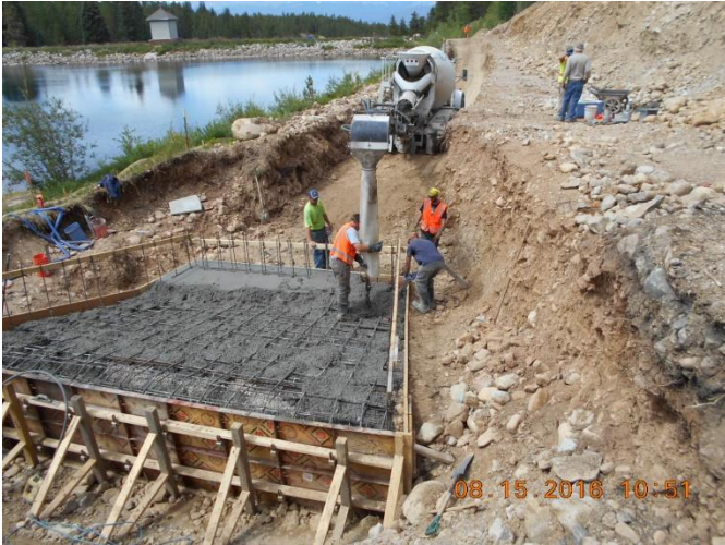
Concrete Being Placed at Inlet
