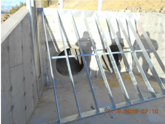
Trashrack at Inlet Structure
