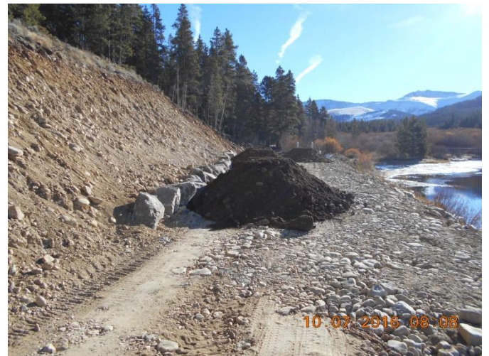
Top Soil Staged for Placement at Trench
