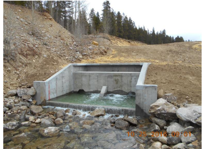
Water Flowing Out of Outlet Structure
