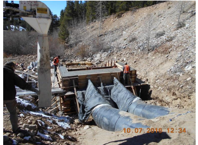
Final Finishing of Concrete at Outlet
