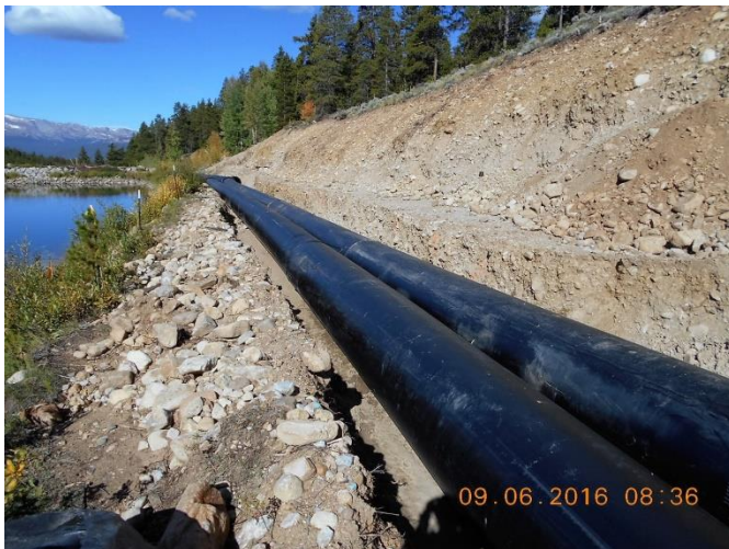
48" HDPE Pipes Placed in Trench
