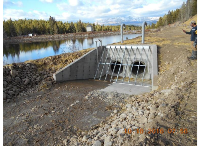
Completed Inlet Structure
