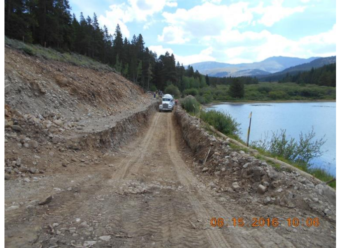
Concrete Truck Placing Concrete at Inlet
