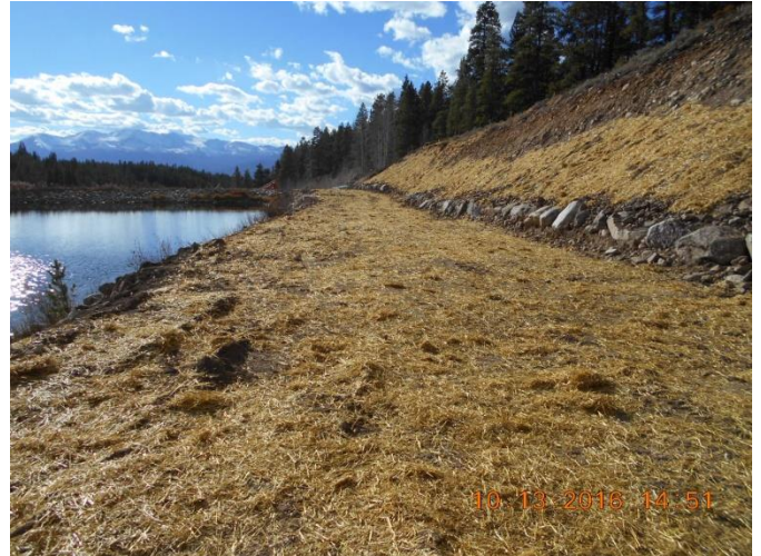
Straw Placed At Work Area for Reclamation
