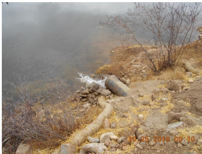
Water Being Diverted From Stream Into Reservoir
