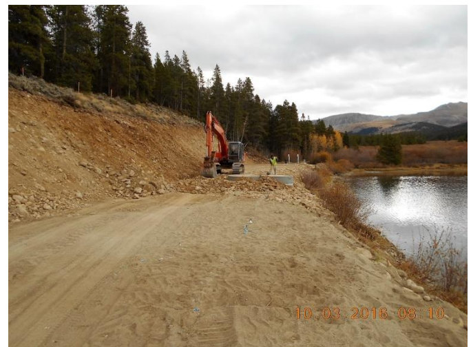
Slope Being Re-contoured
