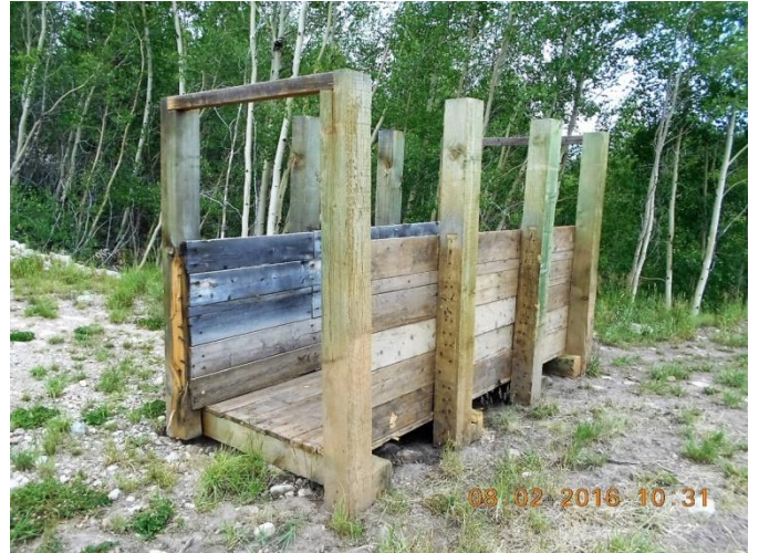
Display Section of Old Flume
