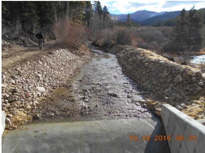
Water in Stream Entering Inlet Structure
