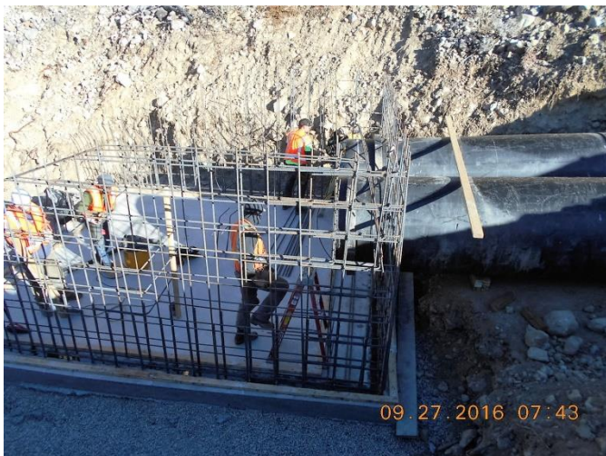
Outlet Structure Rebar Being Placed
