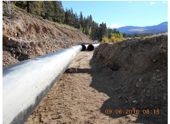
48" HDPE Pipes Being Placed In Trench
