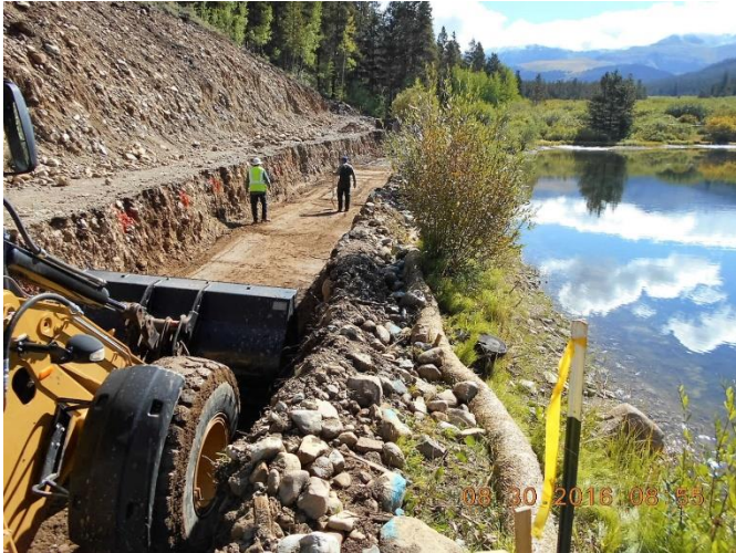
Pipe Trench Bedding Being Placed
