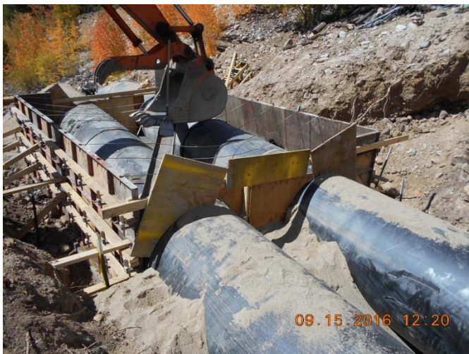
Lean Concrete Fill Area at Dam Abutment
