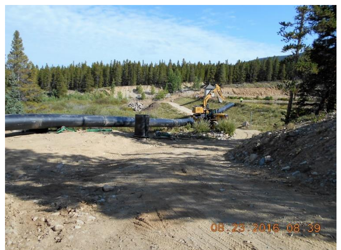
48" HDPE Being Staged Before Installation
