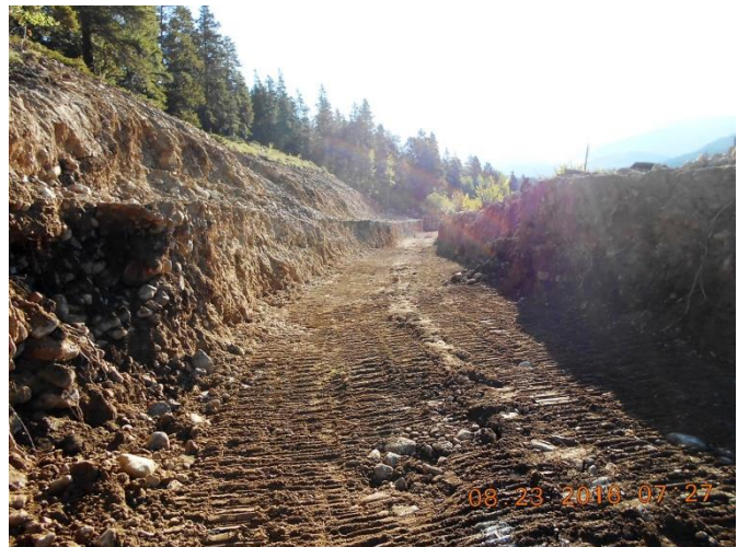
View of Rough Pipe Trench
