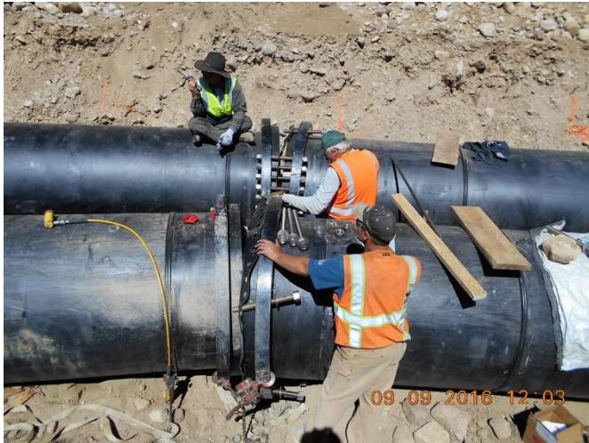
HDPE Flanges Being Made
