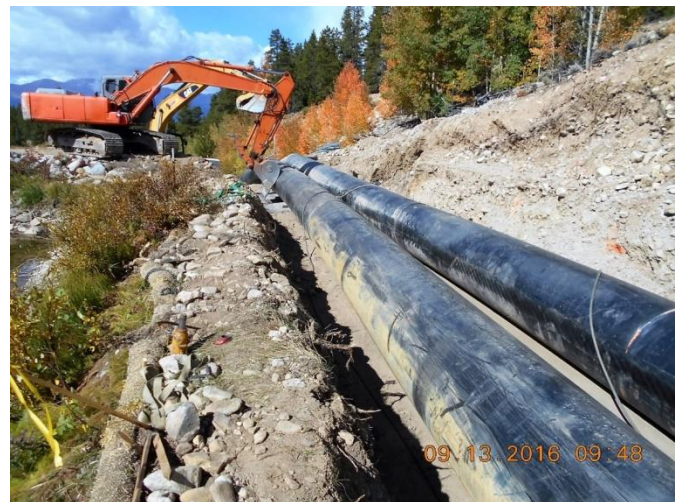
48" HDPE Pipes Being Positioned In Trench
