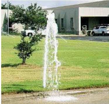
Geyser! (broken head)
