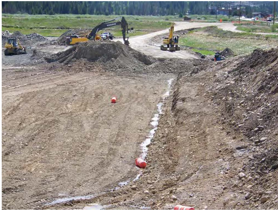
West berm excavation overview.
