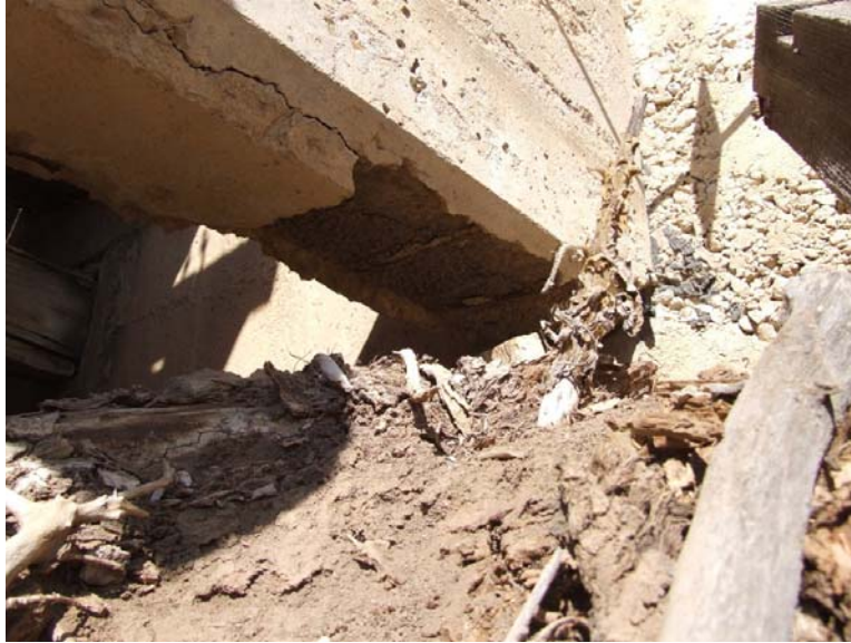
Figure 4. North end of eastern girder showing typical concrete cracking and spalling at bottom flange of encased steel beam.
