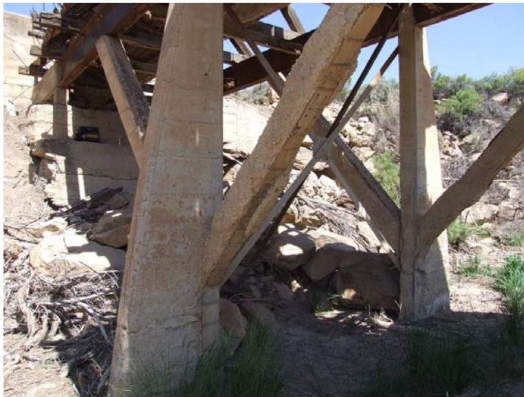
Figure 7. South diagonal brace of northwestern frame showing severe concrete spalling. Both top and bottom flanges are fully exposed.
