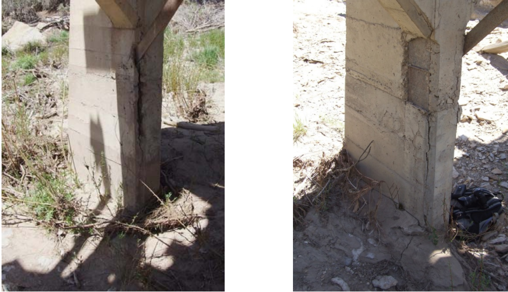
Figure 6. Spalling and concrete deterioration at base of columns. At left: southwestern column. At right: southeastern column.
