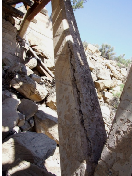
Figure 12. Concrete crack near top flange of encased steel element at north brace of northeastern frame. The crack extends for approximately 6 ft. Similar crack was observed at the north brace of the northwestern frame.
