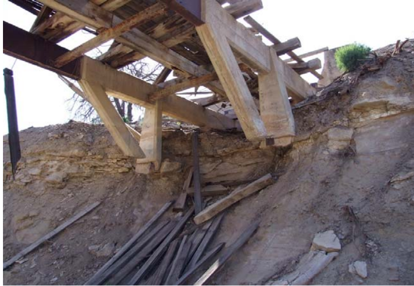
Figure 22. Unsupported piers and diagonal braces at south end of flume due to soil erosion.
