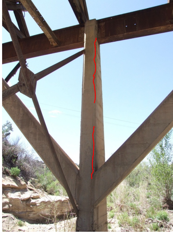
Figure 10. Typical vertical cracks (marked with red lines) at concrete columns. This photo shows the southwest frame, looking west.
