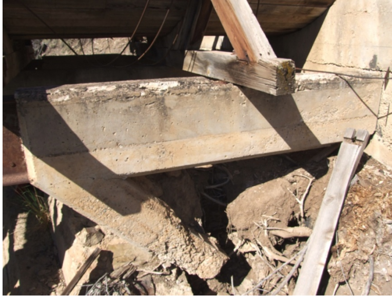
Figure 24. Diagonal brace without support at north end of east girder.
