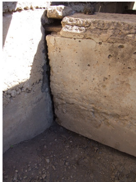
Figure 15. Corrosion at the girder inside the bearing pocket was observed. The empty cavity is likely to trap water and moisture, which will accelerate the corrosion process.
