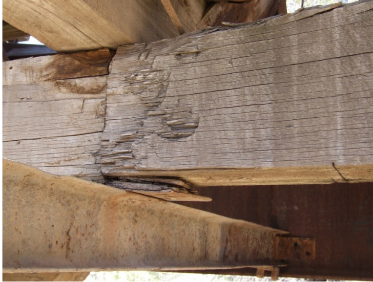
Figure 20. Typical severe corrosion affecting the stringers supporting plates. Note the amount of uplift experienced by the stringer due to the increase in steel volume.
