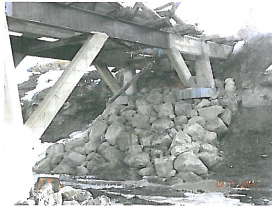
After: New Footers and protective rip rap.
