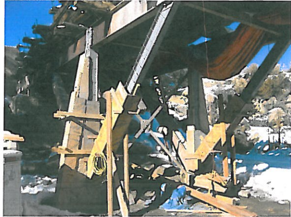
Formwork and steel preparation for new concrete
