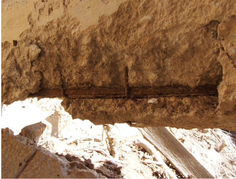
Figure 14. Moderate corrosion was observed at the portions of girders encased in concrete. This photo shows corrosion at the bottom flange of the east girder, near the north abutment. Note severe corrosion of metal ties.
