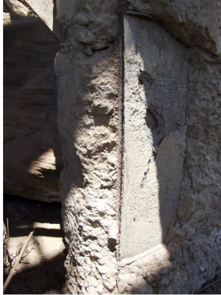
Figure 18. Severe corrosion at the flange of the encased column at the northeastern frame. 55% loss of original thickness was measured at this location.
