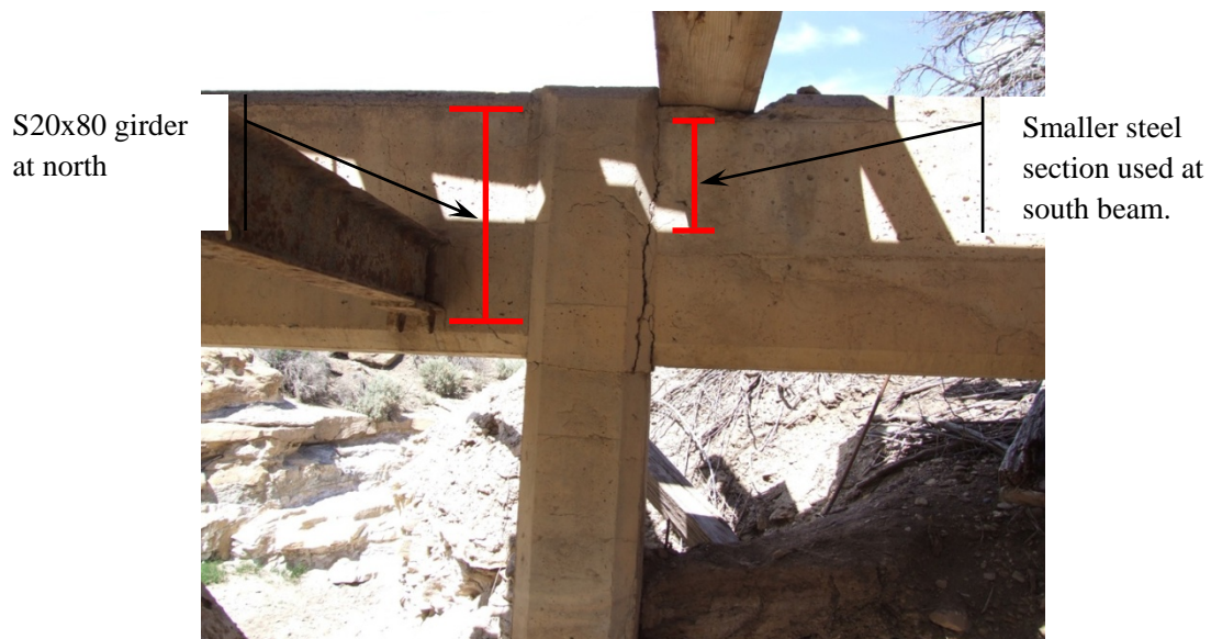
Figure 23. Flexural cracks at pier-girder connection at the south end of the flume. A smaller steel beam was used in the construction of the south beam that spans from the pier to the abutment (steel sections shown in red). The connection between the encased steel beams and column is likely a shear connection. Similar cracks were observed at the opposite pier.
