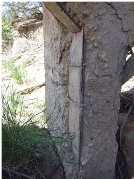
Figure 5. Spalling and concrete deterioration at base of columns. At left: northwestern column. At right: northeastern column. Severe distress conditions were observed at these locations.
