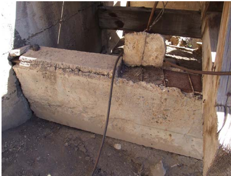
Figure 3. North end of western girder showing typical concrete cracking and spalling at top flange of encased steel beam.
