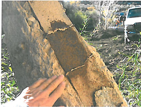
Deteriorated concrete and corroded steel
