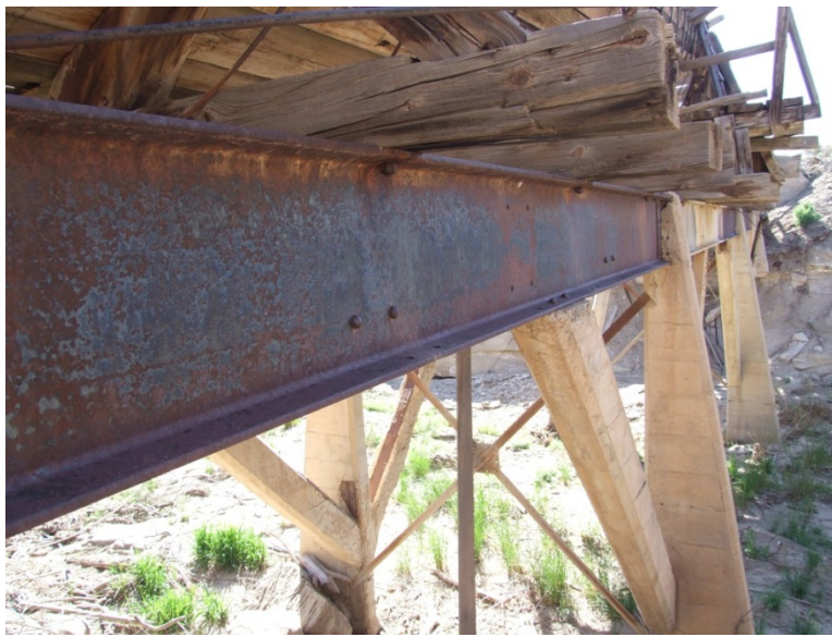
Figure 13. Minor surface corrosion affecting the majority of the steel girders exposed surface.
