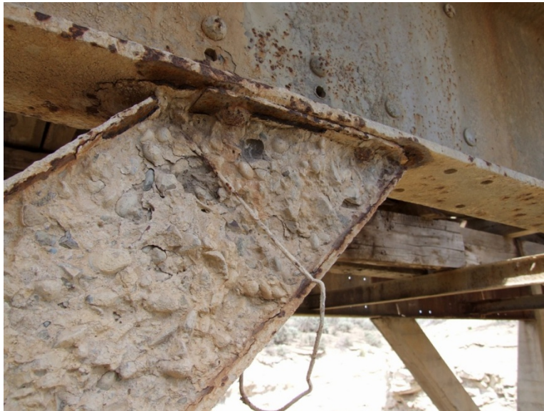
Figure 19. Typical corrosion at the diagonal brace-girder connection. The corrosion is particularly severe at the bottom surface of the girder's flange and the angle used to connect the two structural elements.
