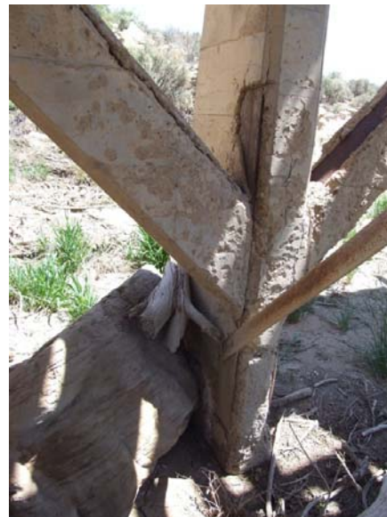
Figure 5. Spalling and concrete deterioration at base of columns. At left: northwestern column. At right: northeastern column. Severe distress conditions were observed at these locations.
