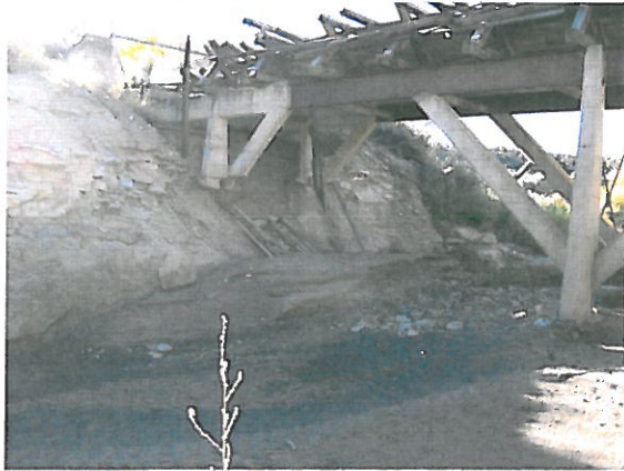
Before: Severely eroded foundation
