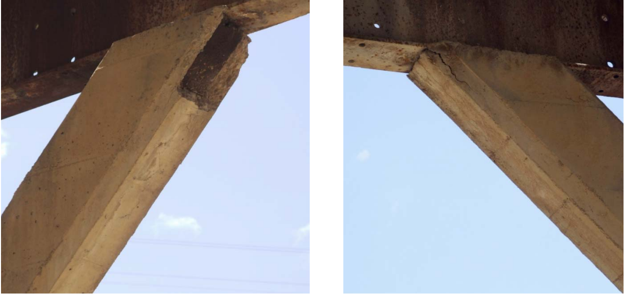
Figure 8. Typical spalling and concrete cracking at top of diagonal braces of southern frames.
