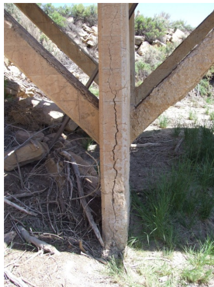
Figure 11. Large vertical crack at west side of northwestern column. The crack is likely due to corrosion of the vertical steel reinforcement that was located by Pachometer scanning.
