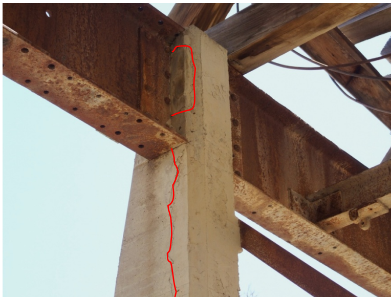
Figure 9. Typical concrete cracking (marked with red lines) at column-girder connection.
