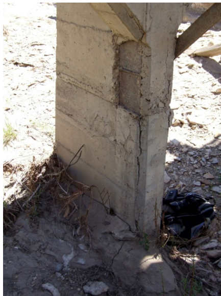
Figure 17. Typical minor corrosion at base of southern columns. At these locations, extensive concrete cracking with some spalling was observed.
