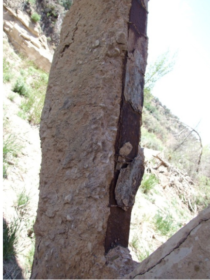
Figure 16. Severe corrosion at the south diagonal brace of the northeastern frame. 25% loss of original top flange thickness was measured at this location.
