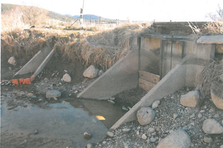
Fire Mountain Canal at turnouts to #80 and East Lateral
