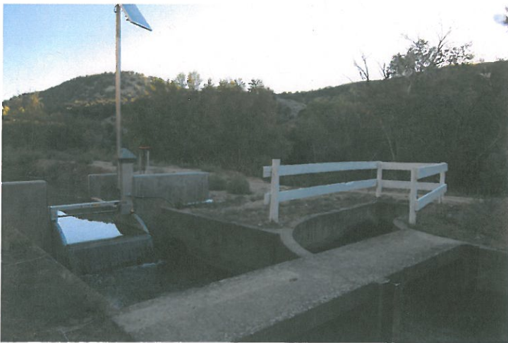
New SCADA gate at Leroux Creek return and siphon
