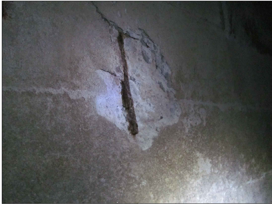
REBAR EXPOSED
