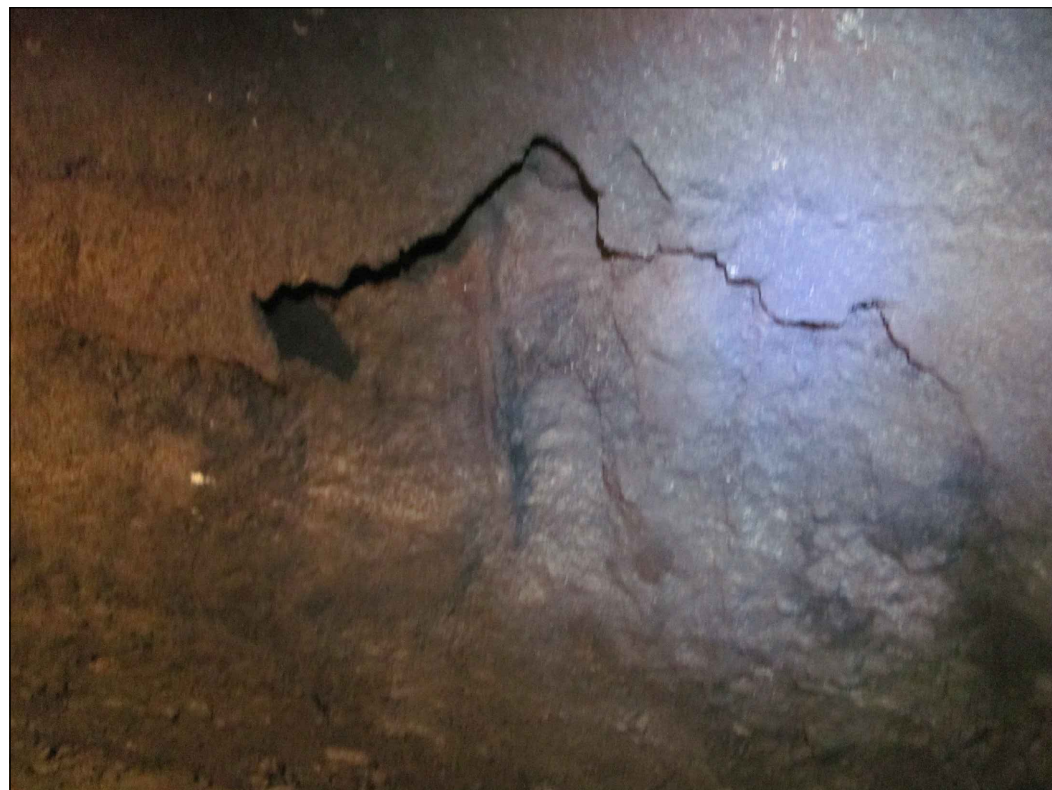
SPALLED PATCHES
