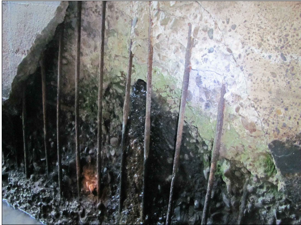
REBAR EXPOSED
