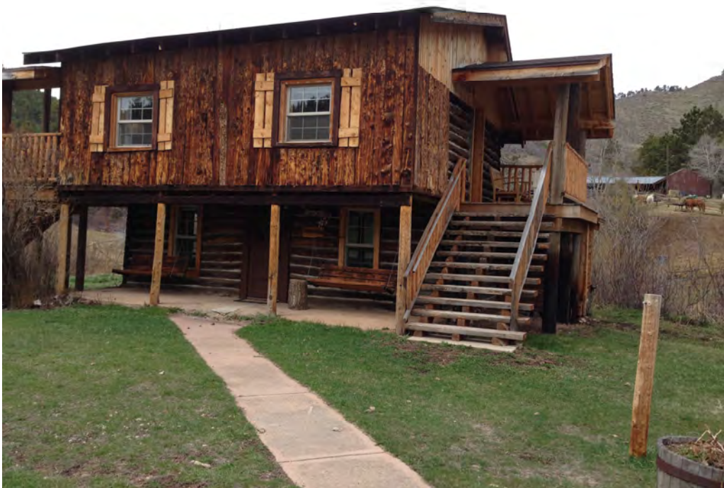
Photo 4 – Structure at Critical Section 17627.5
