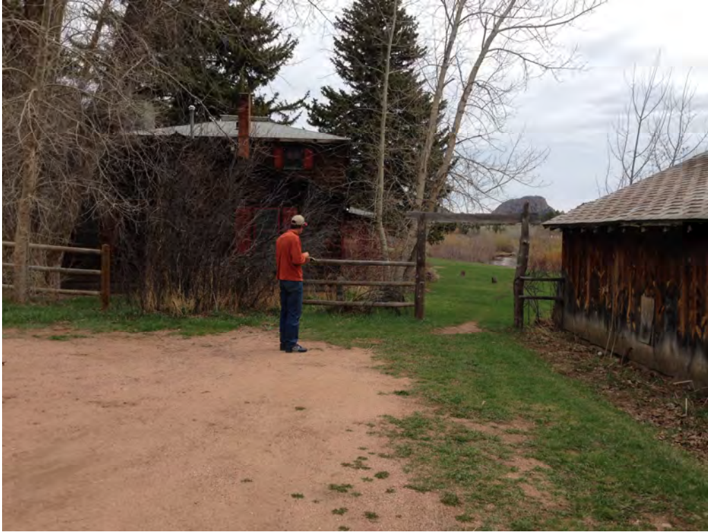
Photo 3 – Structures at Critical Section 17627.5
