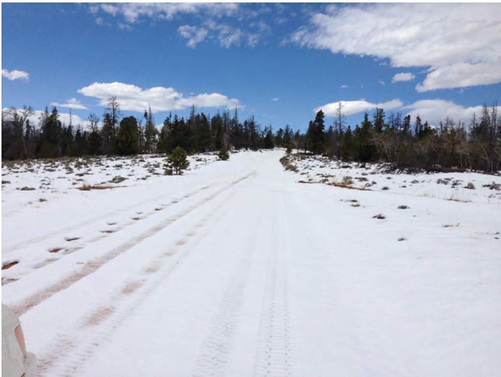
Photo 8 – Snow-covered access road to Worster Dam
