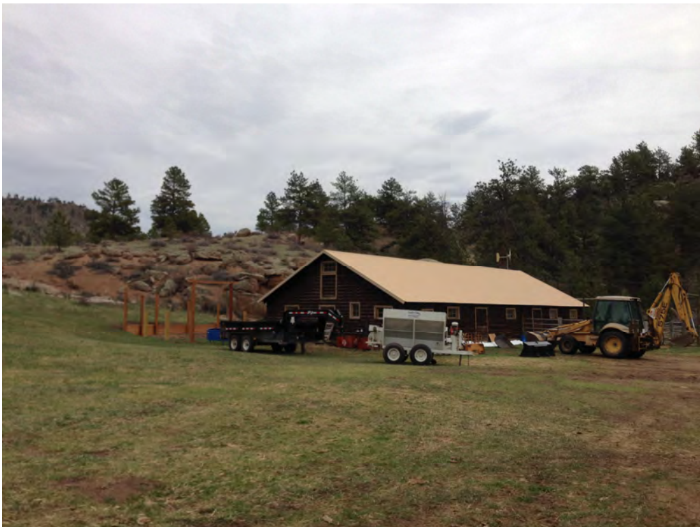
Photo 2 – Structure at Critical Section 16937.9
