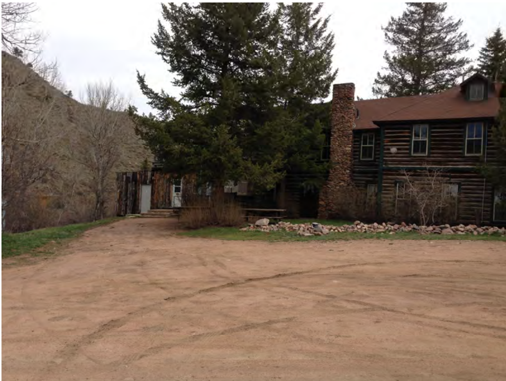
Photo 6 – Structure at Critical Section 20955.1
