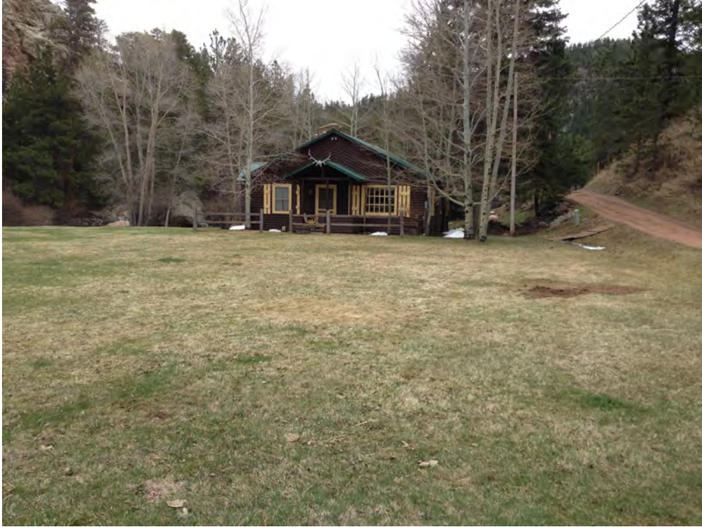
Photo 1 – Structure near Critical Section 16697.8
