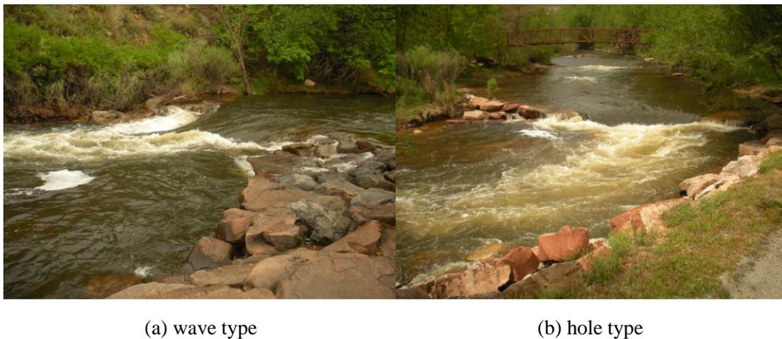
**Figure 2.2. Typical (a) “wave” and (b) “hole” types of WWP structures (Fox, 2013).**
