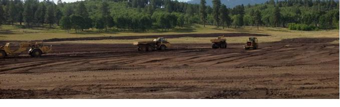
Over the course of the summer and fall, they excavated, processed, placed and compacted over 200,000 cubic yards of material taking the material from what would
