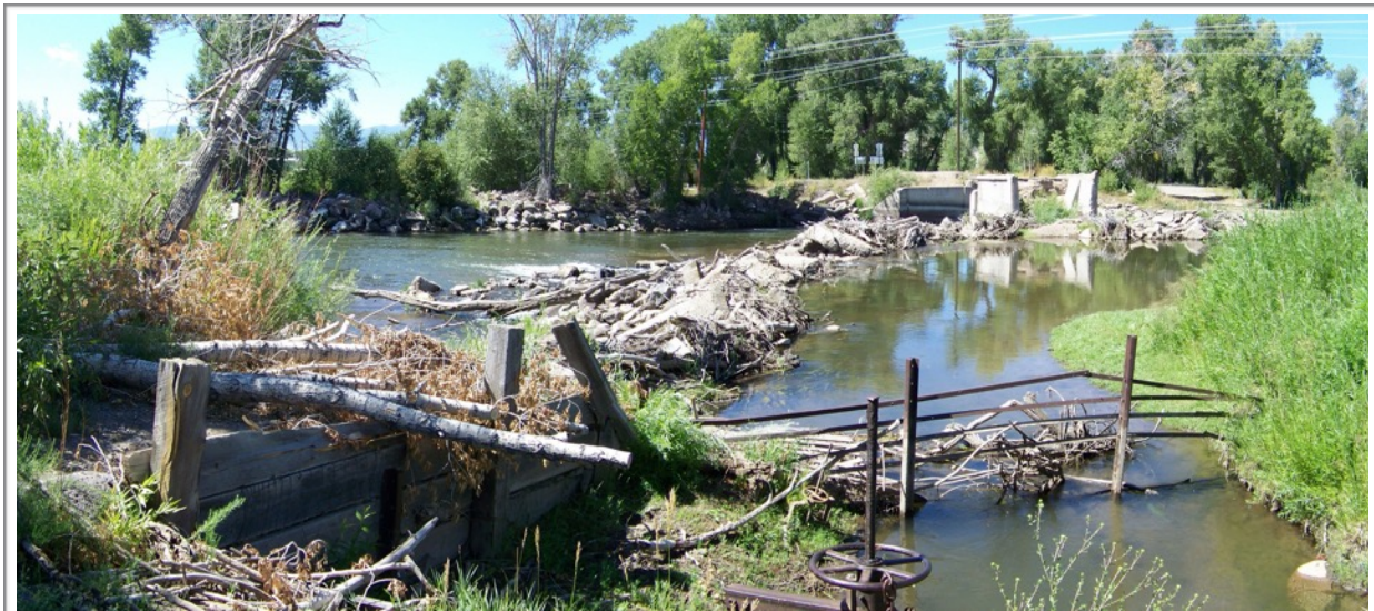
Figure 7: The Old McDonald Ditch Diversion Structure, which the McDonald Ditch will remove in 2016. Grade control and streambank stabilization will occur as shown in Figure 2.
