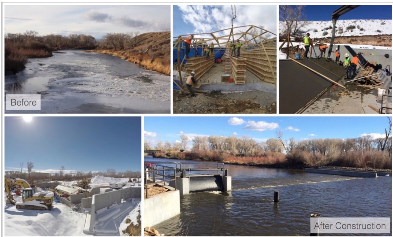
Figure 5: Construction of the new McDonald Ditch Diversion Dam.
