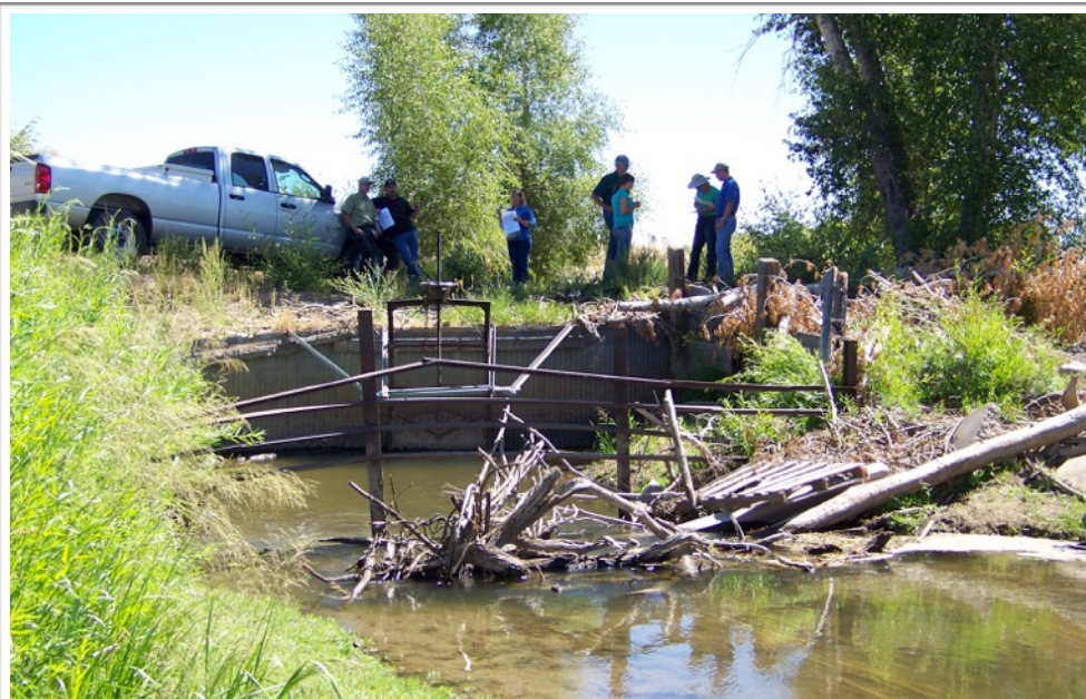
Figure 4: Site visit with NRCS Project engineers and partners.
