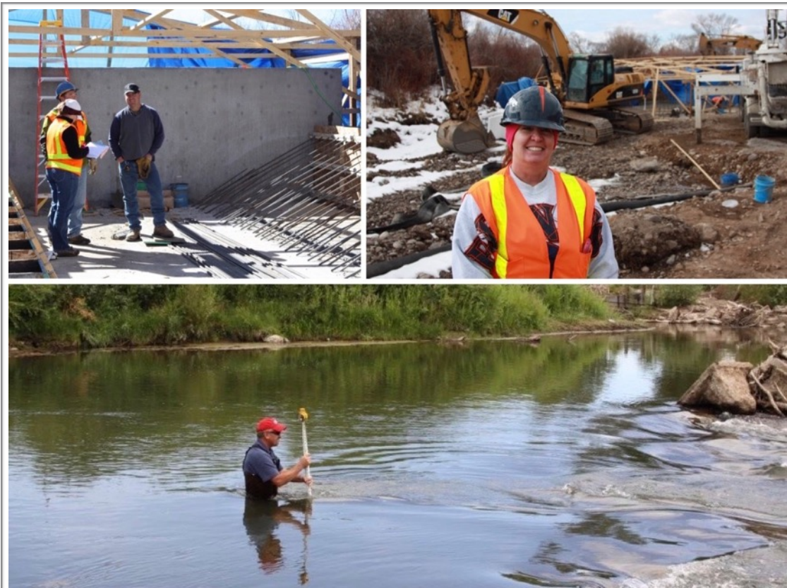
Figure 9: Phase 2 construction monitoring and surveying.
