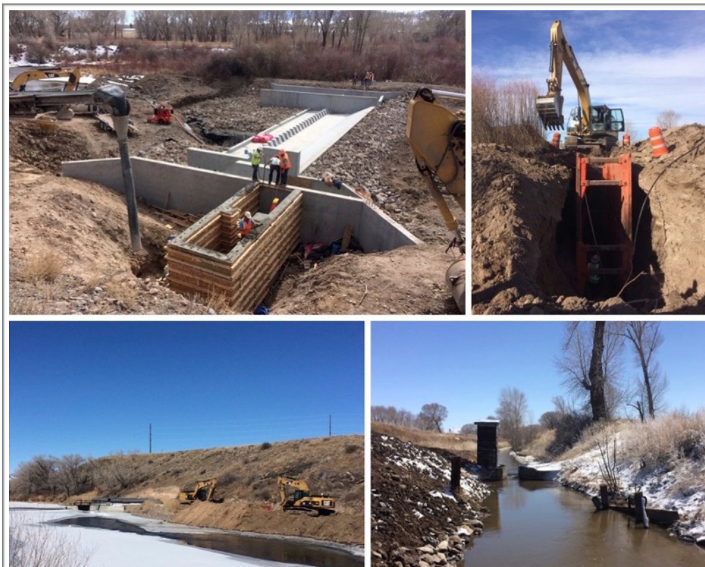
Figure 6: Construction of the McDonald Ditch Headgate and Pipeline, and the completed pipeline bringing water to the McDonald Ditch.
