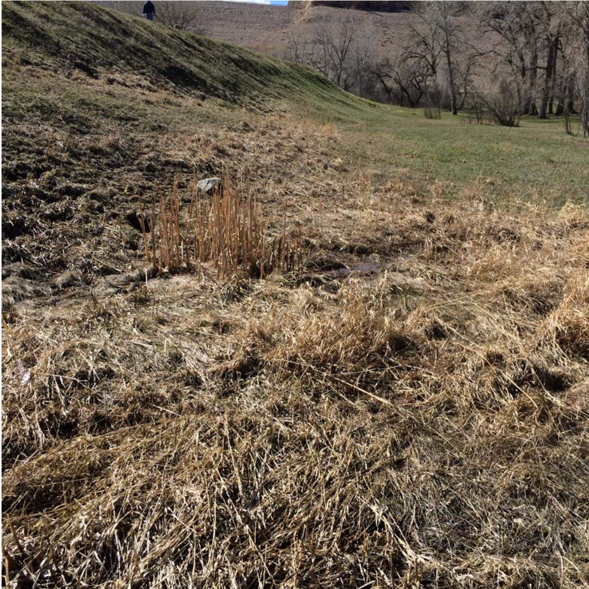
PHOTO 3 – SEEPAGE AREA LEFT OF OUTLET ON DOWNSTREAM SIDE OF DAM
