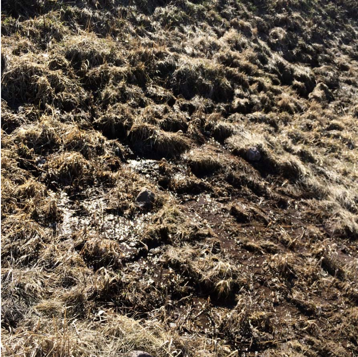
PHOTO 4 – ACTIVE SEEPAGE LEFT OF THE DAM OUTLET
