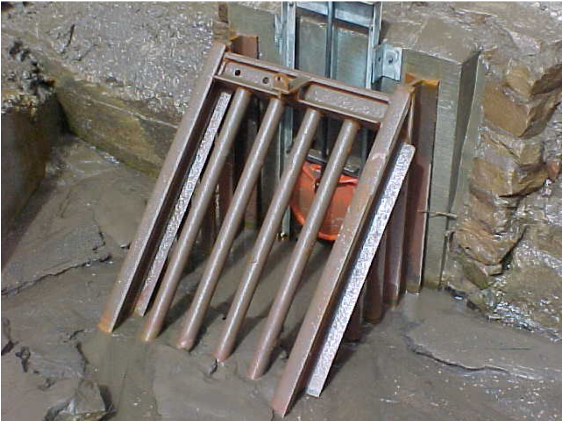
PHOTO 2 – EXISTING TRASH RACK AND 12" DIA. HEADGATE
