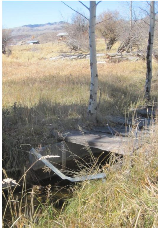
Photo 3: Ekhart Ditch Parshall flume.
