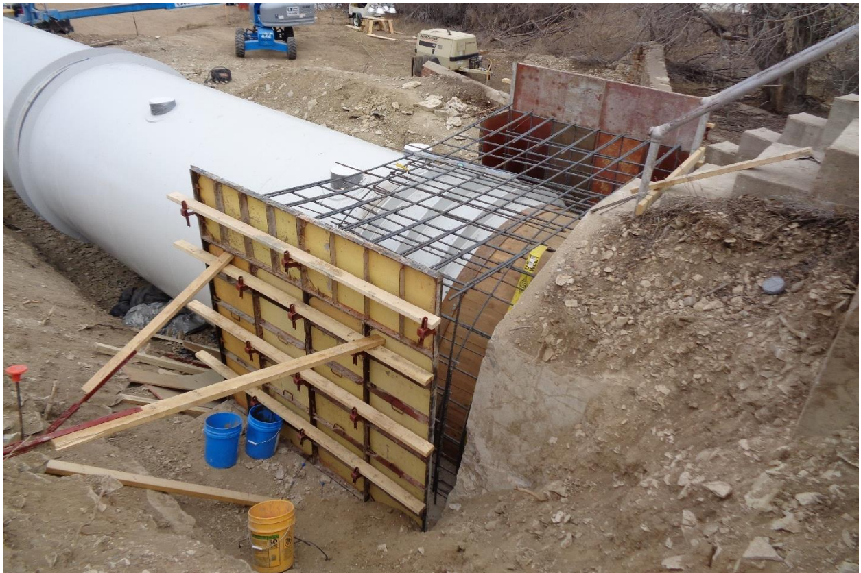
Figure 4 - Inlet Anchor Block
