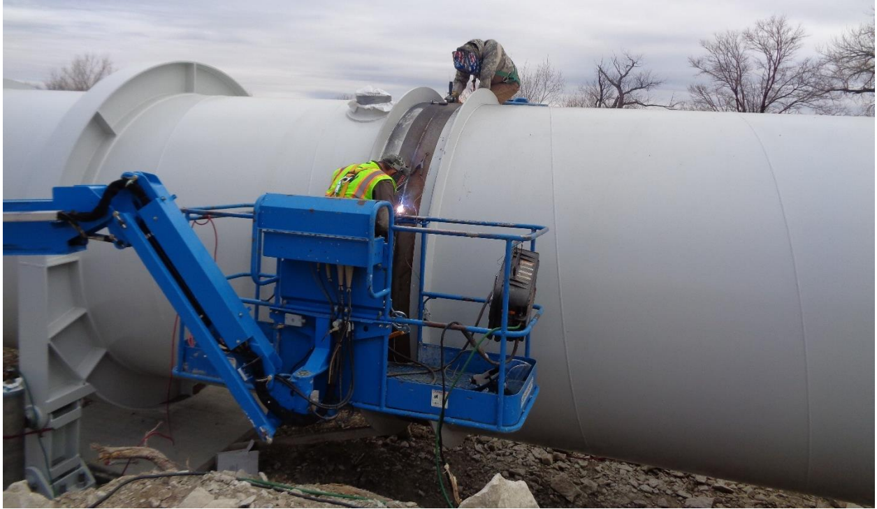
Figure 3 - Joint Weld (MK-2 to MK-3)
