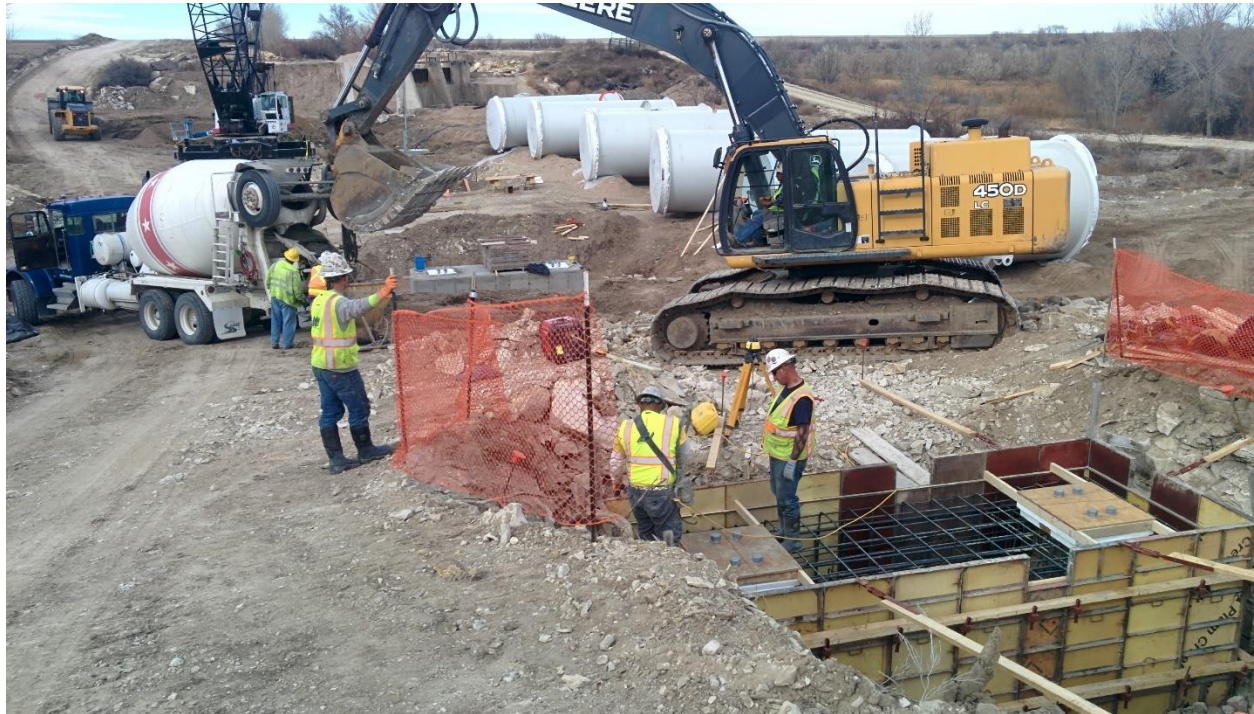
Figure 2 - Pier Installation (Pier 2 Rebar - Bottom, Pier 3 In Place – Top)
