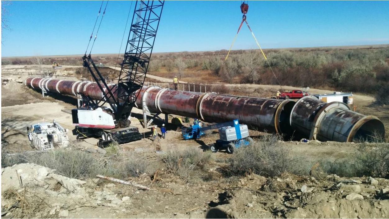
Figure 1 - Pipe Demolition
