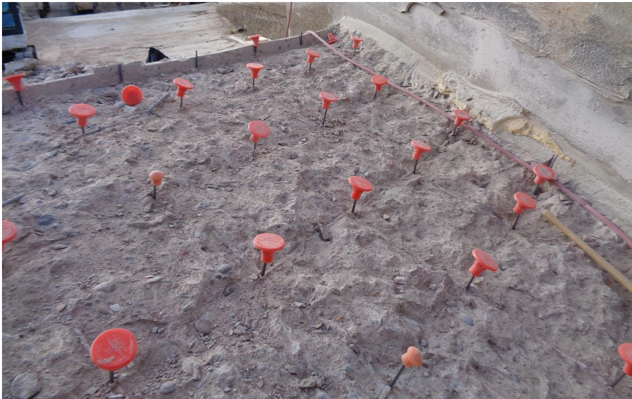
Figure 5 – Upper West Side Inlet Apron Dowels
