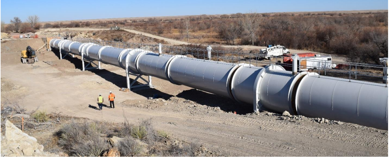
Figure 7 – Completed Pipe Prior to Leak Test
