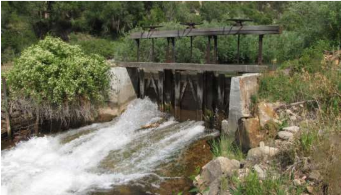
Figure 6: Existing headgate structure at beginning of Highland Ditch.
