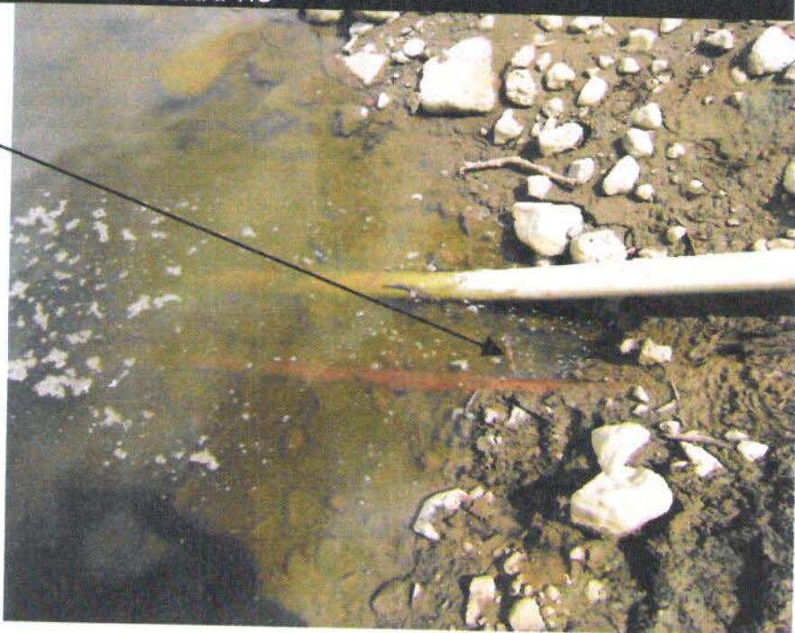
Photo 2 – Sinkhole on embankment slope at approximately gage height 2.8-ft.
