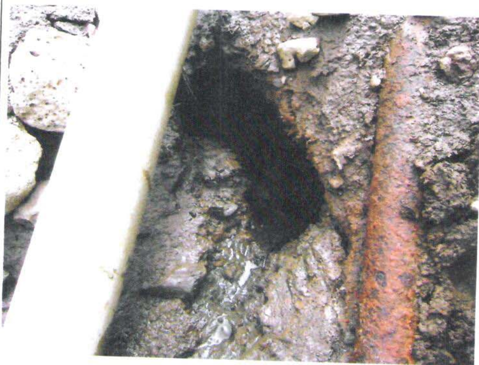
Photo 5 – Close up of flow from reservoir into sinkhole.
