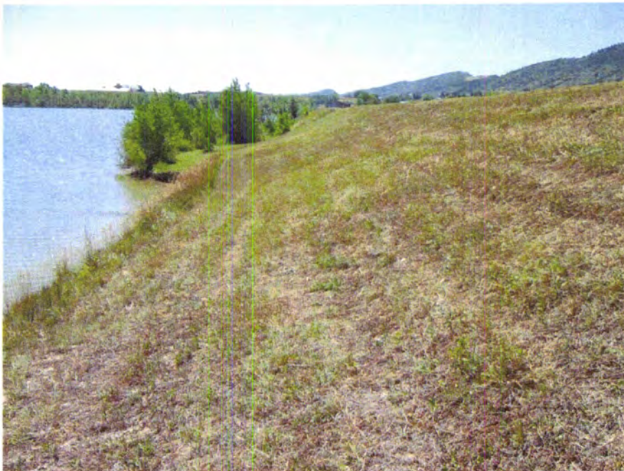
PHOTO C2 – Downstream slope of the dike, looking south. Overall condition of the slope is acceptable. Bergen Reservoir No. 2 is at left side.
