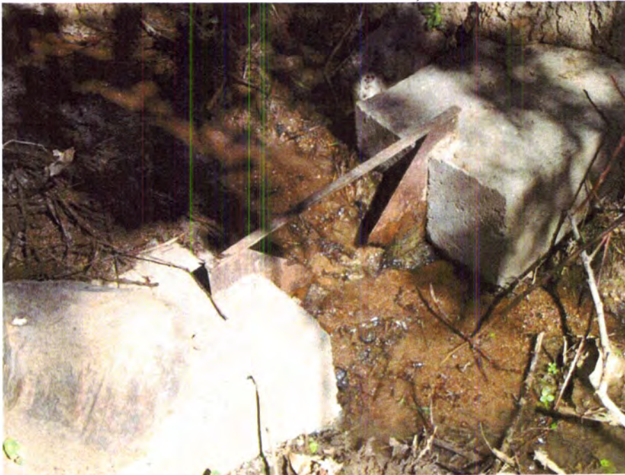
PHOTO B11 – Weir No. 2 just downstream of a 6-inch tile drain. Significant Sediments were accumulated between the weir and the tile drain.
