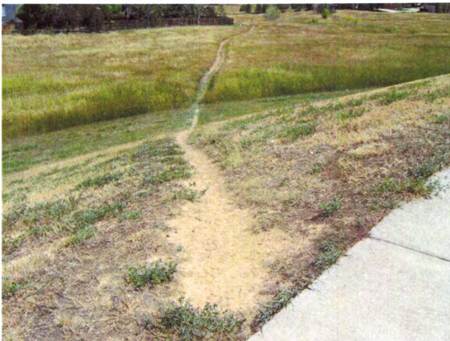
PHOTO D4 – View of the downstream slope of the dam, looking downstream, showing minor erosion of the slope face from a second footpath on the slope.
