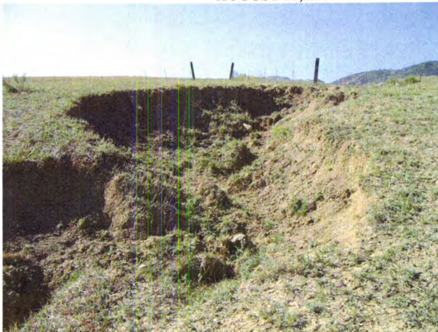
PHOTO B17 – Erosion in spillway discharge area, downstream of the downstream cutoff wall. This erosion area is at least 200 feet from the dam, and is not a dam-safety problem.
