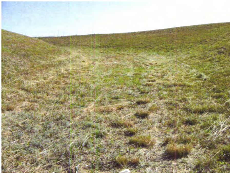
PHOTO B16 – Spillway discharge channel downstream of control sill, looking downstream. Low areas were reported in this channel. Otherwise channel is in good condition.
