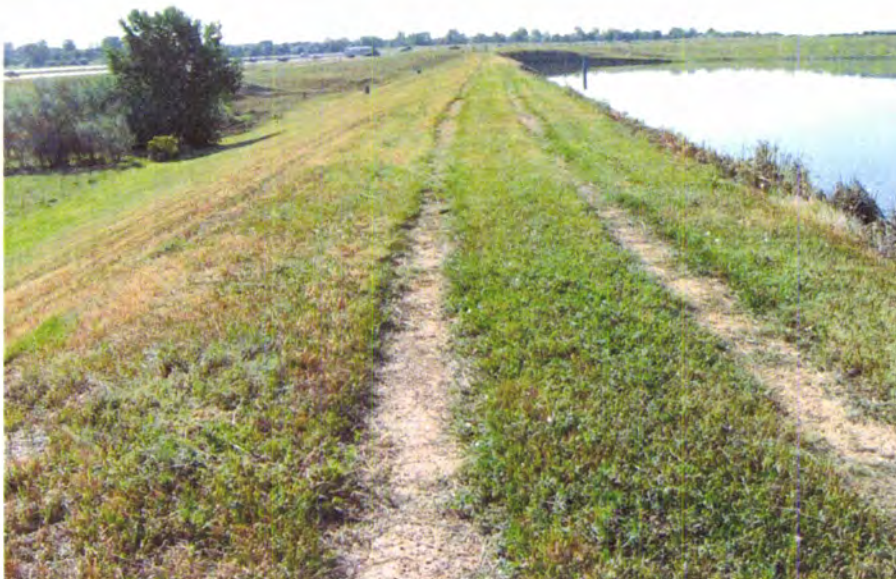
PHOTO B6 – General view of the dam crest, looking east toward the right abutment. Note minor ruts on the grass-lined crest surface.
