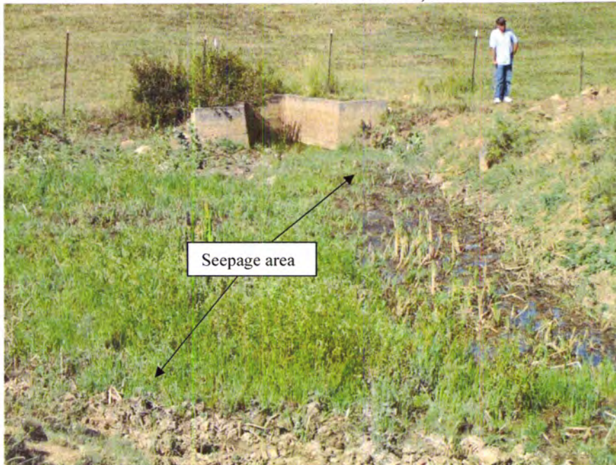
PHOTO B9 – Seepage area at the downstream toe of the dam just downstream of the outlet works discharge.
