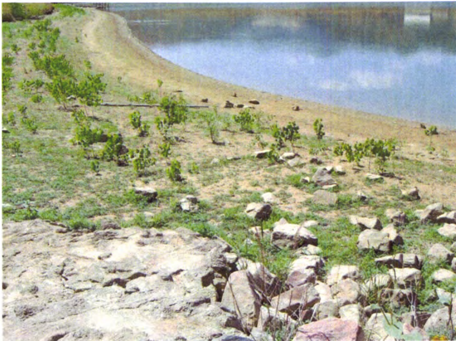
PHOTO D12 – Spillway approach channel, looking upstream. Note numerous tree saplings in the channel.
