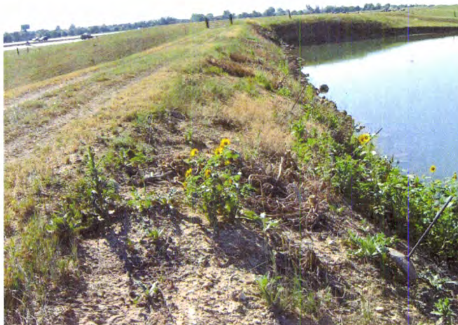
PHOTO B4 – View of the upstream slope near the right abutment. This area of the slope has no riprap protection and showed evidence of slumping and cracking.
