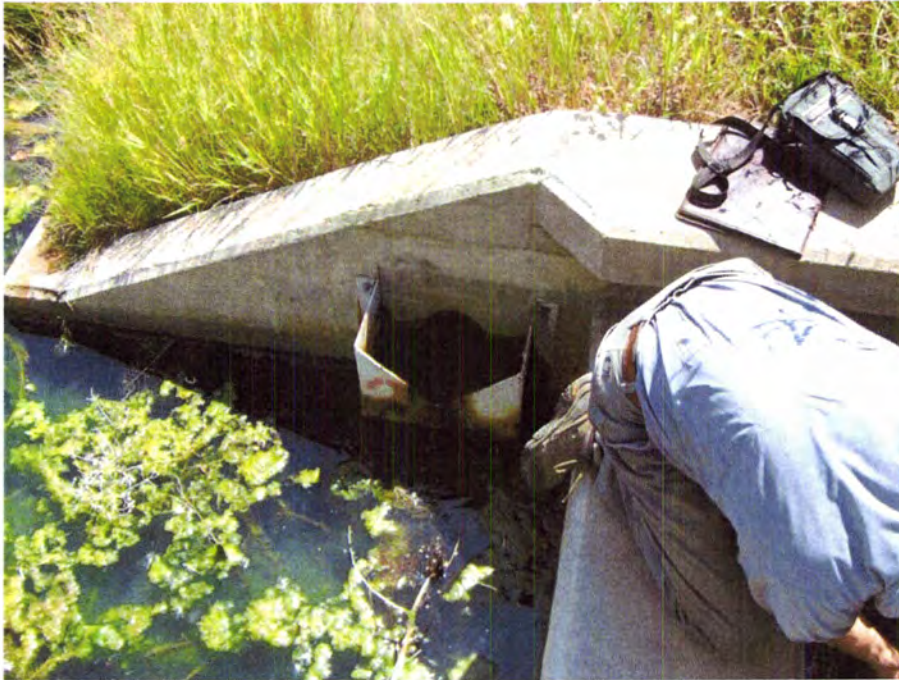
PHOTO D7 – Typical seepage weir mounted on the outlet basin. Note rusting of the weir coating. Also note the backwater in the outlet channel has submerged the entire outlet pipe.
