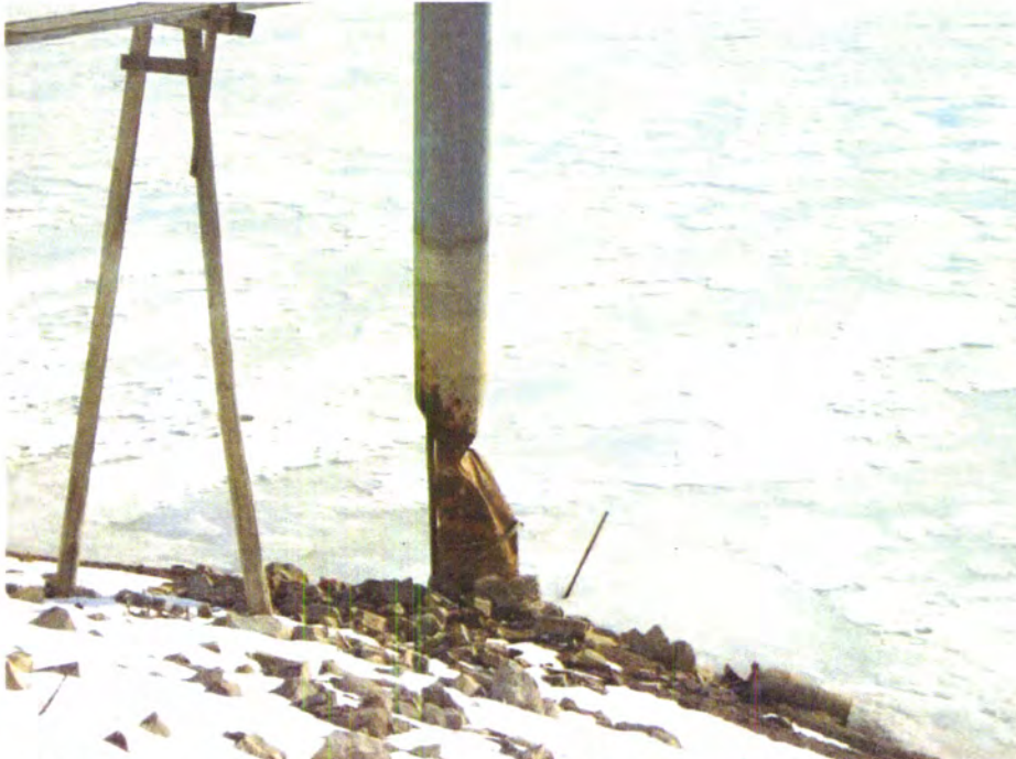
PHOTO B14 – Condition of the damaged riser structure of the outlet works. (Photo was taken on January 11, 2007 during low reservoir level, courtesy of W. W. Wheeler & Associates).
