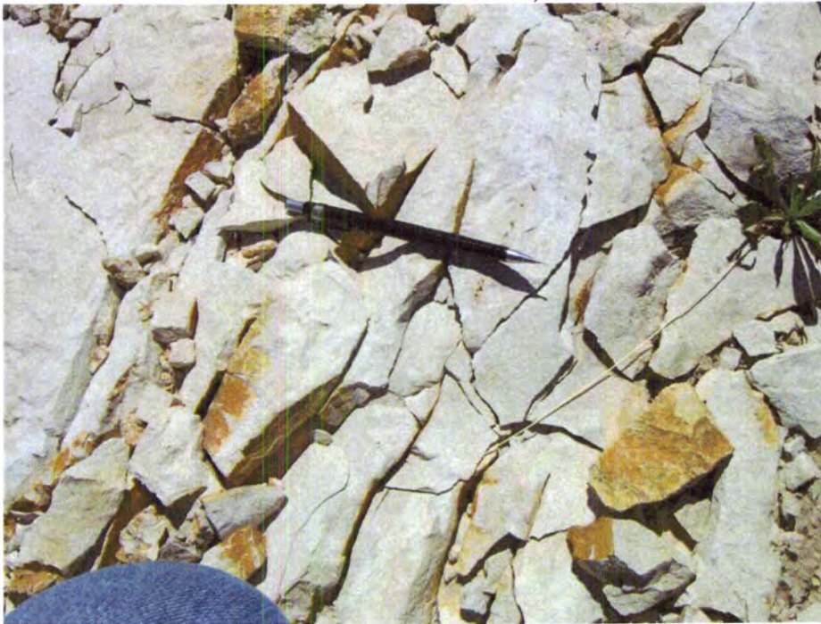
PHOTO C9 – Closeup of the bedrock condition on the emergency spillway of Bergen Dam No. 1.
