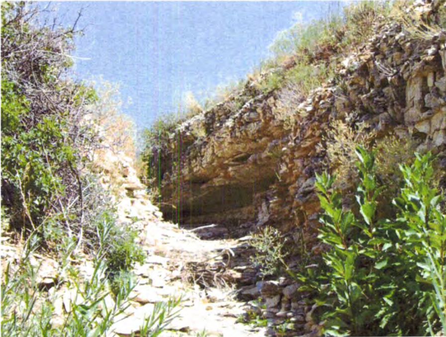
PHOTO C7 – Exposed limestone bedrock along the service spillway discharge channel.
