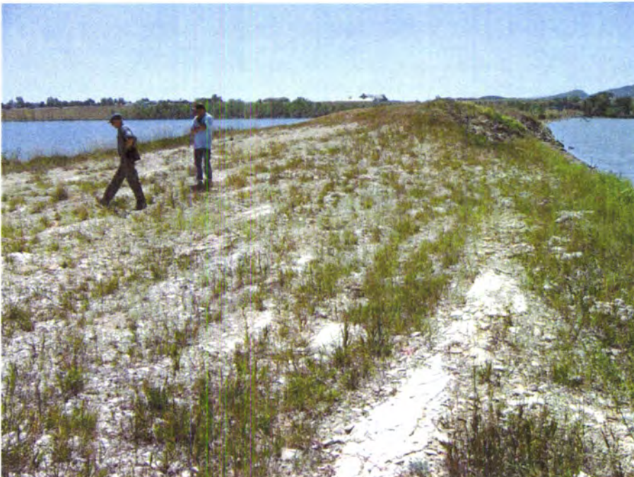
PHOTO C8 – Emergency spillway for Bergen Dam No. 1 at the south abutment of the dike, looking south. The condition of the rock spillway (limestone) is good.
