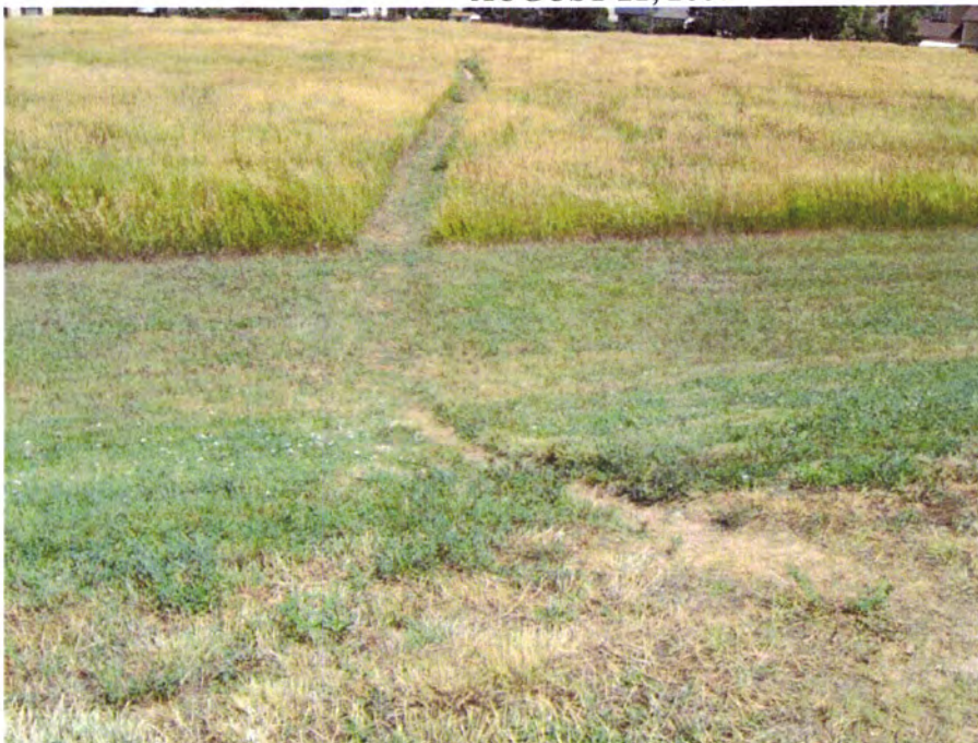
PHOTO D3 – View of the downstream slope of the dam, looking downstream, showing minor erosion of the slope face from pedestrian foot traffic.
