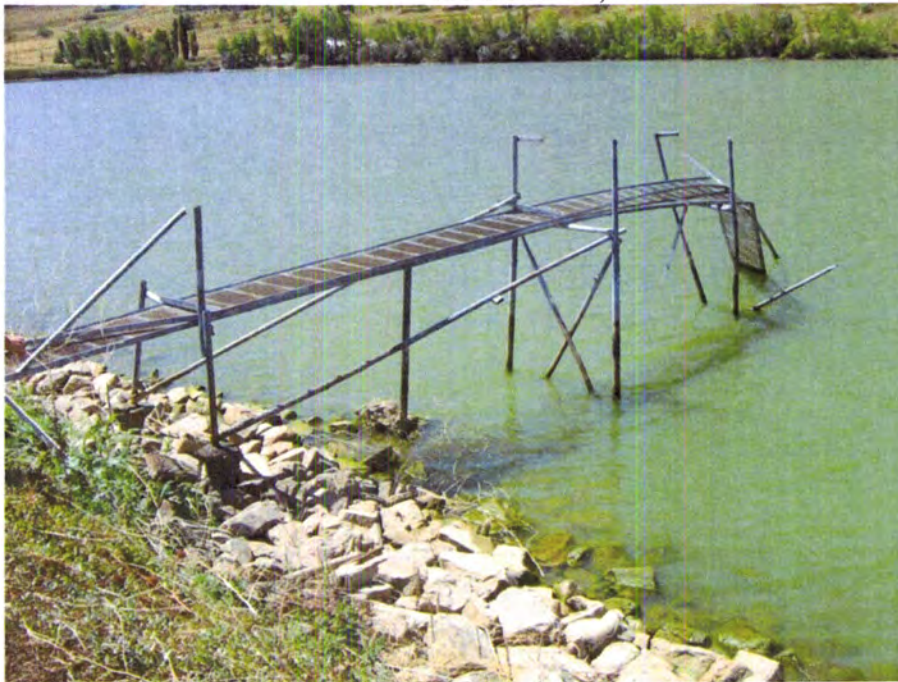
PHOTO C5 – Damaged walkway of the outlet works. The riser structure cannot be observed.
