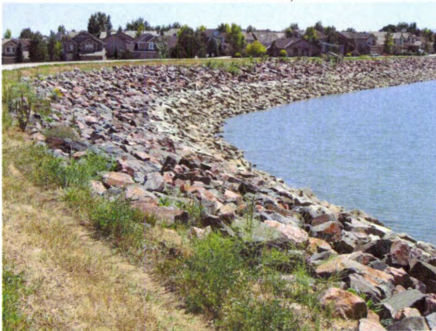
PHOTO D1 – General view of the upstream slope, looking toward the right abutment. The slope and riprap protection are in good conditions.
