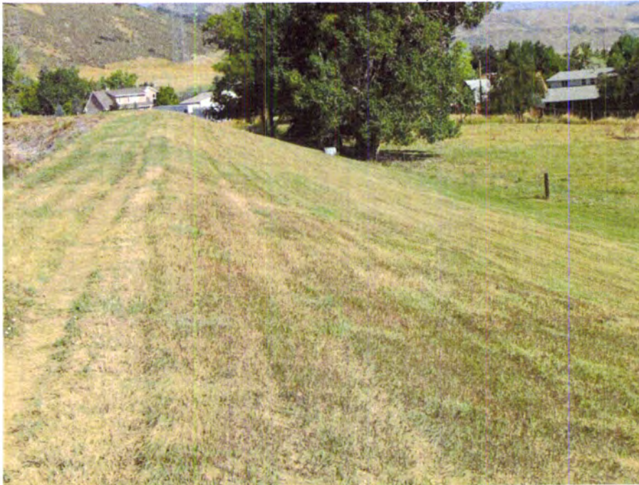
PHOTO B7 – View of the downstream slope, looking west toward the left abutment. The downstream slope is well maintained and in good condition.
