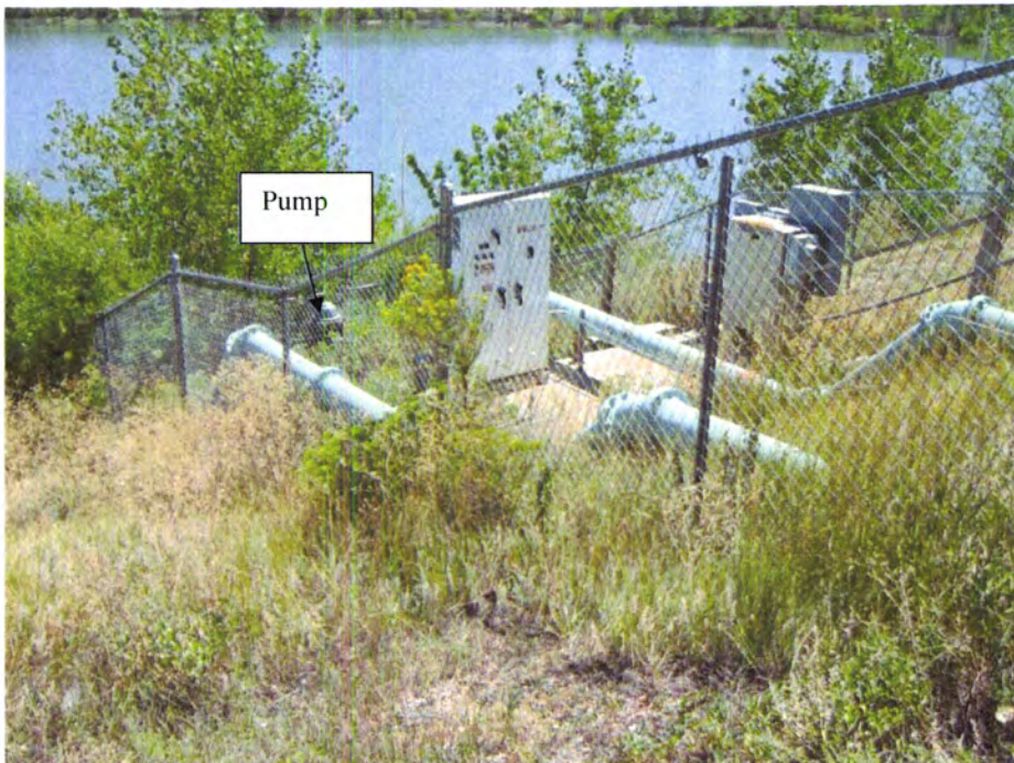
PHOTO C10 – Pumping facility on the north abutment of the dike. Bergen Reservoir No. 2 is in the background.
