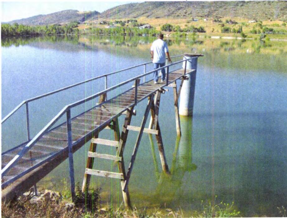
PHOTO B13 – Outlet works walkway and riser structure. Note the tilting of the riser structure.
