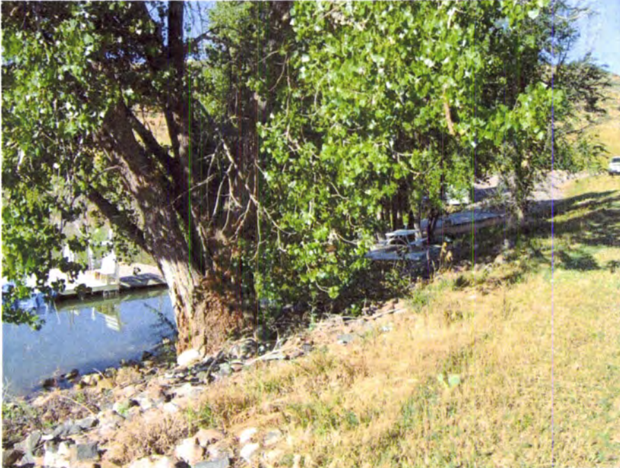
PHOTO B5 – Upstream slope near the left abutment. Note several trees growing on the slope in this area.
