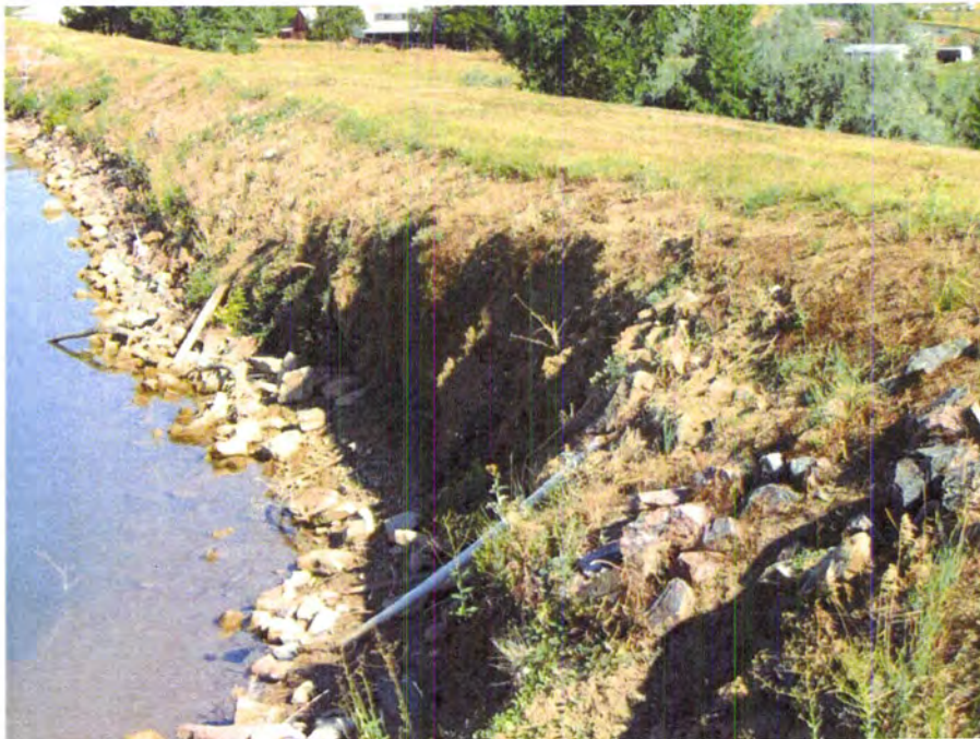
PHOTO B2 – View of upstream slope near the right abutment, looking toward the left abutment (west). Note near-vertical erosion scarp at the top 8 to 10 feet of the slope.
