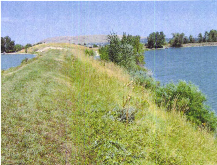
PHOTO C3 – Downstream slope of the dike looking south. This area of the slope is locally steep and includes some woody vegetation.
