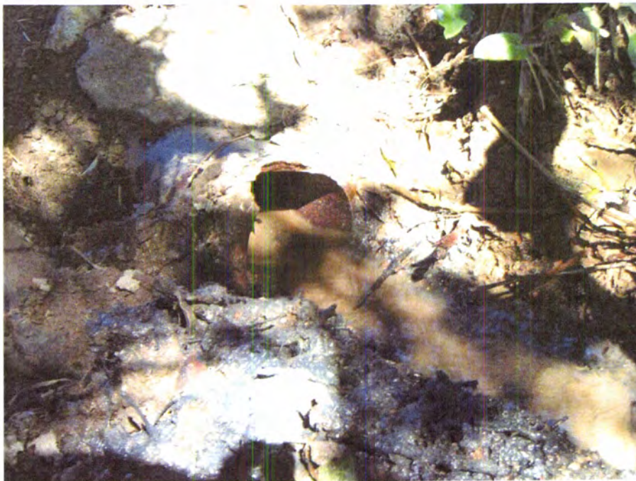
PHOTO B12 – Exposed 6-inch tile drain flowing about several gallons per minute. Sediments were observed at the bottom one-third of the drain. Cloudy water was caused by attempt to remove the sediments, and water became clear shortly thereafter.
