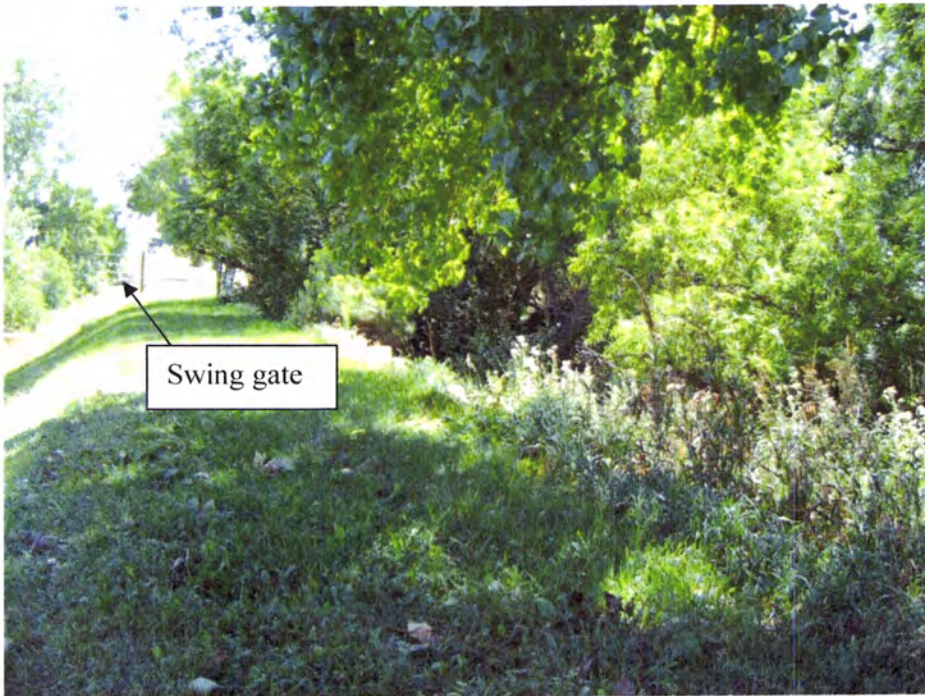
PHOTO A2 – View of upstream slope west of the swing gate, looking toward the right abutment. Note heavy vegetation on the embankment slope.
