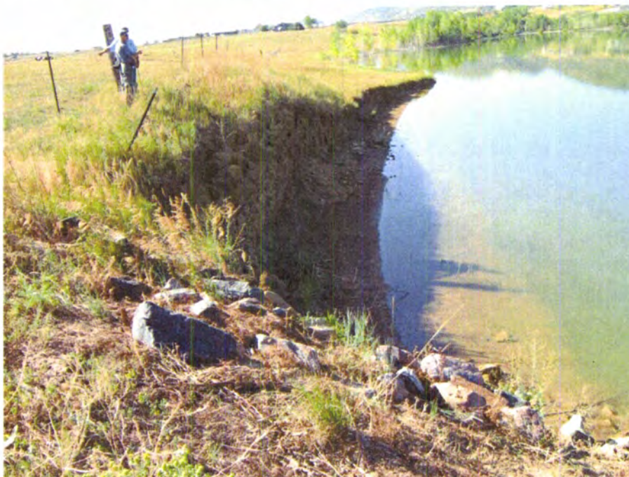
PHOTO B8 – Vertical scarp in the upstream right abutment just upstream of the dam.
