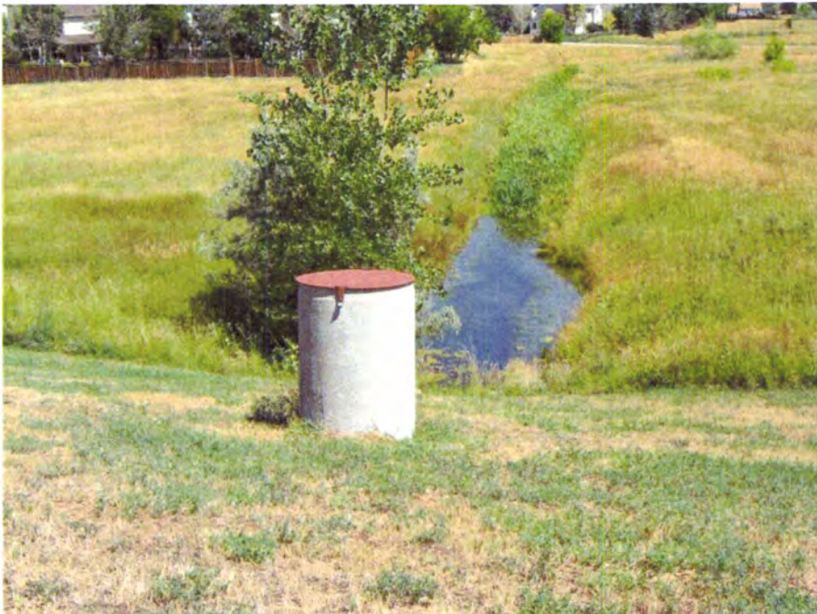
PHOTO D6 – View of the downstream toe of the dam at the outlet works discharge, looking downstream. Note drain manhole on the slope, outlet channel, and tree at the toe of the dam.
