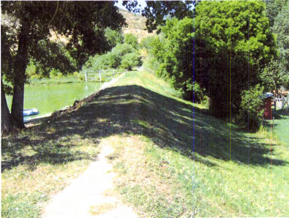
PHOTO A3 – View of dam crest and downstream slope, looking from the right abutment. Note heavy vegetation along entire toe of dam.
