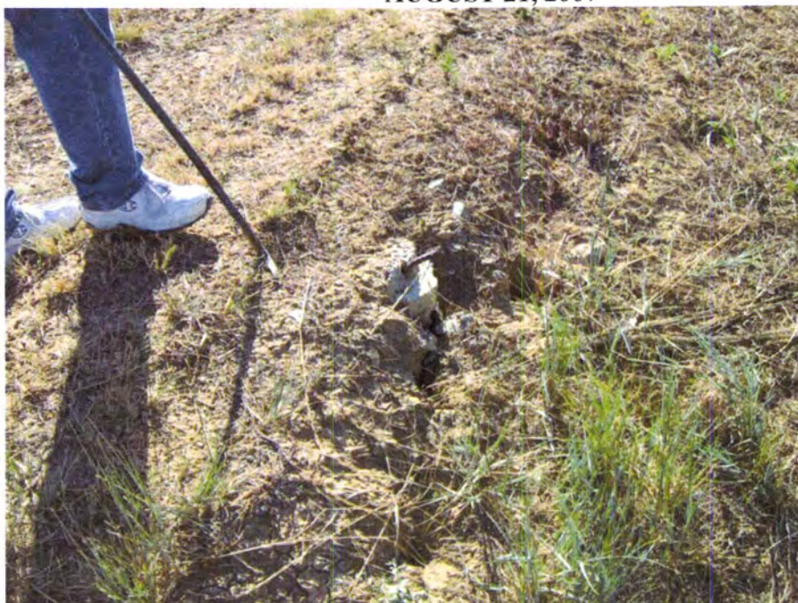
PHOTO B3 – Closeup of longitudinal crack at the top of the upstream slope near the right end of the embankment.
