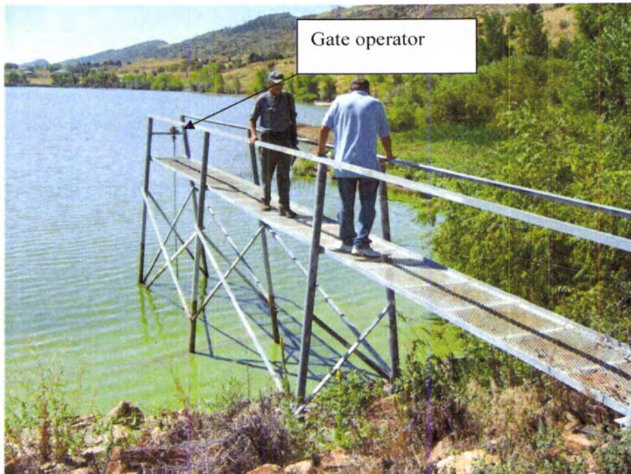
PHOTO A6 – Outlet works walkway. Note gate operator at the end of the walkway.
