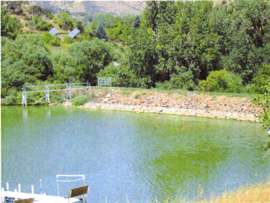
PHOTO A1 – View of upstream slope of the embankment and access walkway for the outlet works. The upstream slope and riprap protection are in good conditions.
