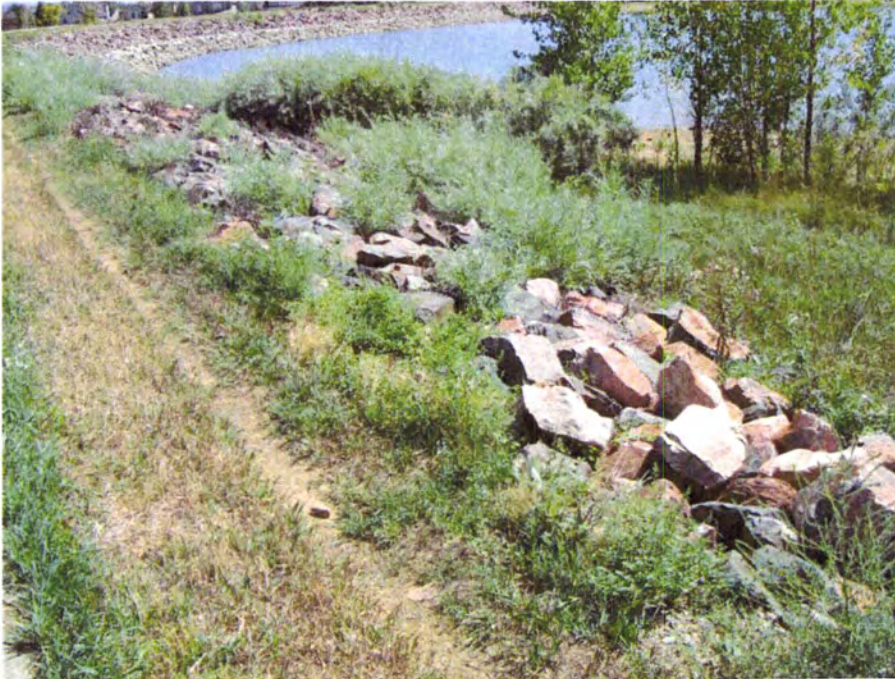
PHOTO D5 – View of the upstream left abutment and left end of the dam. Note minor vegetation on the upstream slope among the riprap.
