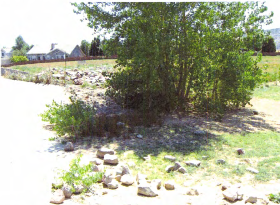
PHOTO D10 – Spillway approach channel, right side. Note several grown trees in the channel.
