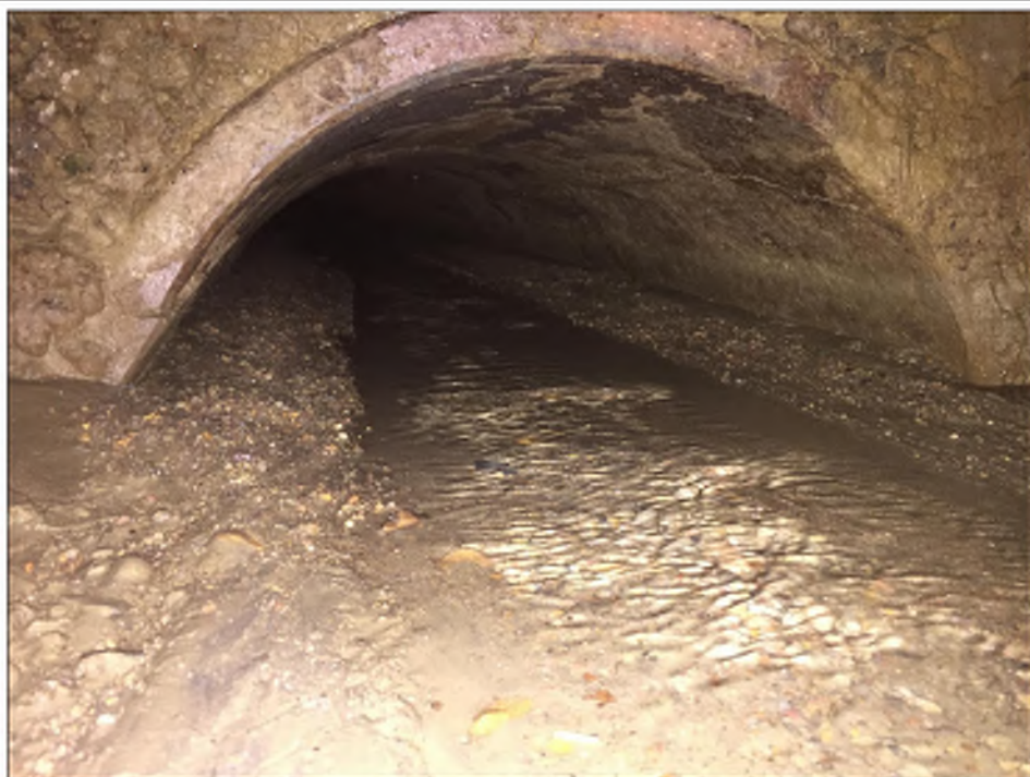
PHOTO 3 - NORTH 24" DIAMETER VCP OUTLET WORKS PIPE
