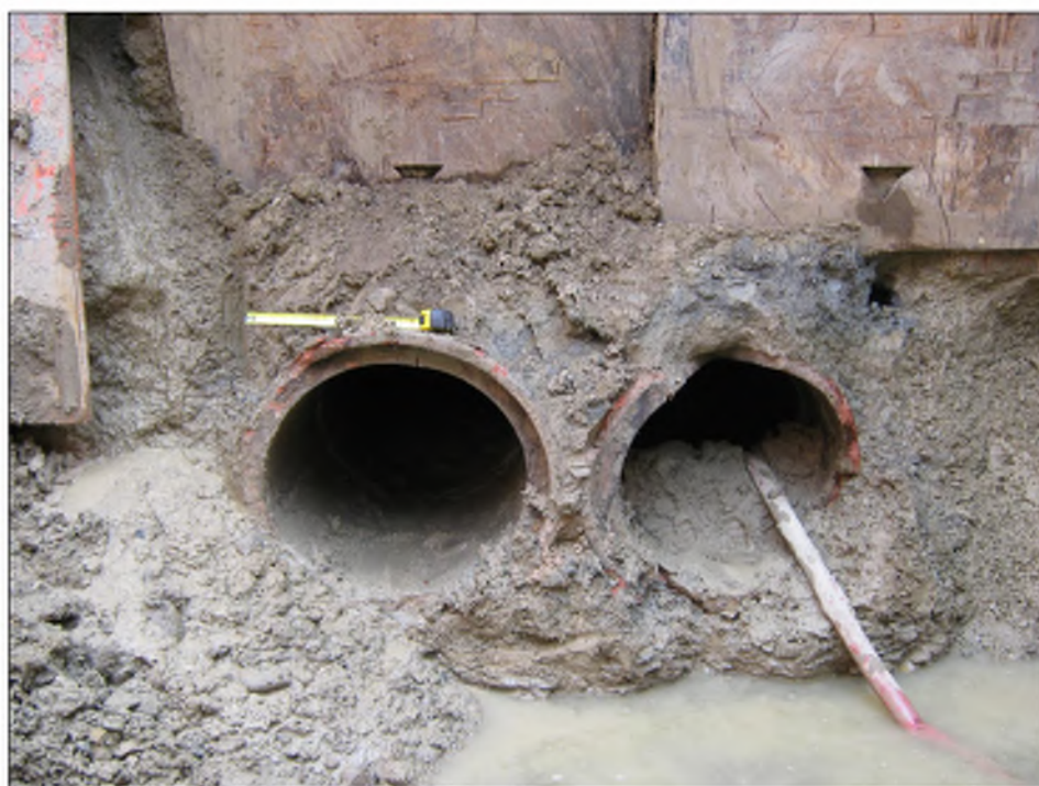
PHOTO 2 - WEST END OF THE 2-(24") VCP OUTLET WORKS PIPES
