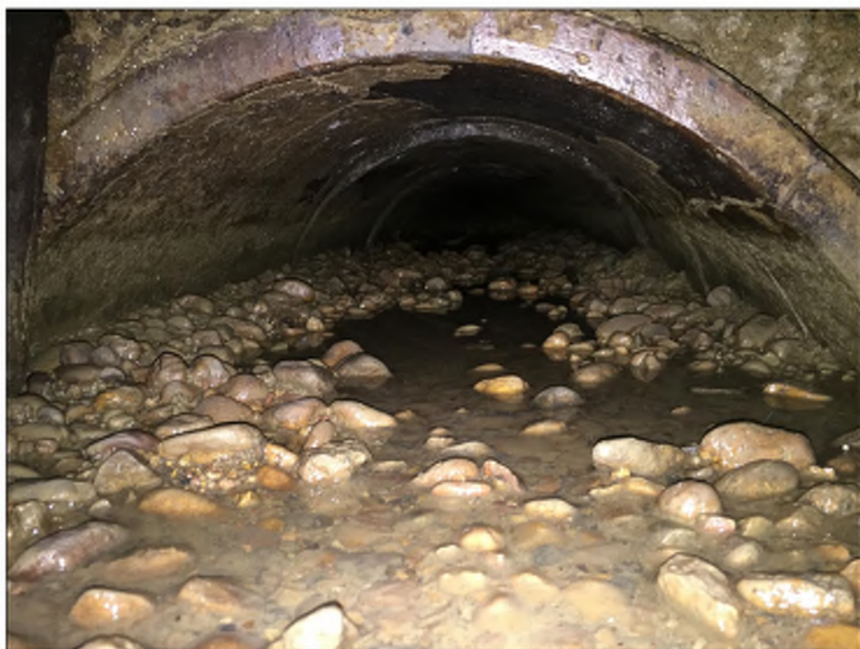
PHOTO 4 - SOUTH 24" DIAMETER VCP OUTLET WORKS PIPE
