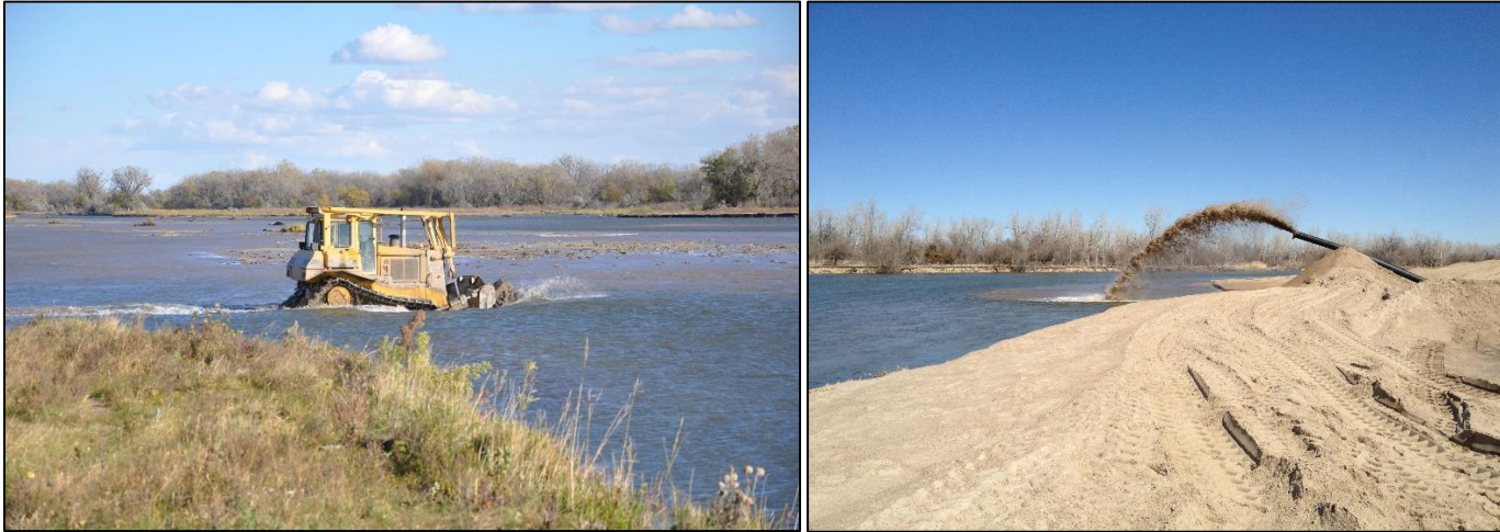
Figure 3. Example of mechanical augmentation (left) and sand pumping augmentation (right). Mechanical augmentation provides the ability to distribute sediment evenly across the channel. Point-source sand pumping produces limited capacity to entrain augmented material.
