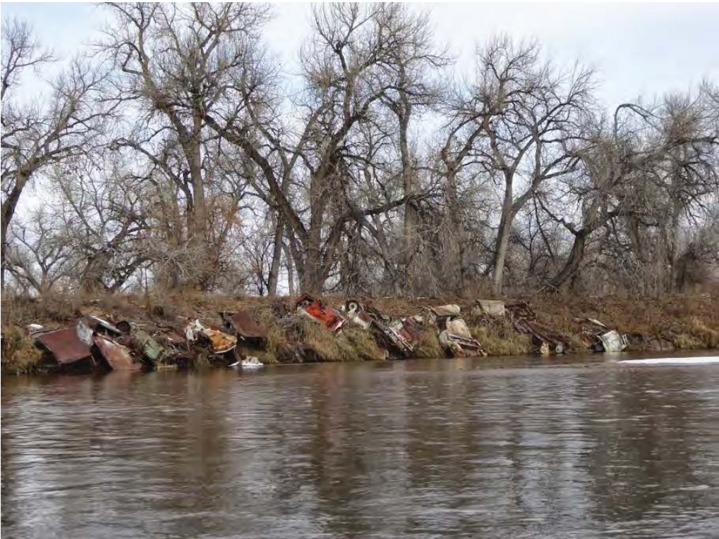
Figure 4-2. Bank Protection with Car Bodies
