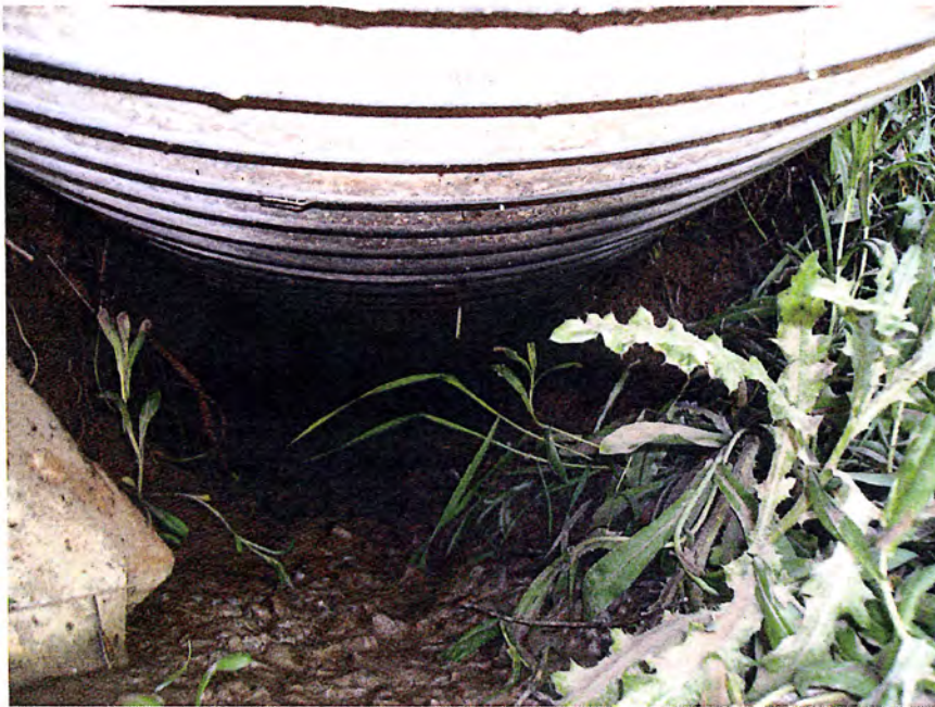
PHOTOGRAPH 3 EROSION UNDER SPILLWAY OUTLET
