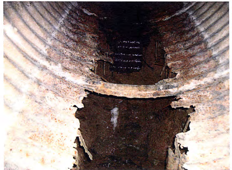
PHOTOGRAPH 2 HOLE IN SPILLWAY OUTLET
