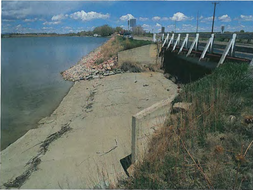
1. Looking at the upstream of the 11C County bridge and spillway for Horseshoe Lake.
