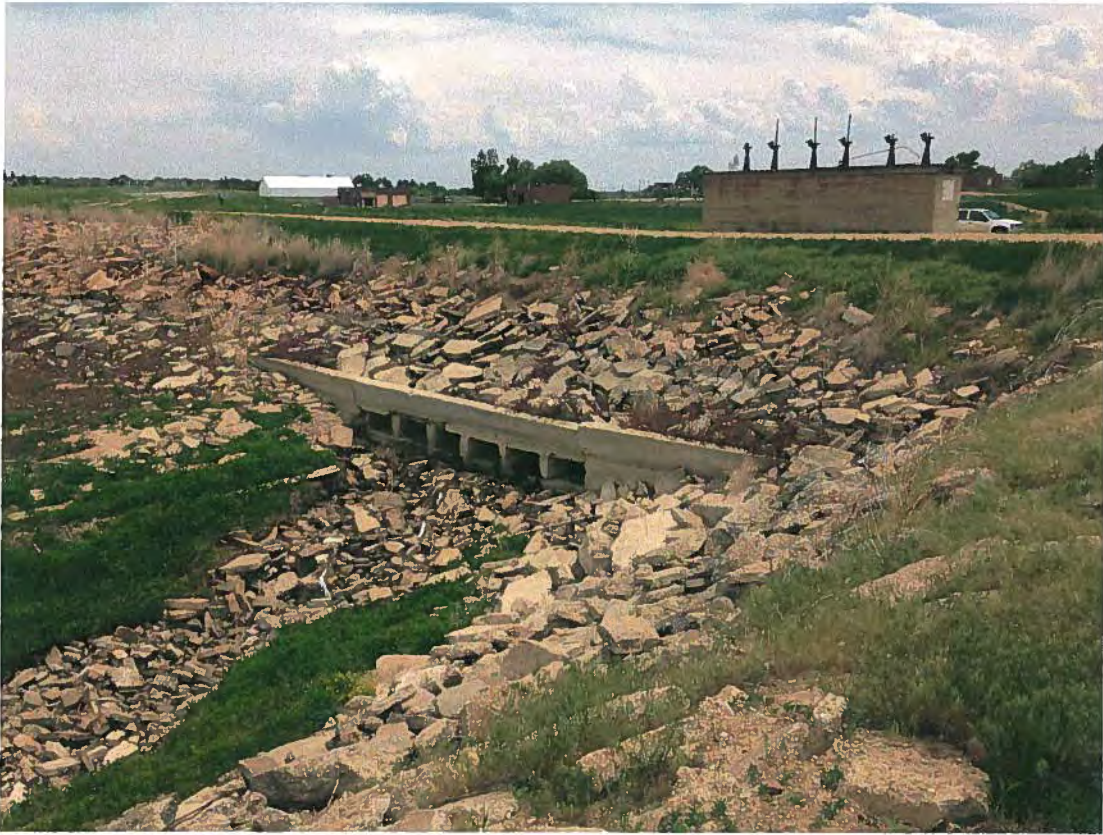
1. Looking at the upstream face of the diversion.
