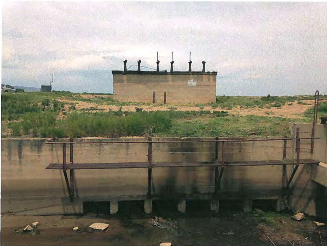
2. Looking at the can side or downstream face of the diversion.
