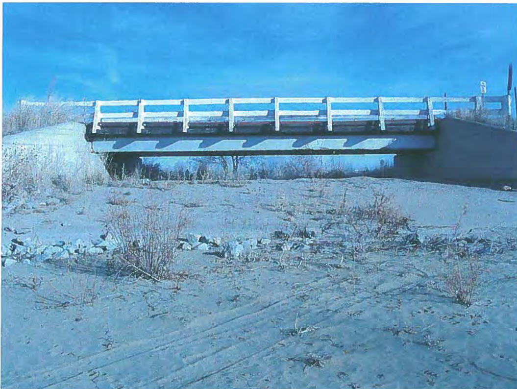
2. Looking at the upstream of the 11C County bridge and spillway for Horseshoe Lake.
