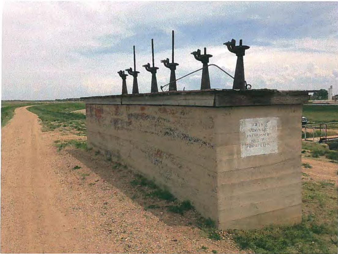
3. Existing gate structure located within the center of the dam.
