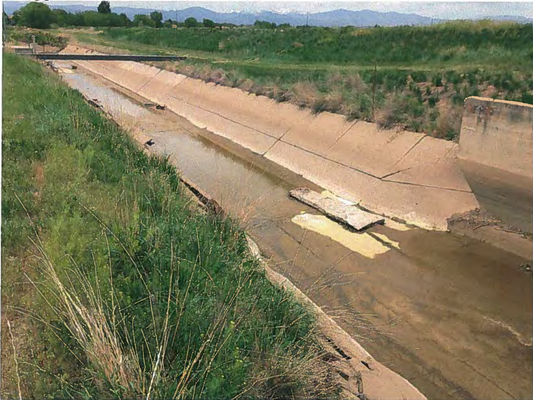
4. Upstream canal section of the diversion.
