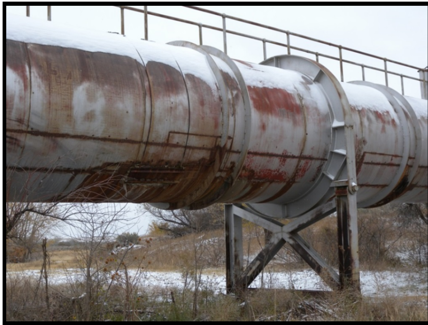
Photo No. 2 – Typical condition, leakage, and ring girder support
