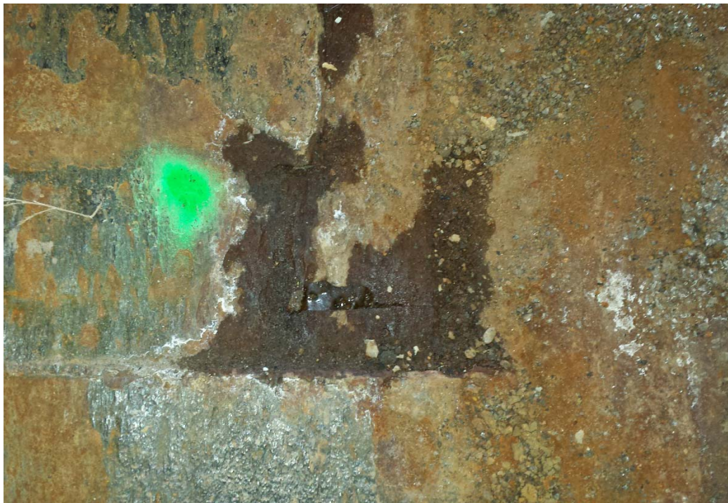
Photo 4: Hole in Cover Plates with Water Present – 2/20/15
