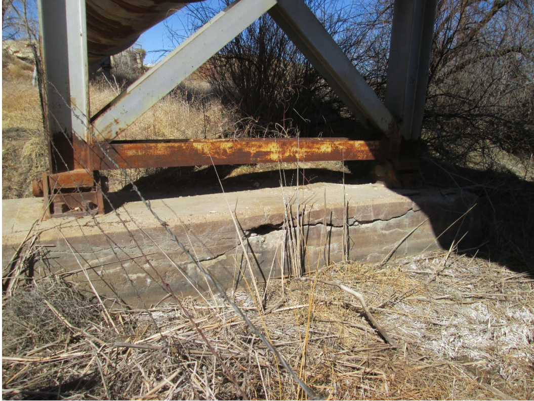
Photo 5: Cracked Foundation Supporting Ring Girder #3 – 2/20/15
