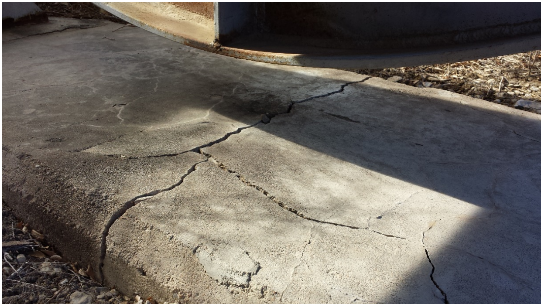
Photo 6: Foundation Broken in Half, Supporting Ring Girder #5 – 2/20/15
