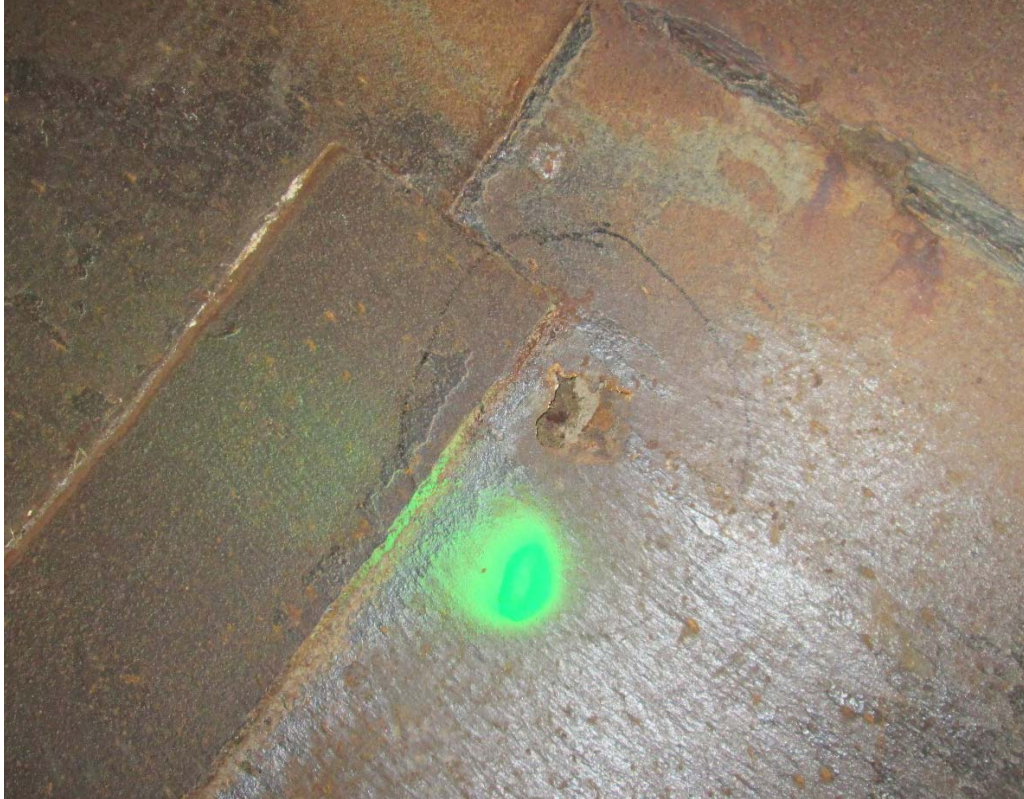
Photo 3: Hole in Cover Plate, Flume Interior – 2/20/15
