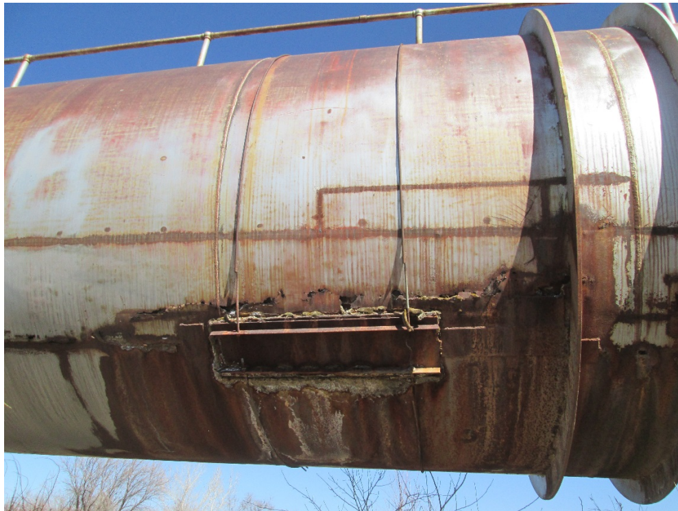
Photo 2: Flume Exterior with Patch and Significant Corrosion Along Weld Line – 2/20/15
