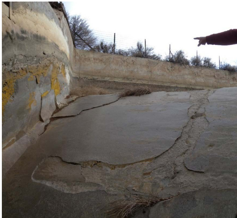
Photo 10: Heavy Abrasion on Concrete Flume Inlet – 2/20/15
