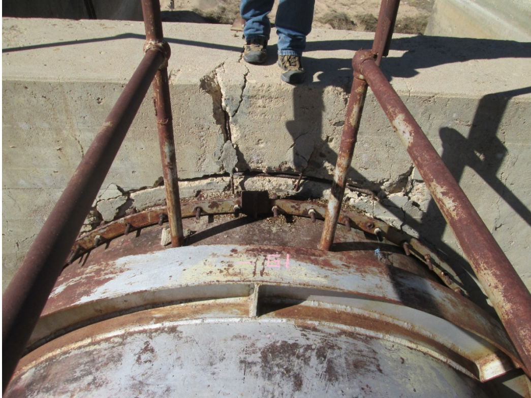
Photo 9: Expansion Joint Being Pulled from Downstream Headwall – 2/20/15
