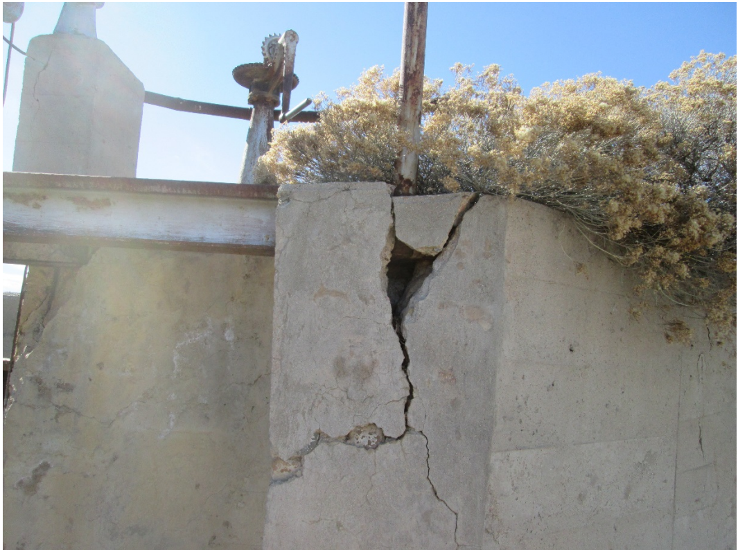
Photo 8: Damage on Outlet Structure, Below Walkway – 2/20/15
