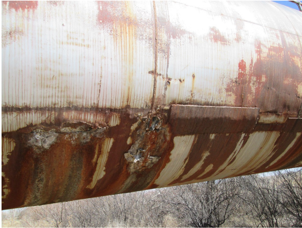
Photo 1: Corrosion and Holes on Flume Exterior – 2/20/15
