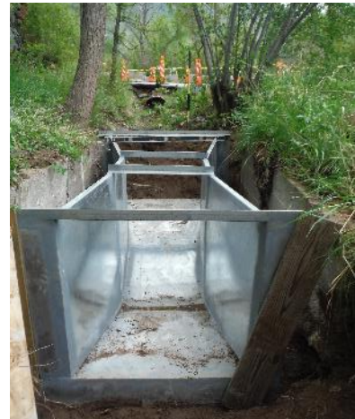
Figure 14. South Ledge diversion Parshall flume
