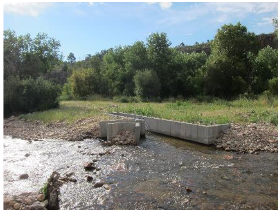
Figure 12. New intake structure and head gate on South St. Vrain Creek (river right)
