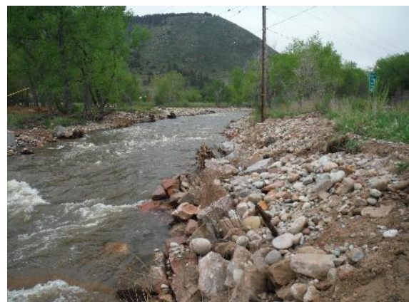
Figure 16. South St. Vrain Creek looking downstream at eroded bank on river left prior to bank stabilization and root wad installation activities.
