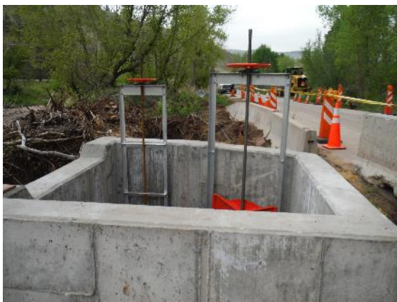
Figure 13. Splitter box that diverts water to Meadow and South Ledge ditches
