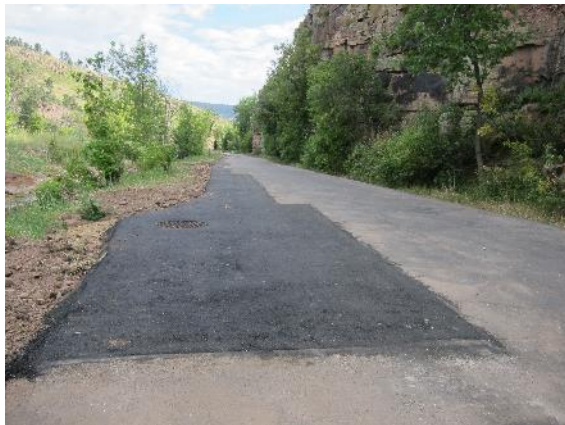
Figure 18. Road repair on Old South St. Vrain Road at manhole location.
