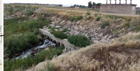
Existing Boyd Lake High-Level Outlet
