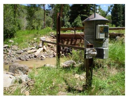
North Fork Gunnison River - New Radar Sensor Installation (Note these installations are more cost efficient as they require significantly less infrastructure than a typical stilling well and shelter)
