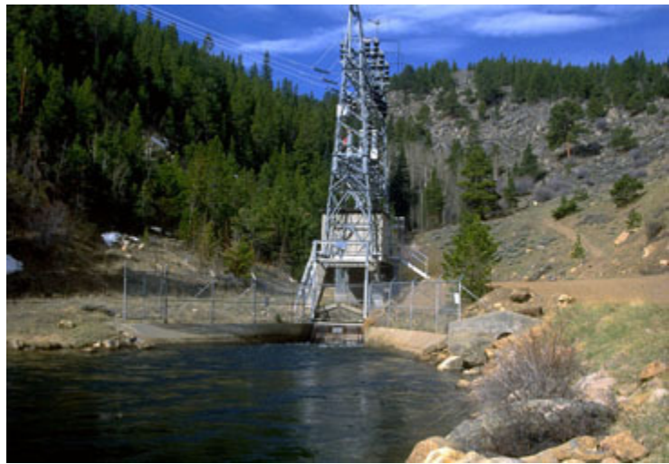
Figure 4: Adams Tunnel East Portal of the Colorado-Big Thompson Project
