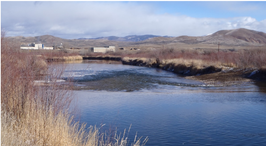
Figure 4-1 Grade Control Riffle at Riverside Ranch
