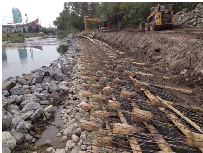
Figure 4-4 Example of Live Crib Wall Construction-Level 2 Alternative
