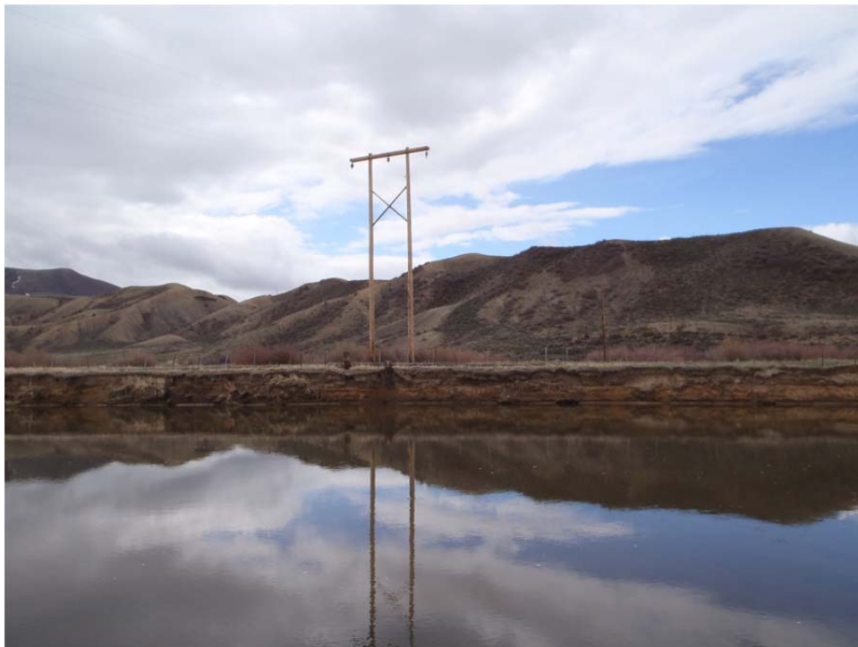
Figure 9. Severe bank erosion between McElroy No. 2 Ditch and McElroy No. 1 ditch. It's likely that the channel has experienced a headcut and now the oversteepened banks are eroding.
