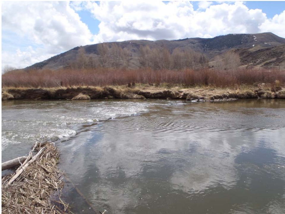
Figure 11 Bank erosion at Thompson Pump No. 1. May be caused by both headcutting and improperly constructed drop structure that focuses stresses on the bank.
