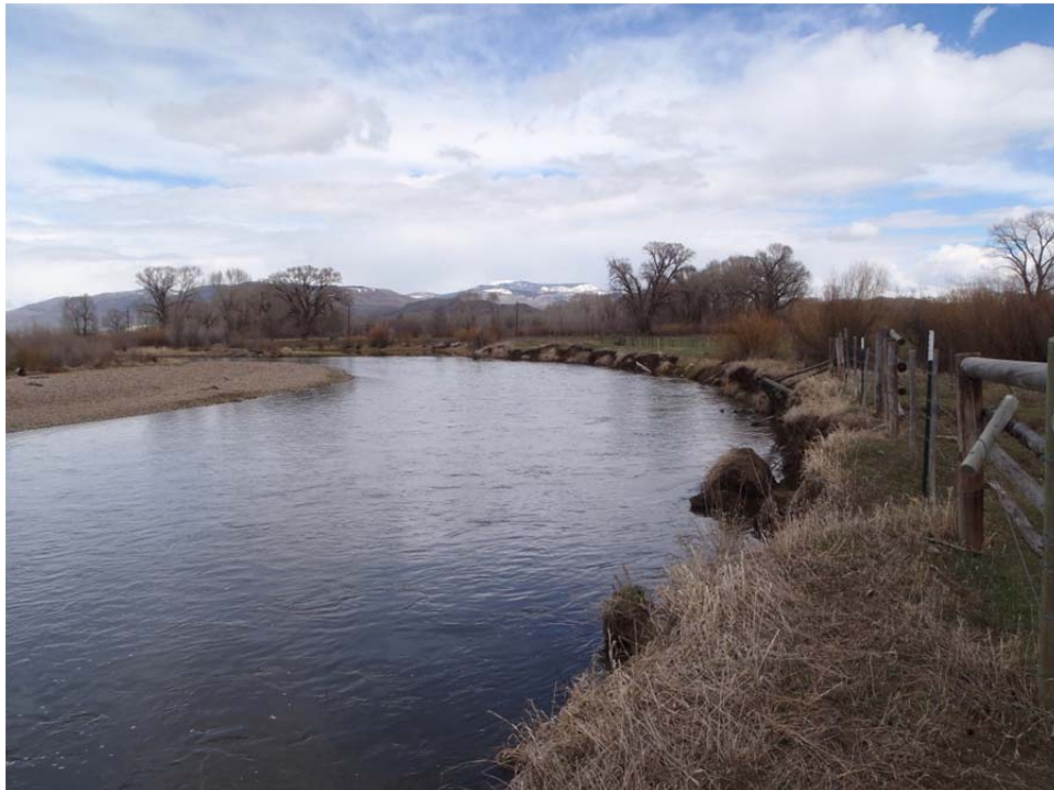
Figure 14. Bank erosion downstream from Ennis Pump Point of Diversion. This reach may be impacted by previous "restoration" activities. Improperly implemented j-hooks may have exacerbated bank erosion. Reach is noticeably narrower than downstream reaches.
