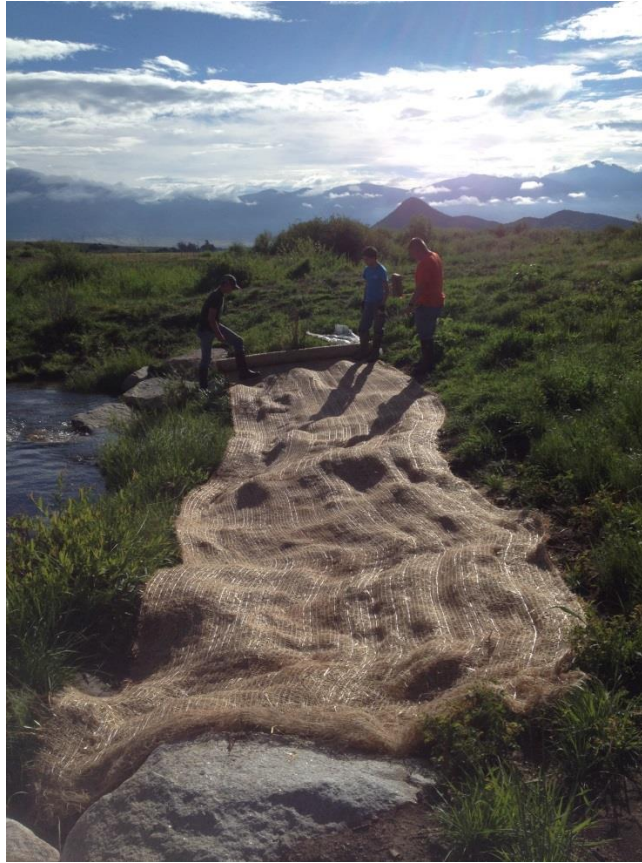
Figure 4.1: Boy Scouts installing erosion control mats on newly reshaped streambanks.
