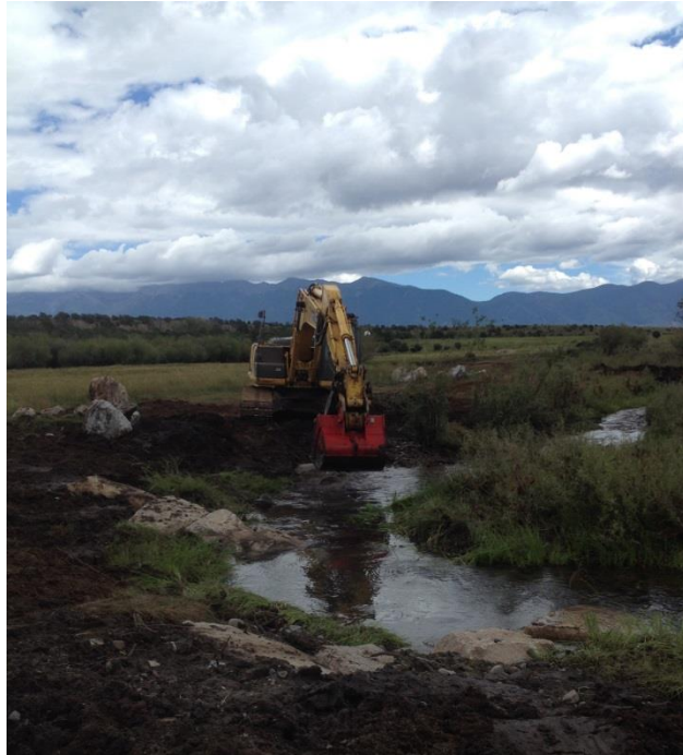
Figure 4.5: Excavator installing in-stream rock structures along Kerber Creek at KC16-E
