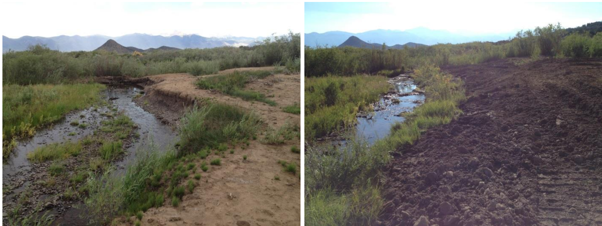
Figure 5.1: KC16-E looking east at degraded steep banks before restoration (left) and after restoration and installation of 3 rock barbs (right)
