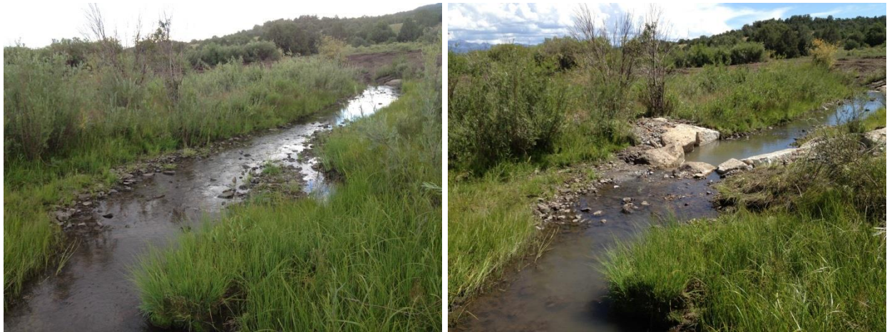
Figure 5.3: KC16-E Featureless section with extended shallow riffle zone (left) and cross vane installation creating downstream pool habitat and grade control before 90 degree bend (right)
