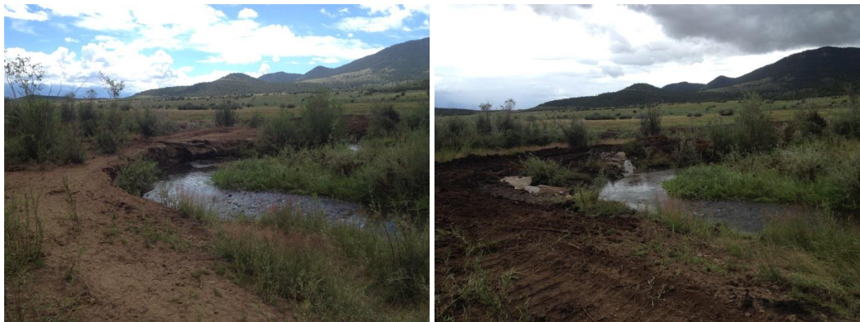
Figure 5.2: KC16-E meander bend before restoration (left) and after installation of two rock barbs and sedge/willow transplants (right)
