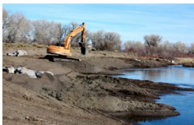
Rock Barb Installation and Topsoiling.
