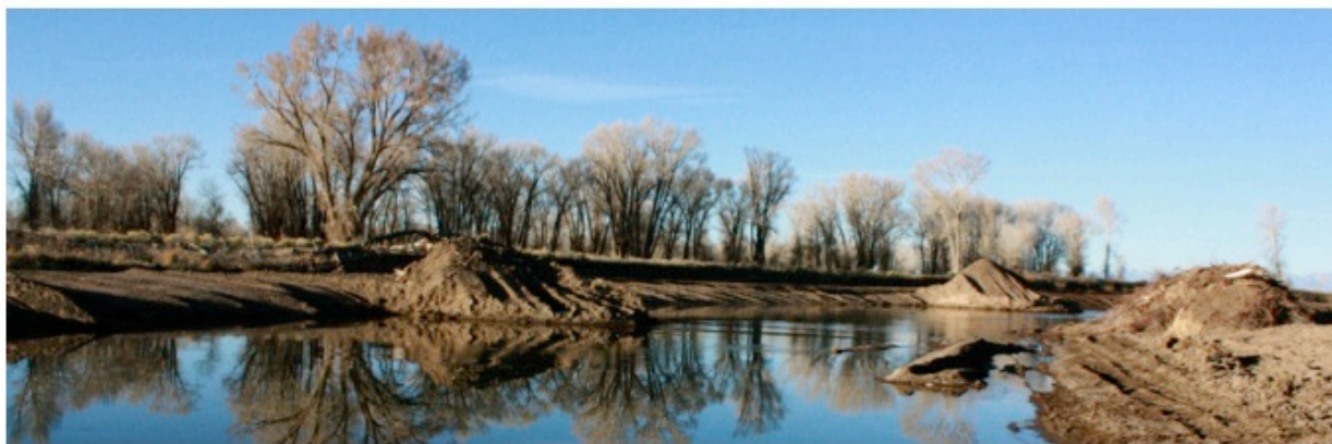
Shaping Streambanks and Piling Topsoil to Spread on Finished Benches and Streambanks.
