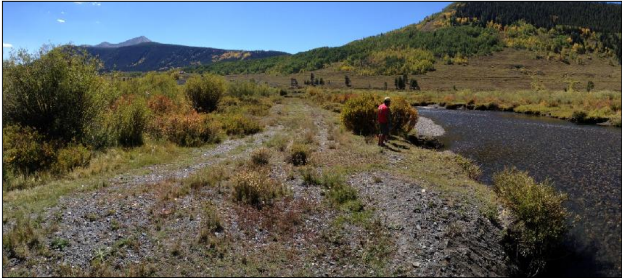
Figure A2-1: The berm is constructed mostly of compacted gravel and is about 1.5-2.5 higher than surrounding floodplain area, making it difficult or impossible for riparian vegetation to establish. As a result, the vegetation on the berm is sparse and mostly xeric. Vegetation to the right of the berm and on the other side of the river is more typical of a healthy riparian area.
