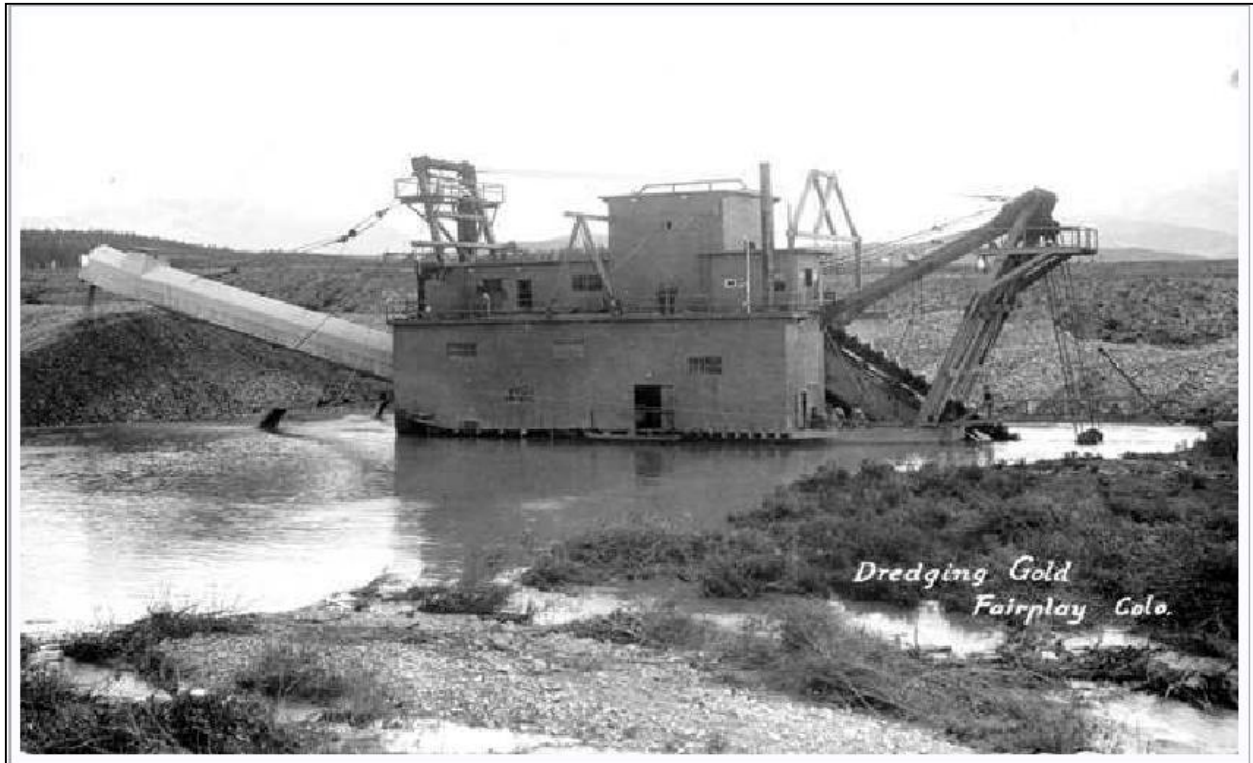
Figure 2: The dredge that operated near Fairplay until the early 1950s was a huge machine. The ones used on Tarryall were probably slightly smaller versions. Dredging in riparian areas required the removal of all soil and inundation of the area behind large dams so that the dredge boats could float along, excavating, working, and then re-depositing deep alluvial material.
