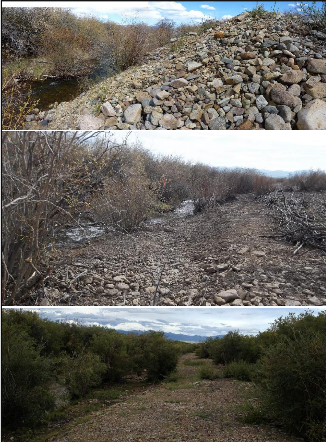
Figure 11: This time series shows the dramatic change in streamside condition. Large tailings piles were removed from the stream edge to construct a riparian bench. The root systems of existing willows were undisturbed. These plants survived and are beginning to spread.
