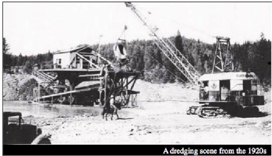
Figure 1: Dredge mining was popular in the 1920s. It was an extremely intensive process where entire streams and riparian areas were often excavated and worked.
