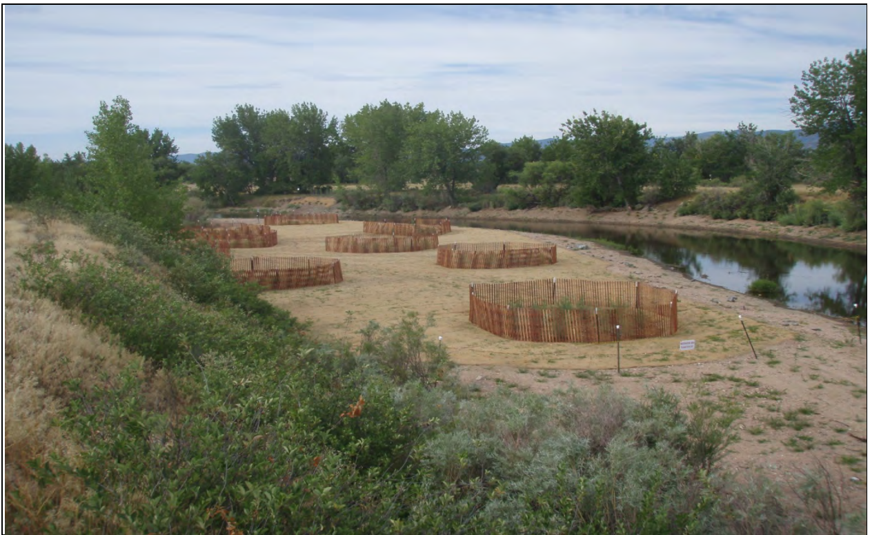
Top: Stage I of constructed point bar revegetation: point bar constructed and top soiled (Apr 2013).
