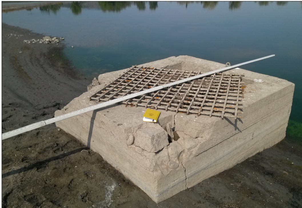
EXISTING CONCRETE INTAKE STRUCTURE WITH CRACKS AND IS IN UNSUITABLE CONDITION
