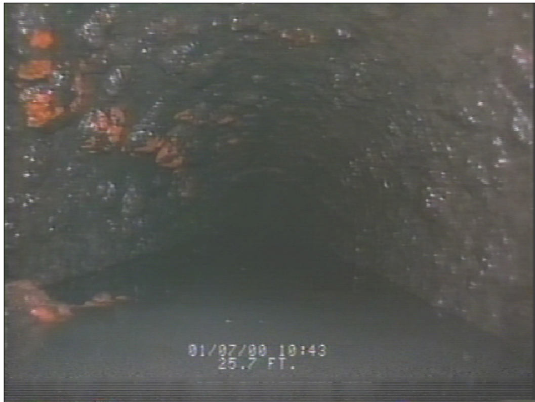
EXISTING CAST IRON PIPE THROUGH DAM EMBANKMENT THAT IS VERY CORRODED AND IN UNSUITABLE CONDITION DURING 2000 SEO DAM INSPECTION
