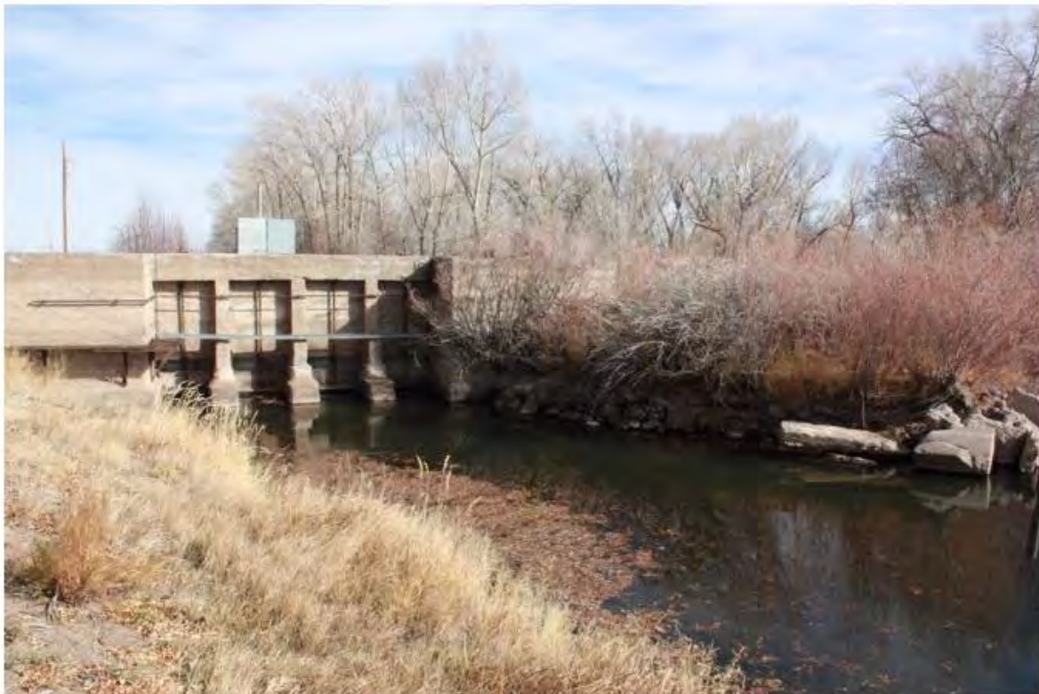
Figure 7. Prairie Ditch Headgate
