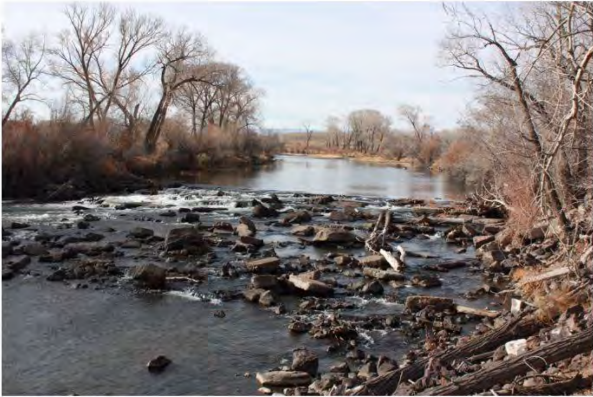
Figure 6. Prairie Ditch Diversion (Looking Upstream)
