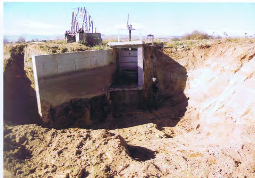
Work on Cheyenne Diversion
