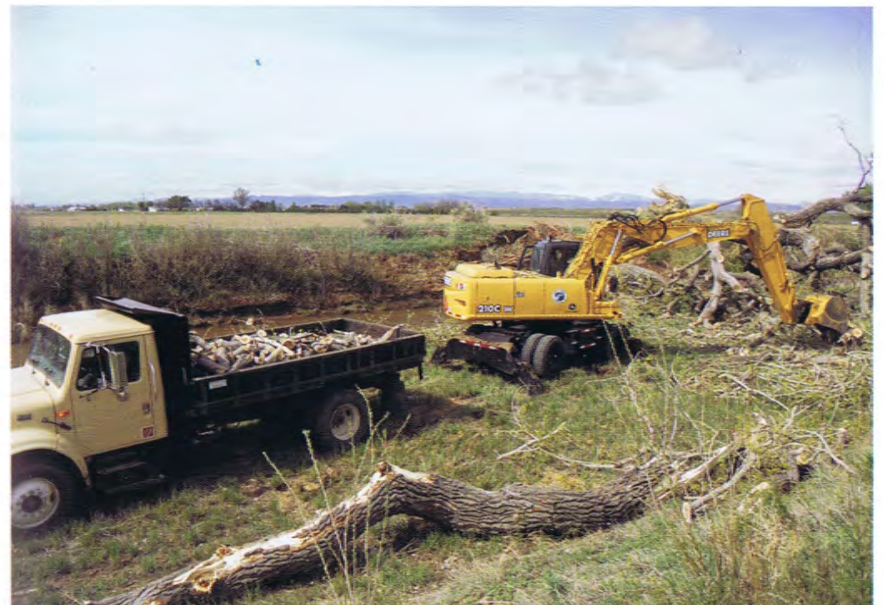
NPIC crew removing downed tree from Main Canal
