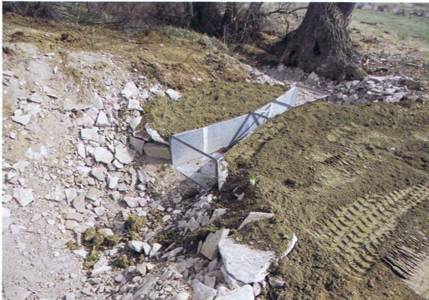
Installation of Measuring Flume on the Upper 10 Ditch completed
