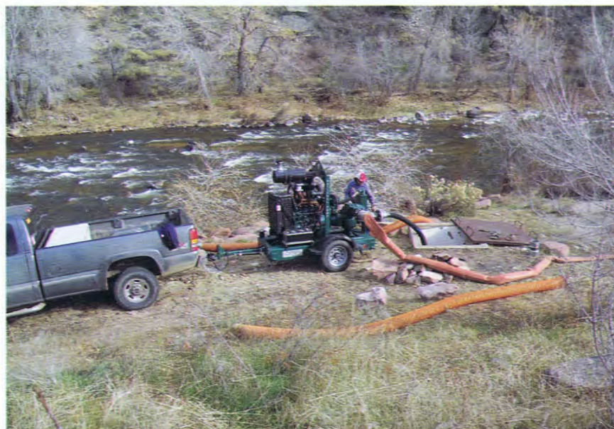
Pumping out Poudre River siphon
