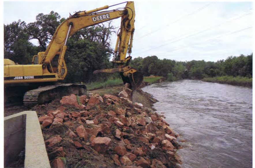
Emergency placement of rip rap above the Fossil Creek Inlet Ditch in order to prevent washout of the structure
