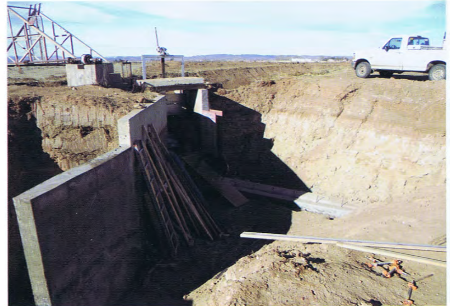
Cheyenne Diversion maintenance work on head walls
