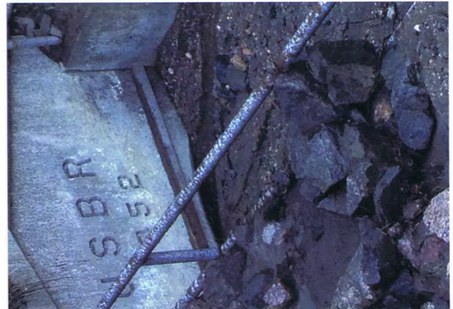
Munroe Canal diversion. June 29, 2013
