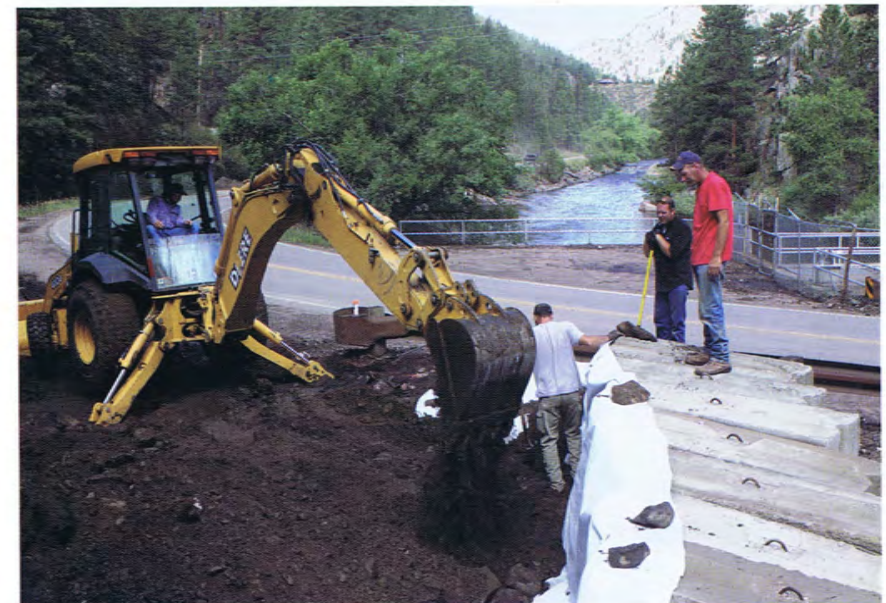
NPIC crew working at Munroe Canal Diversion
