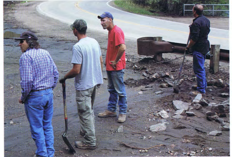
NPIC crew at Munroe Canal diversion
