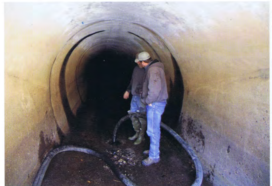
Draining Tunnel #1 above siphon
