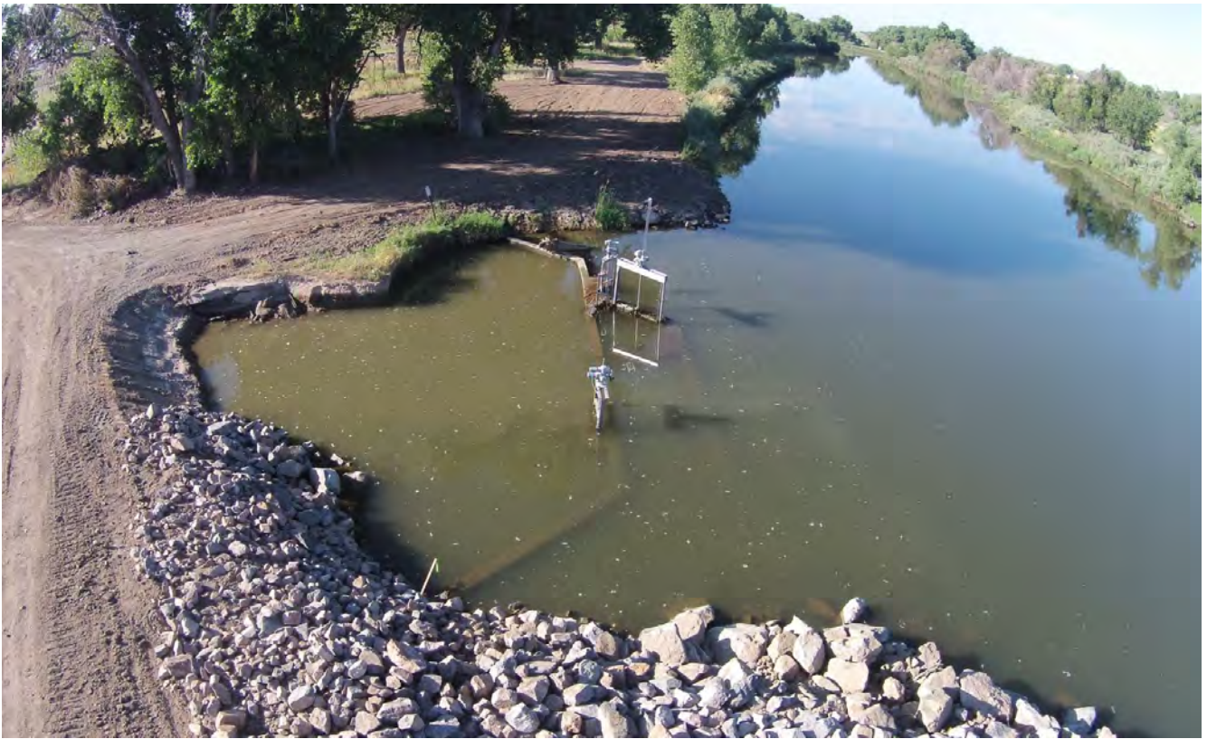
Photo 14: Post-construction aerial taken from over the cofferdam, looking upstream on the South Platte River (south) and showing the dam around the COB headgate. Photo taken July 29, 2015 (by City of Westminster). High flows have returned to the River and the BDC is diverting.
