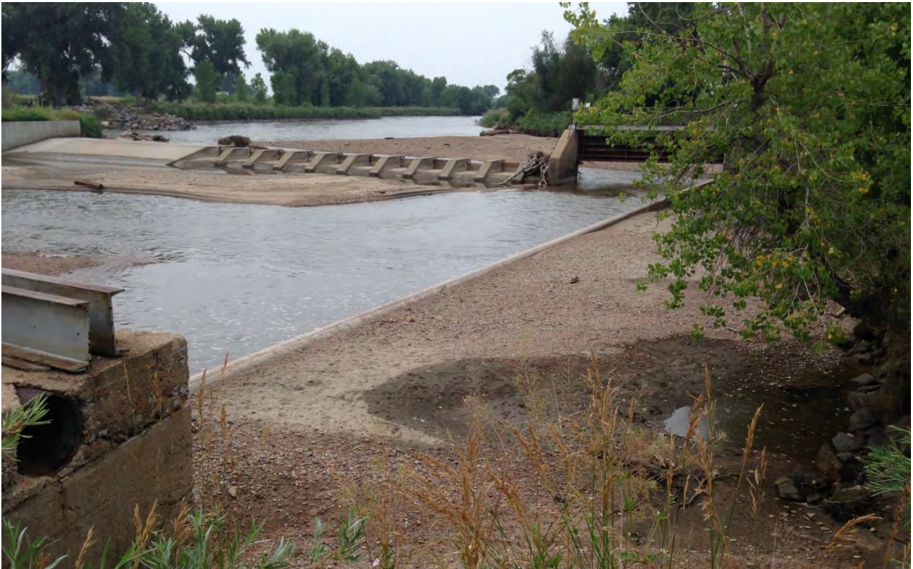
Photo 4: Taken from the BDC headgate on the downstream side of the diversion channel (which is filled with sediment) looking to the south east. Photo taken on July 7, 2015 (by Dawn Jewell) after high flows subsided. No water flowing at the BDC headgate. Majority of South Platte River flows are going through the breach which is visible in the upper left corner and minimal flows are passing through river gate visible on right side of photo. Alternative No. 2 materials are visible in background.
