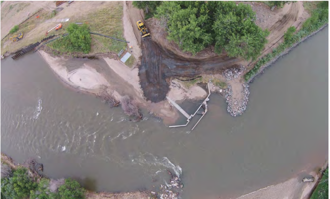
Photo 5: Aerial taken during construction showing the breach, the Alternative No. 2 materials and the beginnings of the repairs with the Zone 2 material over the COB 48" RCP line behind the COB headgate. Photo taken July 13, 2015 (by City of Westminster). COA installation of sheetpiling to protect their Prairie Water Pipeline visible in the upper left of photo.
