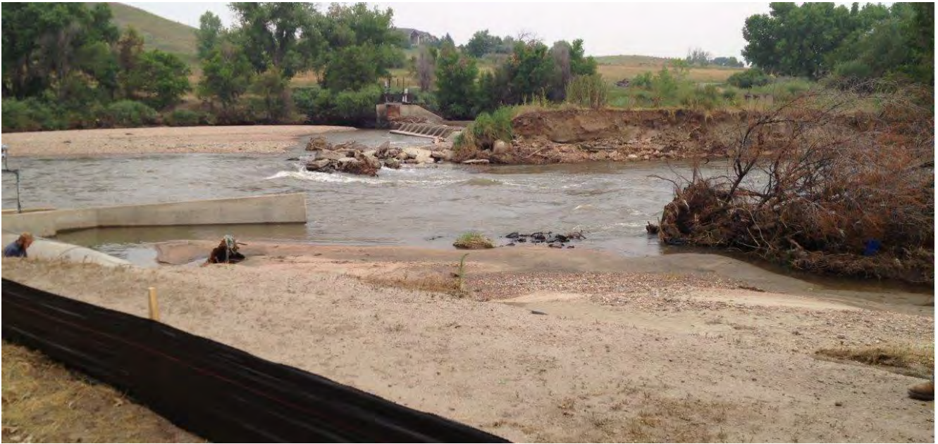
Photo 3: Taken from the east bank looking slightly northwest across breach at the BDC diversion structure in the background. Photo taken July 7, 2015 (by Colby Hayden) after high flows subsided. No water flowing at the BDC headgate. Majority of South Platte River flows are going through the breach with minimal flows passing through the river gate on the diversion dam. Structure in foreground is the COB headgate and 48" RCP line.
