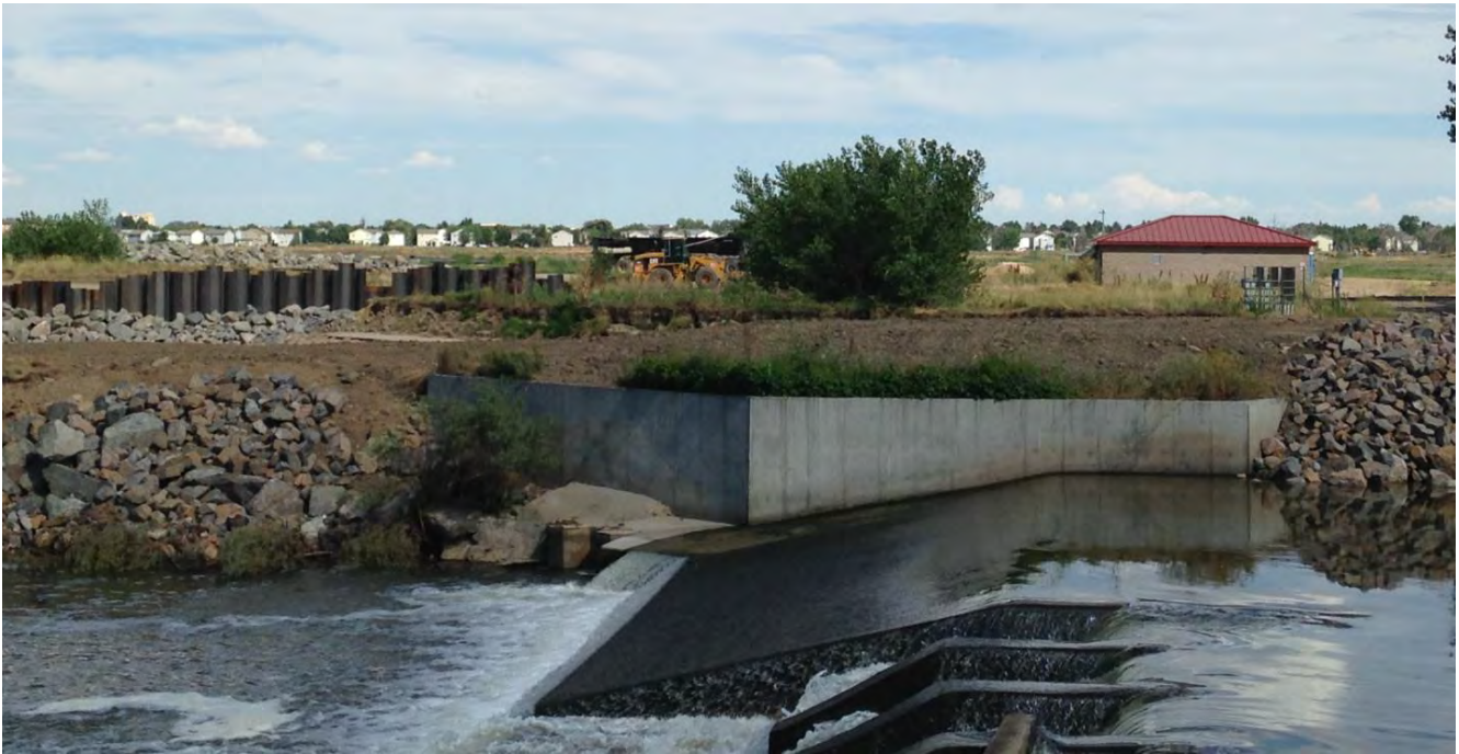
Photo 12: Photo taken from BDC diversion showing the finished cofferdam on the right, pothole repairs on the left (all part of the Alternative No. 4 design), and COA sheet piling and riprap in the back ground. Photo taken July 27, 2015 by Dawn Jewell.
