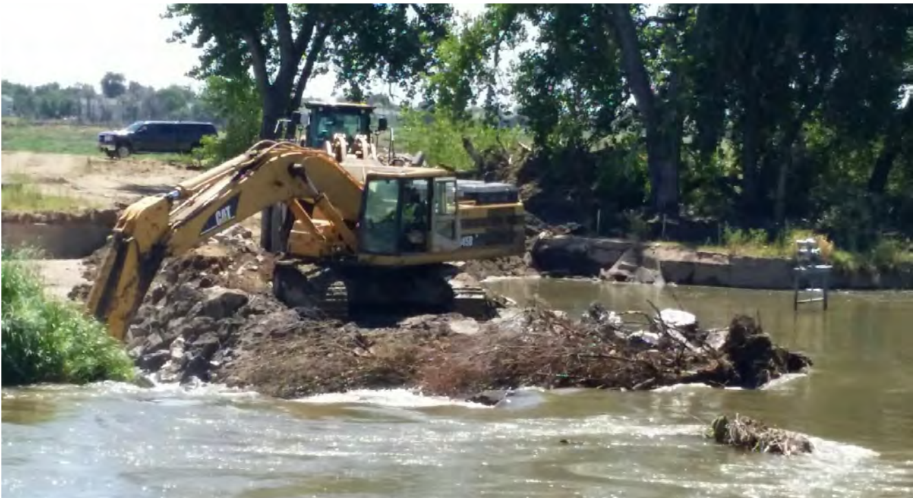
Photo 7: Photo taken from BDC diversion structure showing Alternative No. 4 repairs in progress. Photo taken July 15, 2015 (by Tom Chikuma). The COB headgate is visible but submerged on the right side of the photo. The east wing wall "island" is visible on the left as green vegetation near the end of the coffer dam.
