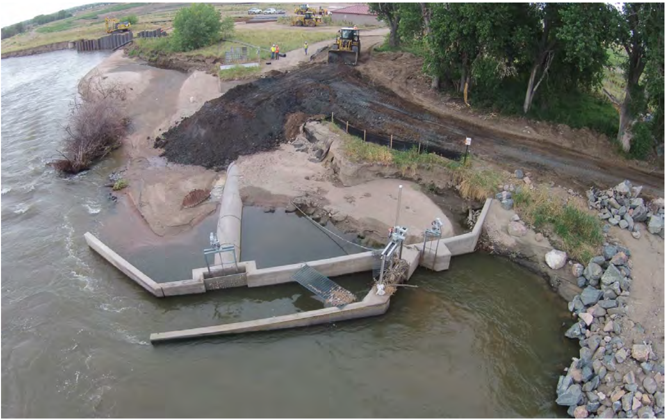
Photo 6: Aerial taken during construction showing the breach, the Alternative No. 2 materials (on the right side of the photo) and the beginnings of the repairs with the Zone 2 material over the COB 48" RCP line behind the COB headgate. Photo taken July 13, 2015 (by City of Westminster). COA installation of sheetpiling to protect their Prairie Water Pipeline visible in the upper left of photo.
