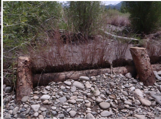
Sediment upstream, gravel downstream & no growth
