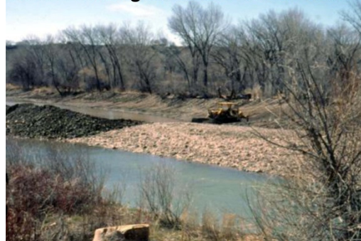
Gravel mining at River Park in 1997
