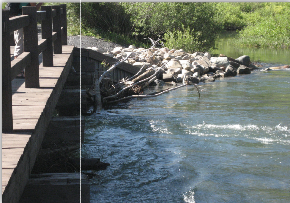
Figure 9: Debris Jams are Common at the Gunsight Bridge
