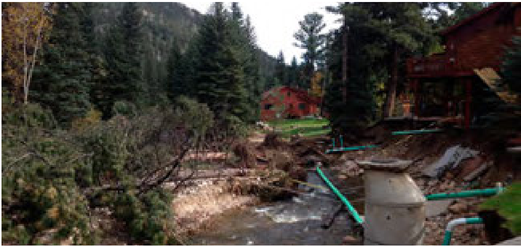
Antlers Point Utility Damage
