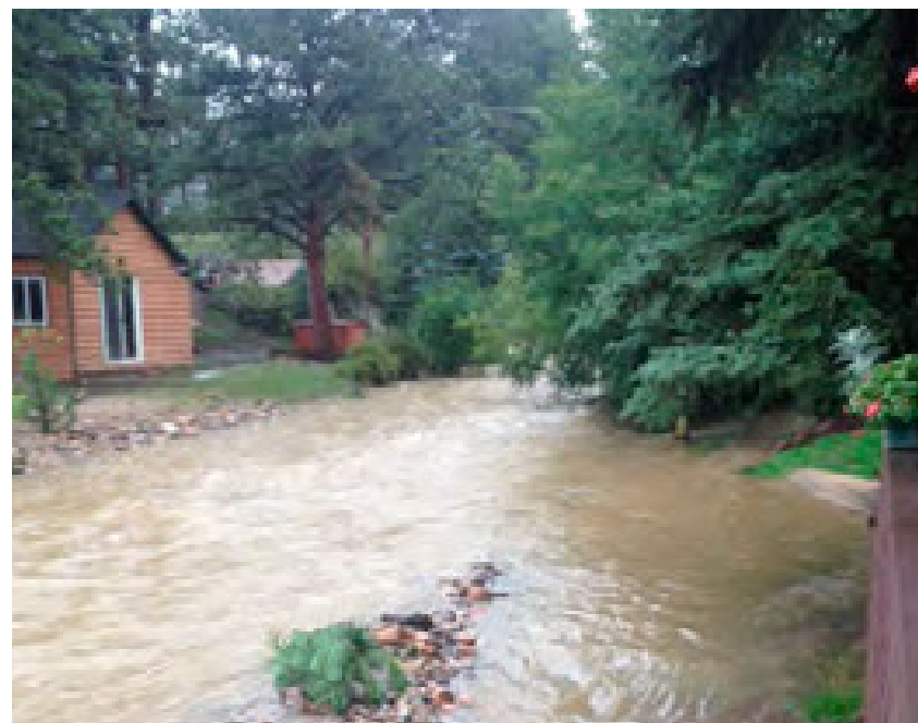
Fall River Post Flood Damage
