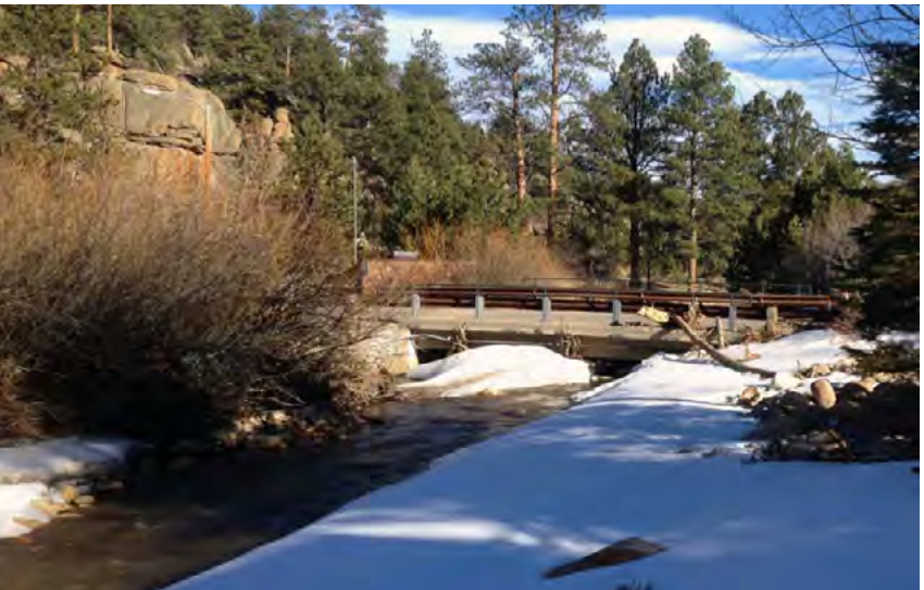
Town Bridge at Fall River Court
