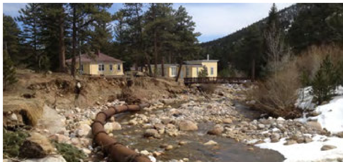
Post Flood Image Looking Downstream
