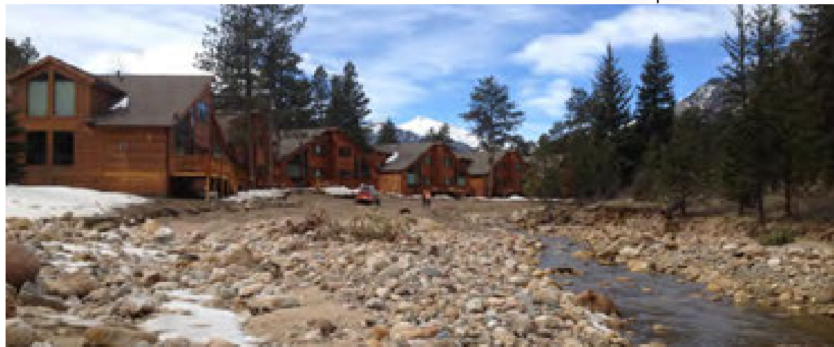
Post Flood Image Looking Downstream
