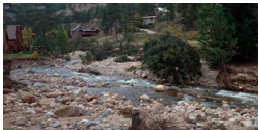
Fall River Post Flood Damage
