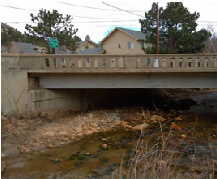
Existing Bridge on Fall River
