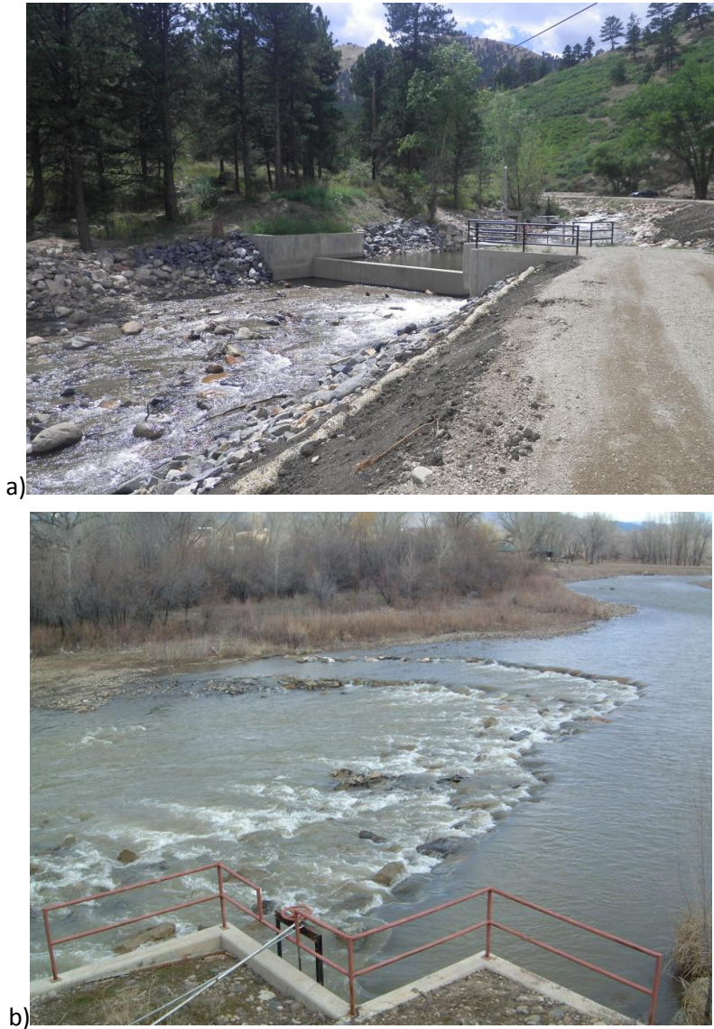
Figure 29. New Diversion Structure at Canyon Mouth
