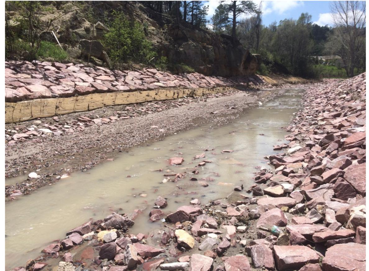
Figure 4-14. Soil Rip Rap Channel with Rip Rap Bank Stabilization at Greencrest Channel
