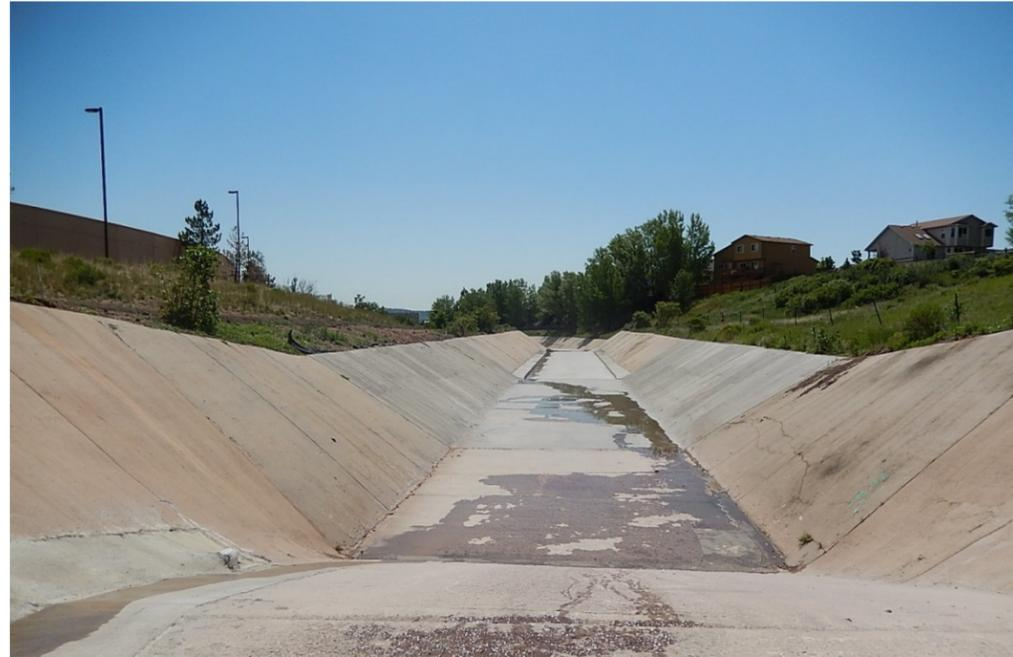
Figure 4-9. Full- Lined Concrete Trapezoidal Channel in Douglas Creek, Colorado Springs
