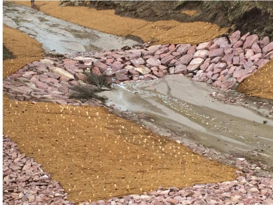
Figure 4-6. Constructed Small Drop Structure in Greencrest Channel, Colorado Springs
