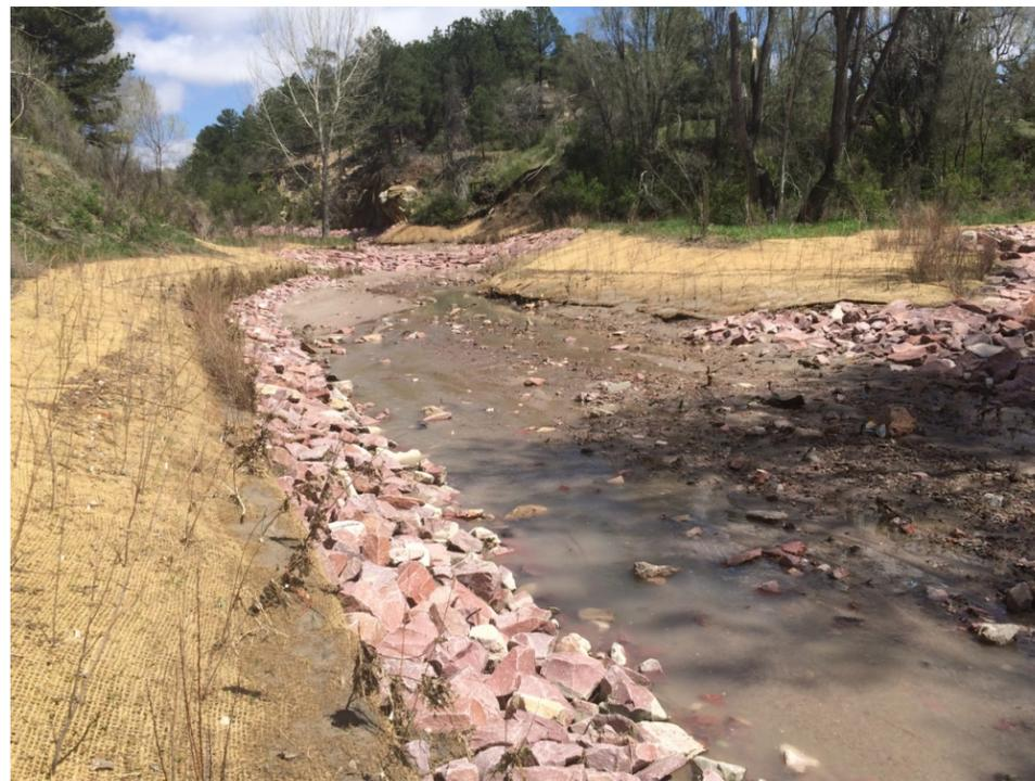
Figure 4-7. Constructed Side Slope Toe Protection in Greencrest Channel, Colorado Springs
