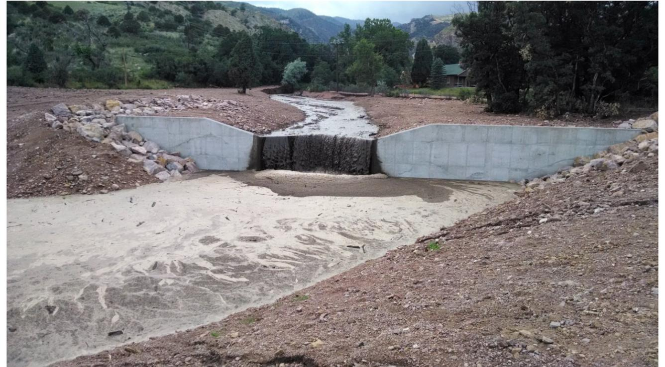
Figure 4-8. Constructed Large Drop Structure in Camp Creek, Colorado Springs
