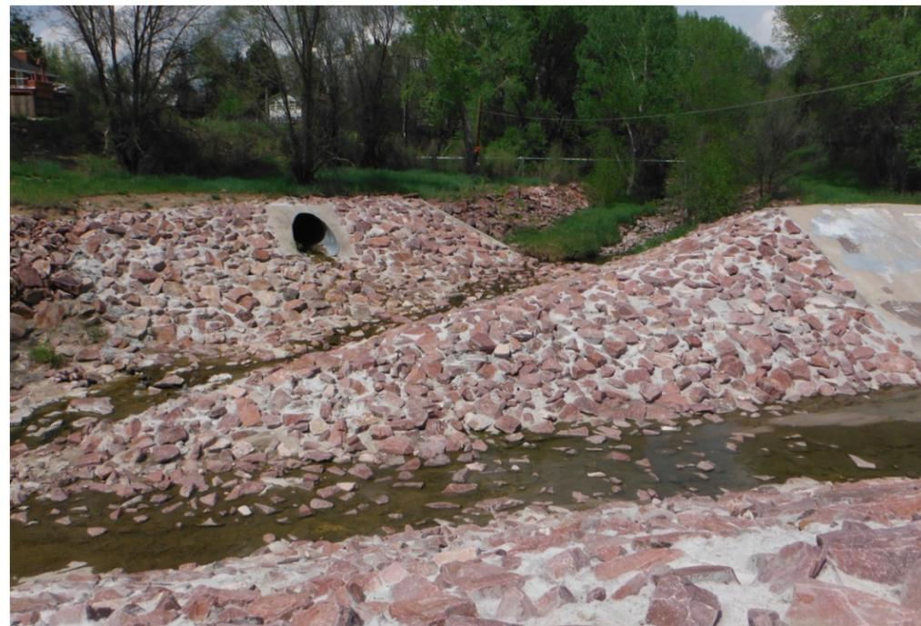
Figure 4-10. Fully-Lined Rip Rap Channel in Greencrest Channel, Colorado Springs
