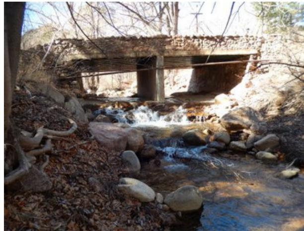
Figure 3-8. Evans Bridge Failed Grade Control
