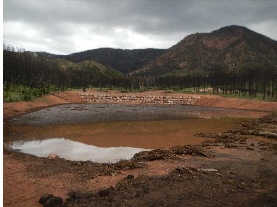
Figure 4-13. Constructed Sediment Basin at North Douglas Creek, Colorado Springs
