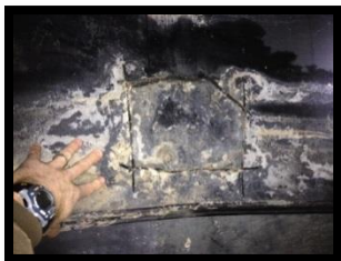
CUT HOLE IN TUNNEL PIPE
