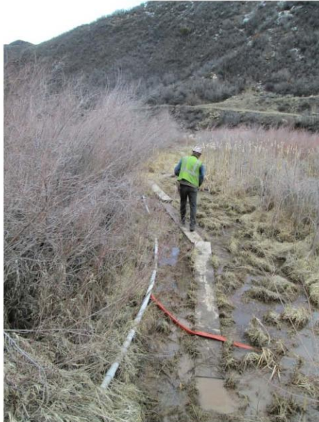
Picture of white pipe bring water from the river to the pond and the red pipe bring water directly to the pump house cistern. Picture is from the pond looking toward the river.
