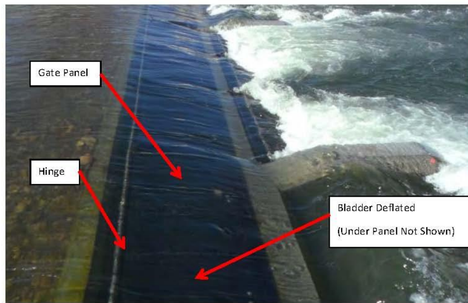
Figure 7 – Overshot Gate in “Down” Position at Thurman Mill Diversion Boise River, ID
