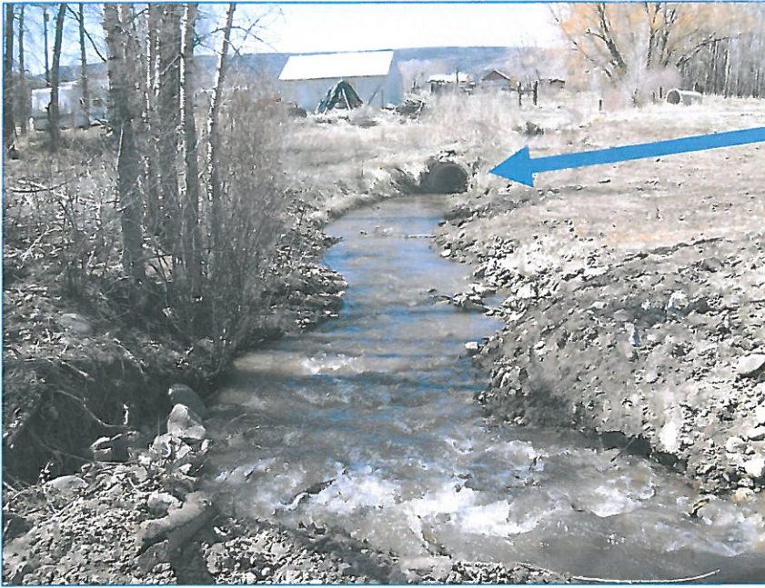
Concrete Culvert Structure before Picture— was impeding the water flow downstream from the newly built structure.
