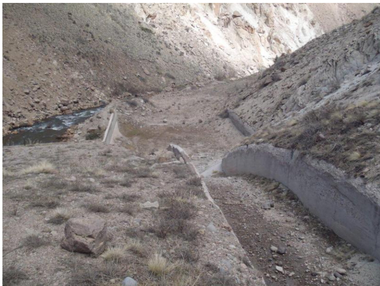
Looking down the spillway chute into the stilling basin located at the downstream dam toe.
