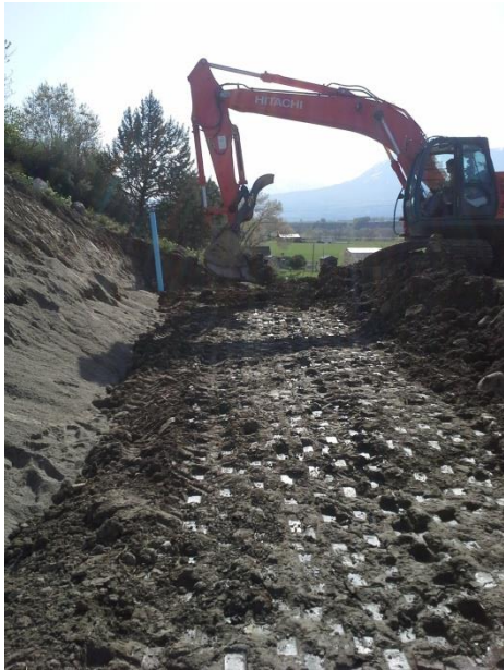
Photo 3 Drain Backfill and Compaction
