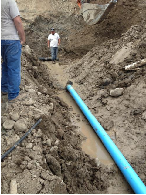
Photo 2 – Drain Install
